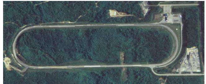
Figure 1. Top Down View of NCAT Track
