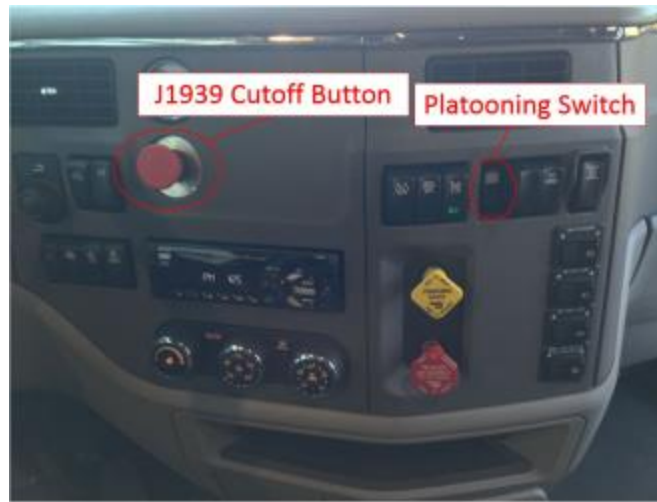
Figure 4: Installation of Platooning Switch and Cutoff Button
