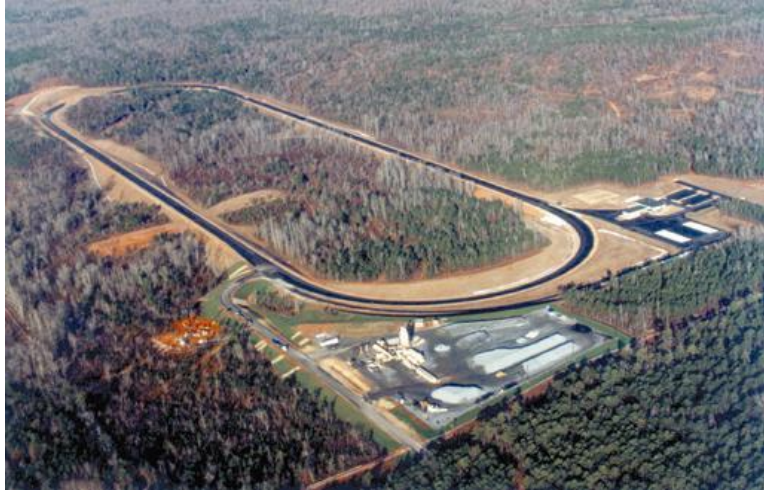
Figure 97: The test track at the National Center for Asphalt Technology.
