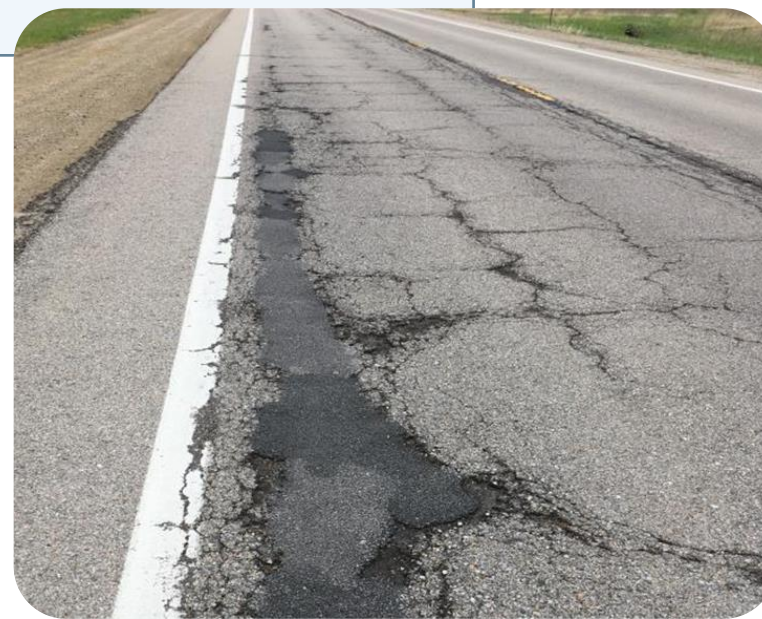
Conventional Paving - .05 gal/yd 2
