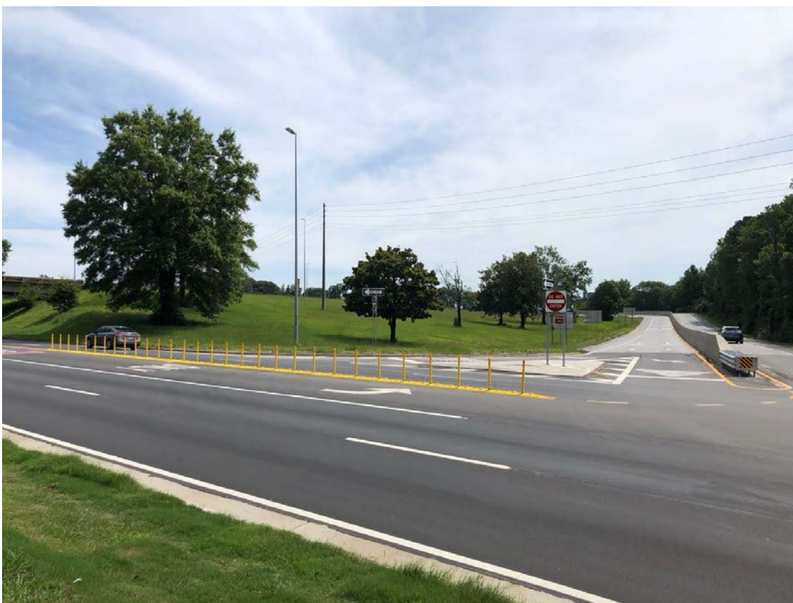
Figure 42. Quick Kurb Installed on the Crossroad near an Off-Ramp Terminal
