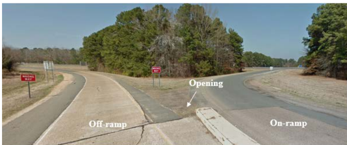
Figure 30. Example of Median Opening Before the Fork Area (I-30 Exit 63, AR) (Source: Google Maps)
