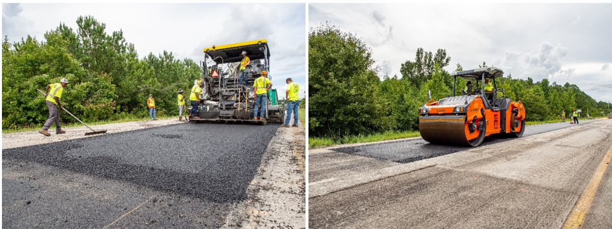
FIGURE 6 Construction of Section S7B.
