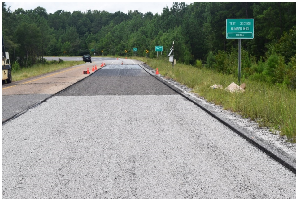
FIGURE 3 Section N12-C chip seal with No. 7 stone (foreground) and N13-A chip seal with RAP (background).
