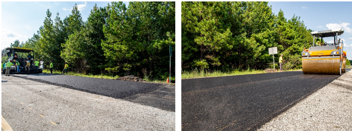
FIGURE 16 Laydown and compaction of N9 surface mix.
