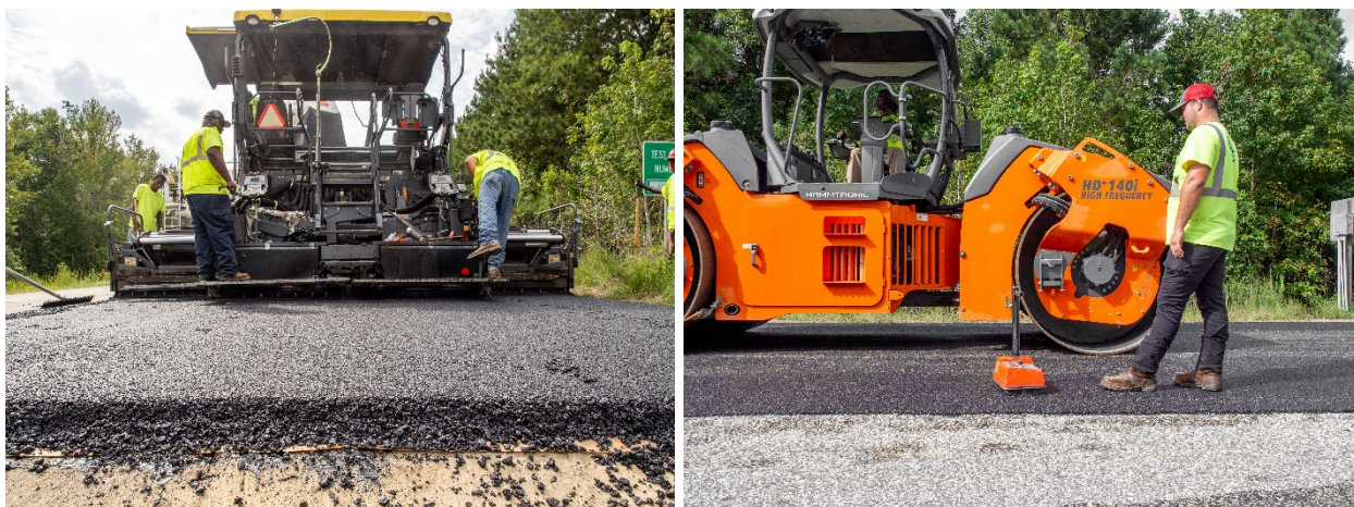
FIGURE 6. Constructing Section N6 with a BMD mix.
