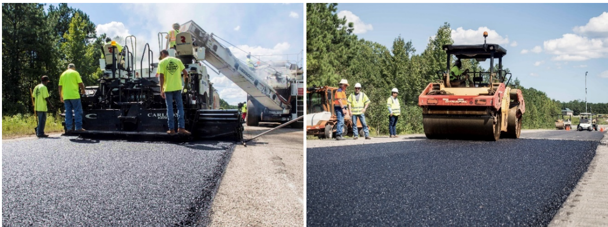
FIGURE 4. Constructing Section S10 with a BMD mix.
