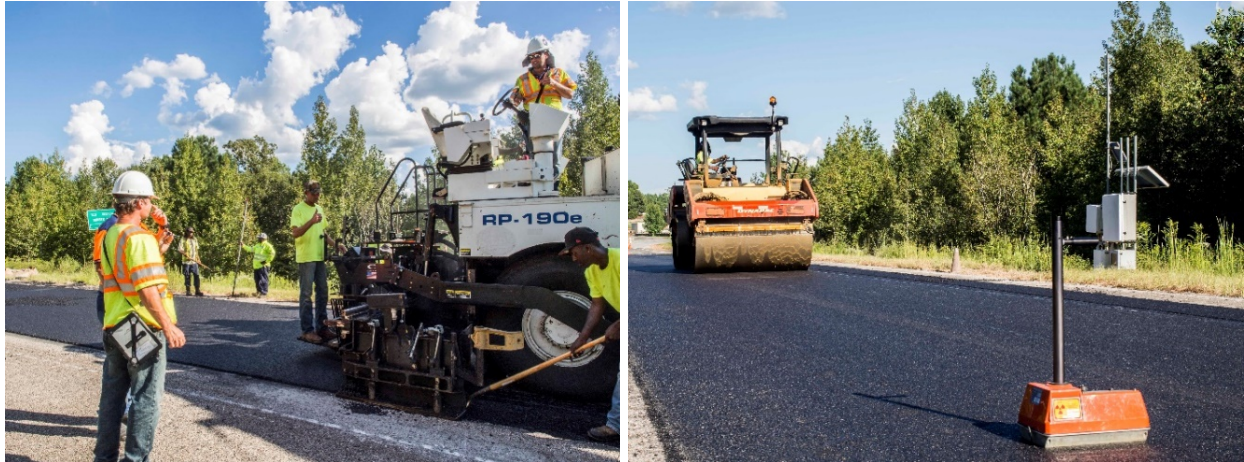
FIGURE 5. Constructing Section S11 with a volumetric mix.
