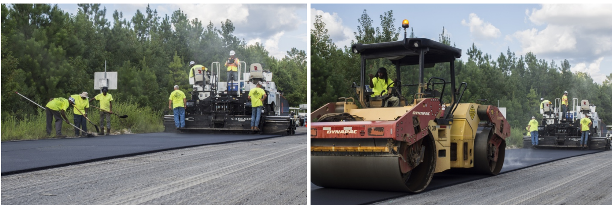
FIGURE 1 N10 mix placement and compaction.
