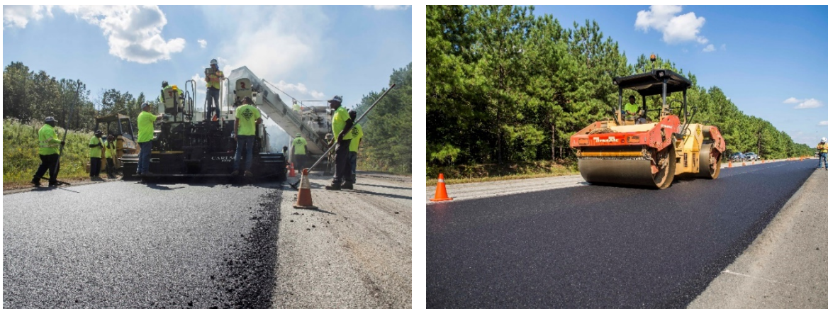
FIGURE 4 Laydown and compaction of S1 surface mix.
