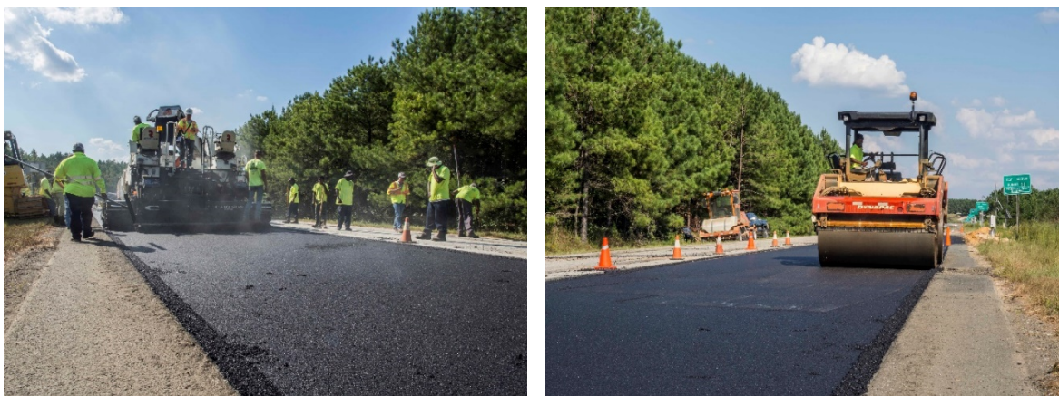
FIGURE 3 Laydown and compaction of S1 base mix.
