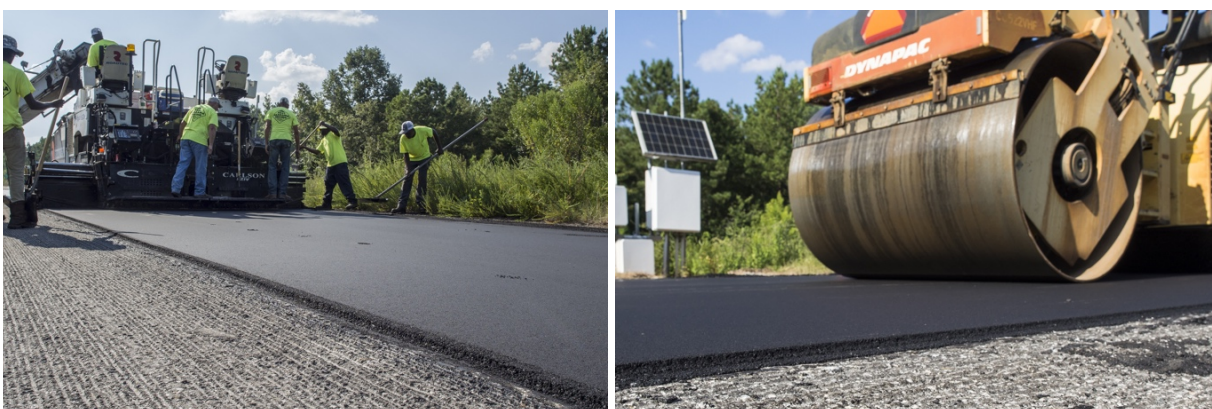
FIGURE 2 N11 mix placement and compaction.
