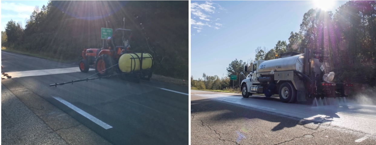
FIGURE 1 S3-A and S3-B application of spray-on rejuvenators.
