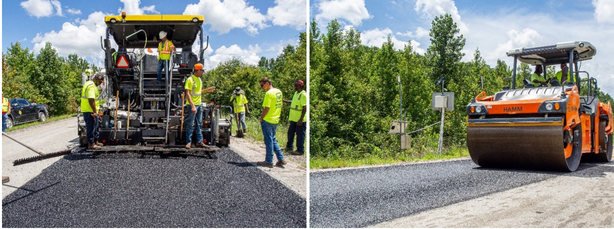
FIGURE 5 Construction of Section S7A.
