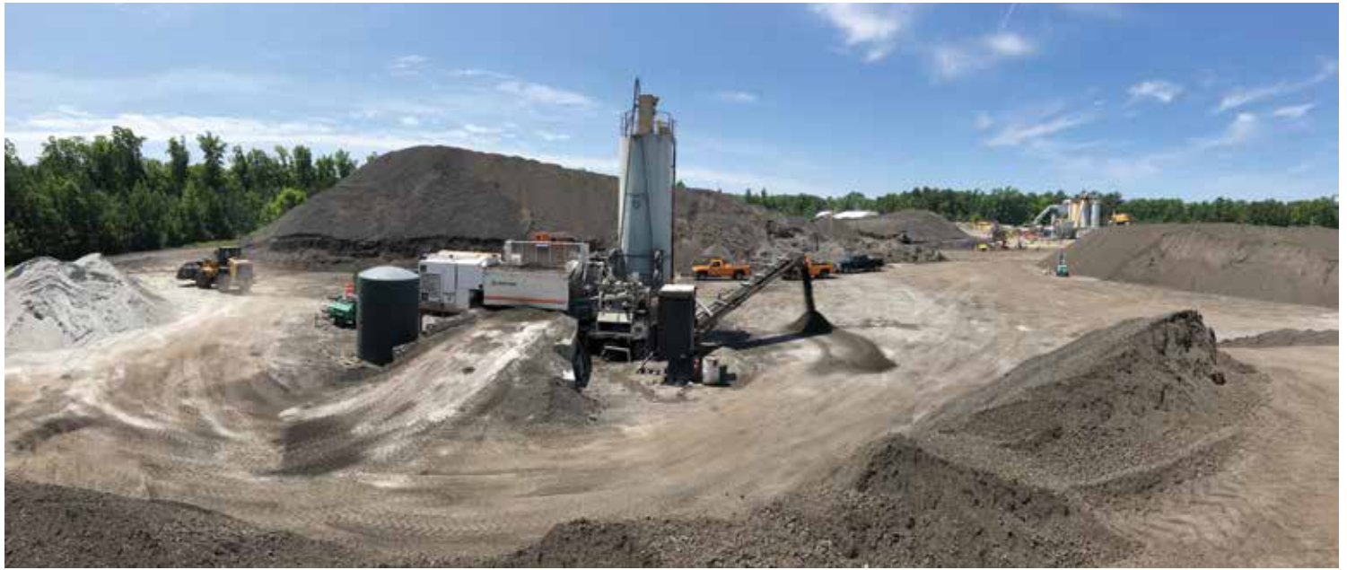
In cold central plant recycling, the asphalt recycling takes place at a central location using a stationary cold mix plant.
