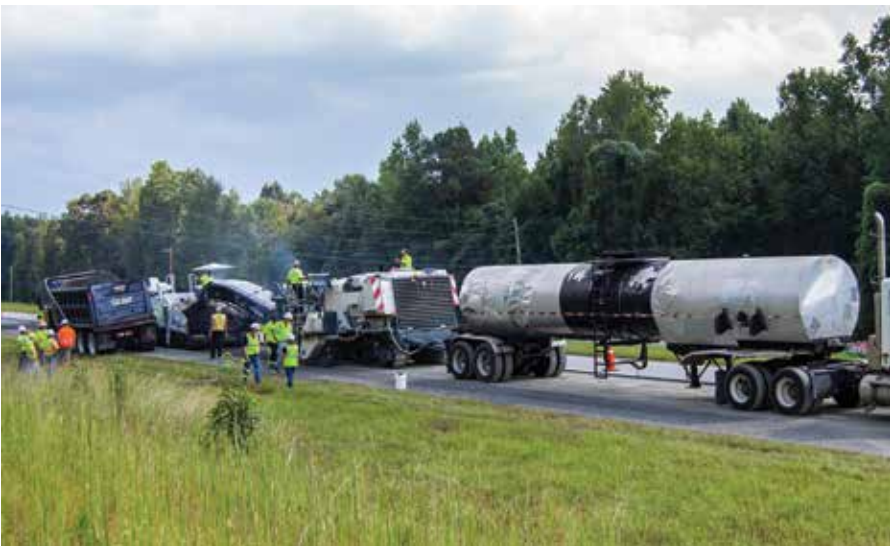
Cold in-place recycling involves the same process as cold central plant recycling except that it is performed in-place by a train of equipment.
