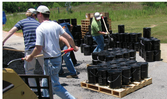
During test section construction, mix is collected prior to laboratory testing.
