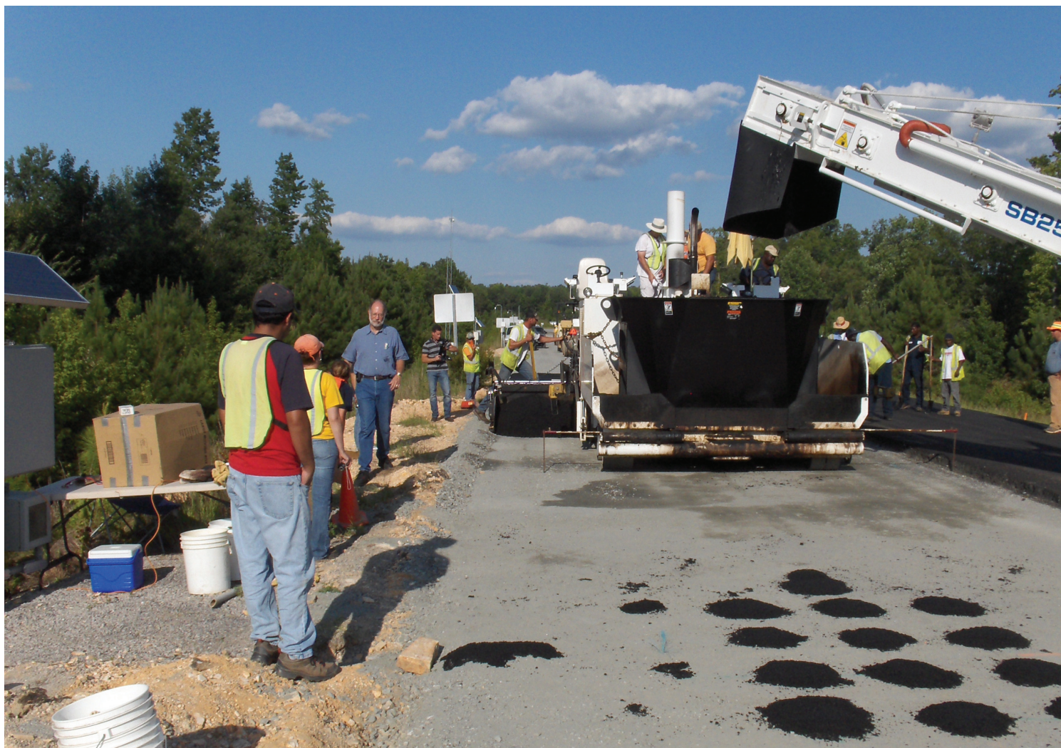
Prior to paving a structural section at the Test Track, hand-sifted mix is placed over strain gauges.
