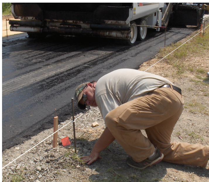
The paving crew used stringline to establish the correct elevations for leveling the inside lane at the Test Track.
