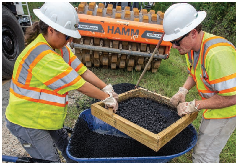
Rachel Cousins (left) works with Matthew Sasser (right) to sieve mix for embedding the instrumentation in Section S5 of the Additive Group experiment.
