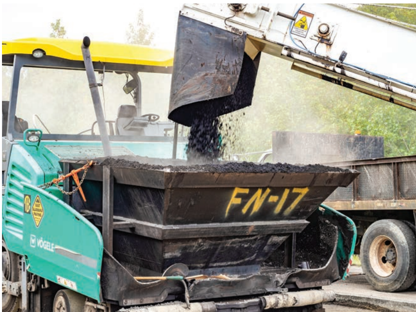
The mix for BASF's Section S13 is transferred from the truck to the paver by a shuttle buggy.
