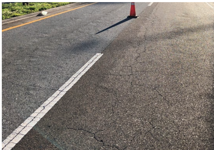
Example of road worms, photo courtesy of Greg Sholar.
