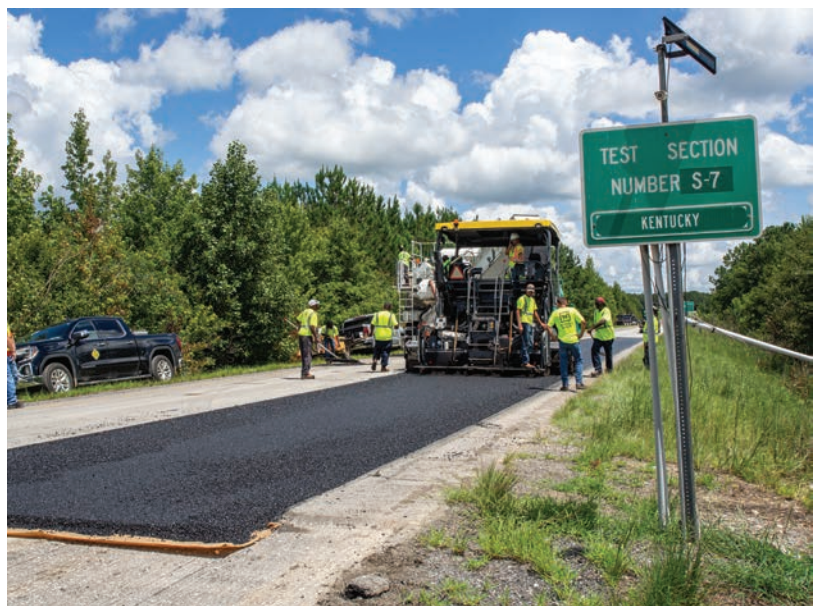
The crew paves Kentucky's balanced mix design Section S7.
