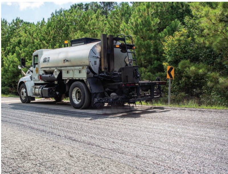
Tack coat is applied to North Carolina's Section W4 in the Test Track's west curve.
