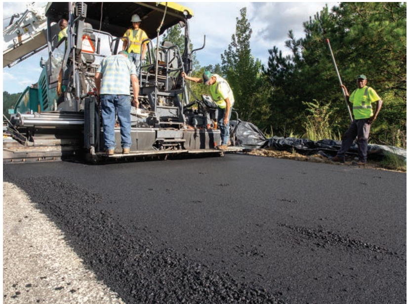
Section S6 of the Additive Group is paved on the south side of the NCAT Test Track.
