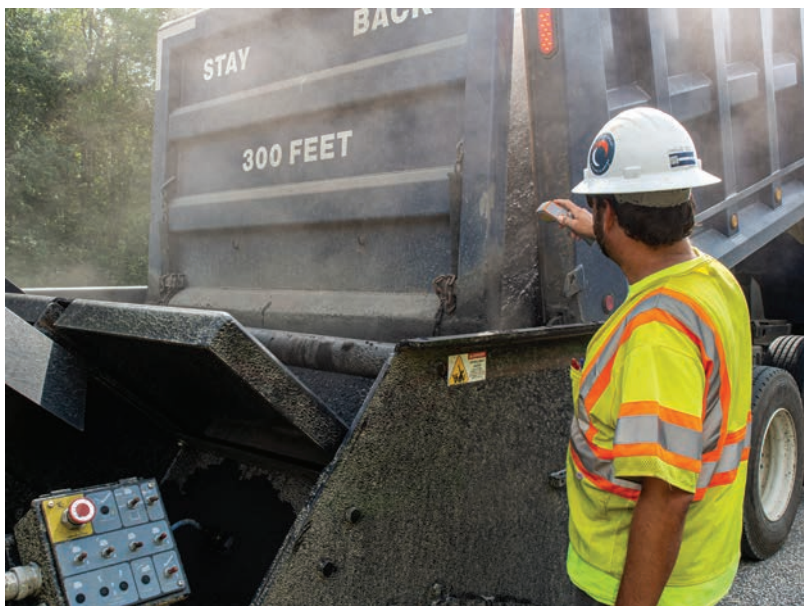
Assistant Research Engineer Grant Julian verifies mixture temperature for Section N6.
