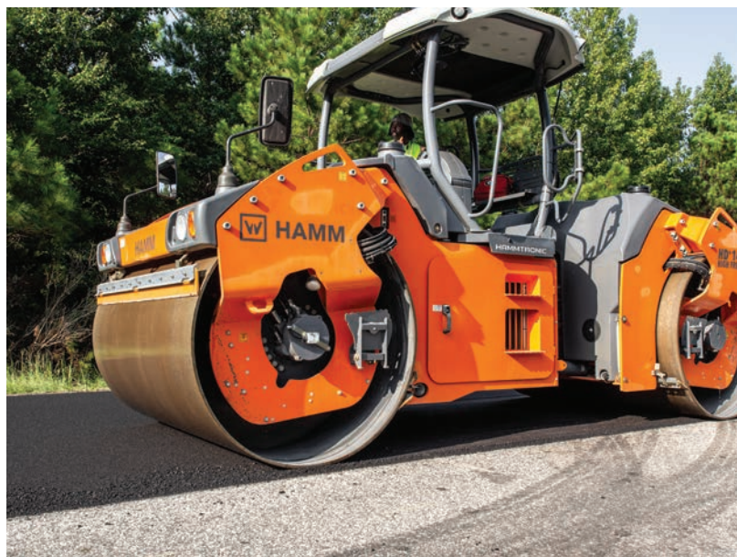
Oklahoma's Section N9 is compacted by a vibratory smooth drum roller.
