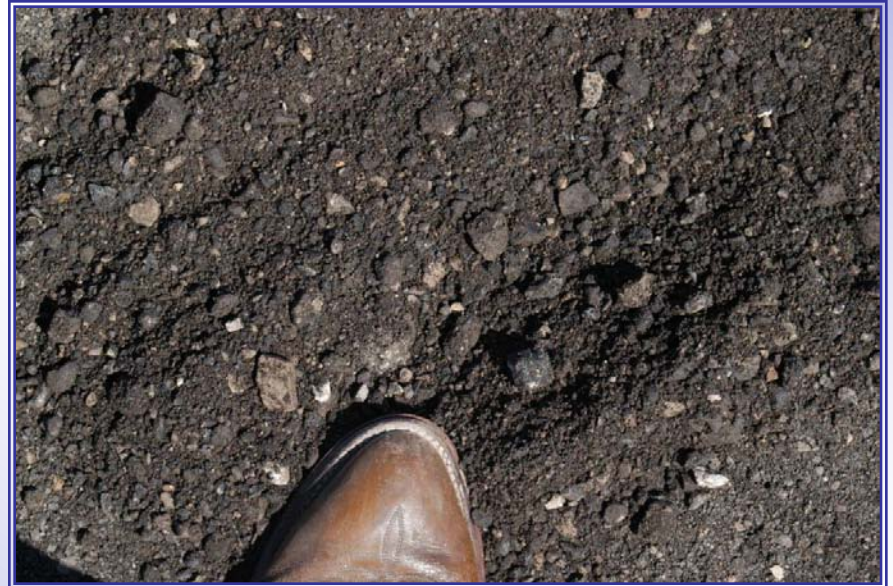
RAP after Soil Stabilizer
