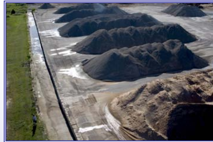
Paved /Sloped Surface
