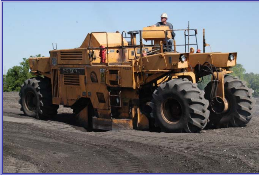
RAP Processed with Soil Stabilizer
