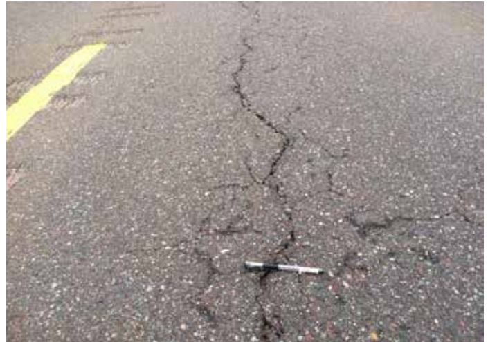
Figure 1 Pavement Cracking
