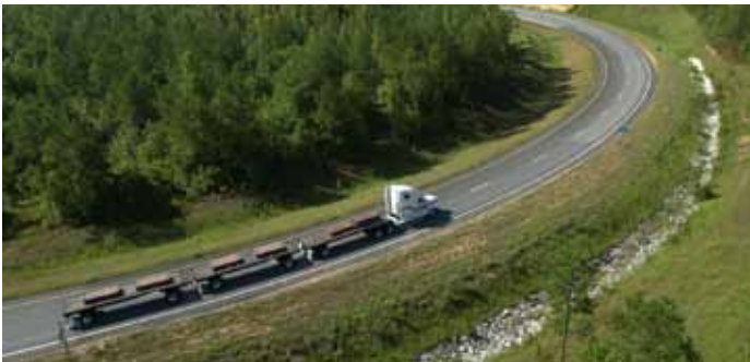
Figure 1. NCAT test track
