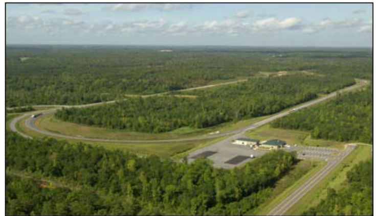
Figure 2. Aerial photo of the NCAT Test Track
