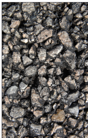
Figure 1 Close-up of OGFC on NCAT Pavement Test Track.
