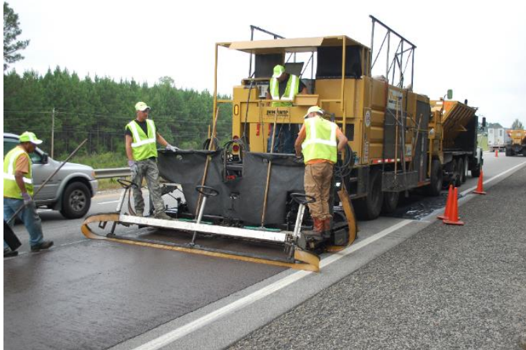
Figure 24. Micro surfacing application.
