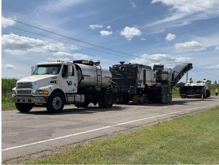
Figure 46. 70 th Street CIR equipment train.
