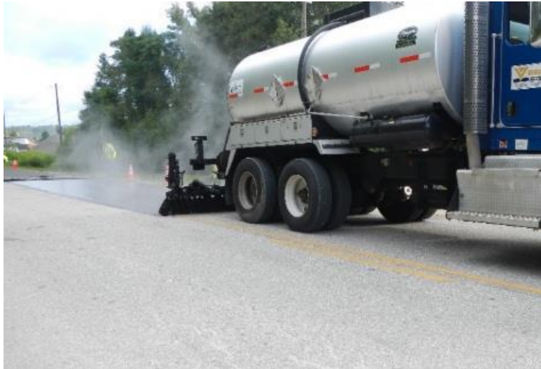
(a) Asphalt emulsion application
