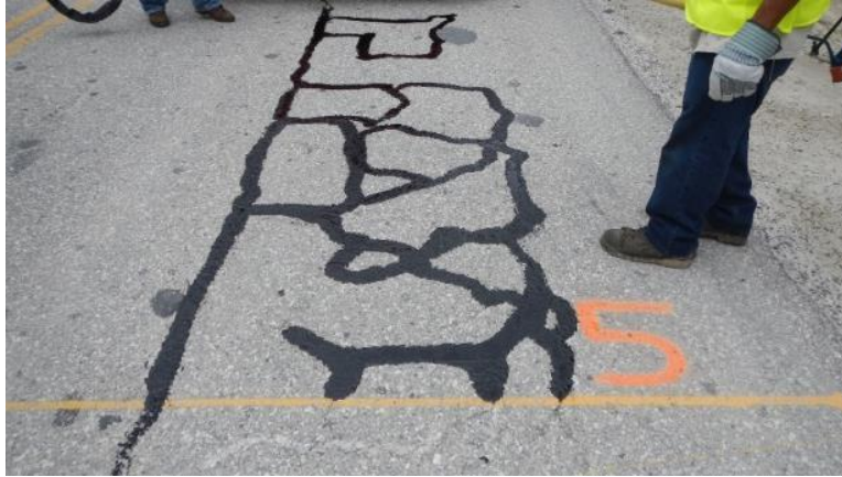
Figure 7. Crack sealing with overband configuration.
