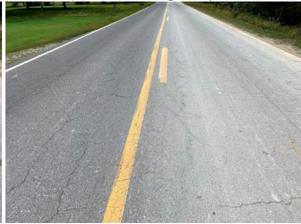
(f) Crack sealing + micro surfacing
