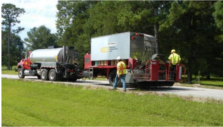
Figure 17. Fibermat® installation.
