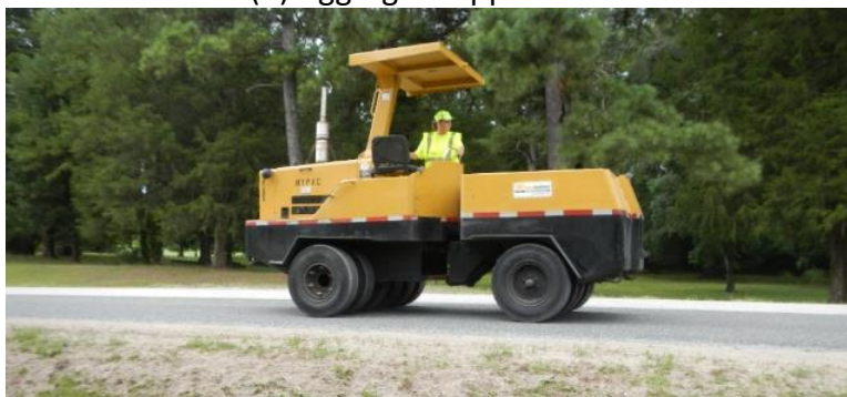
(c) Rolling newly placed chip seal with pneumatic roller
