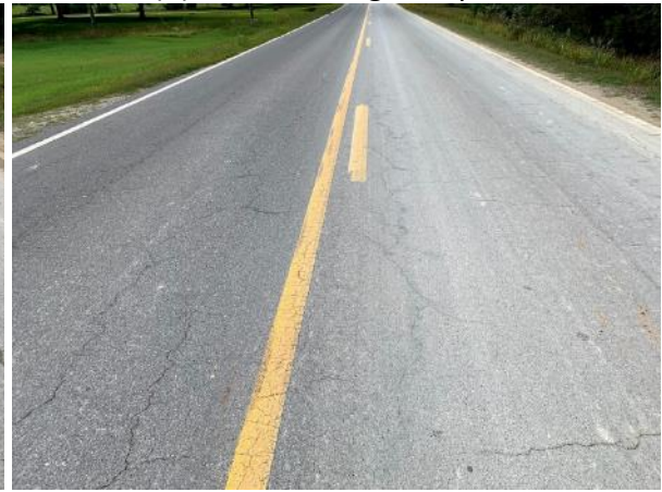
(f) Crack sealing + micro surfacing
