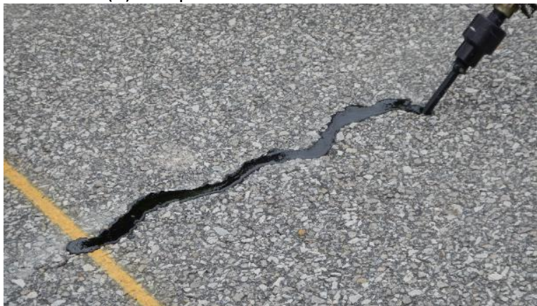
(c) Crack sealing
