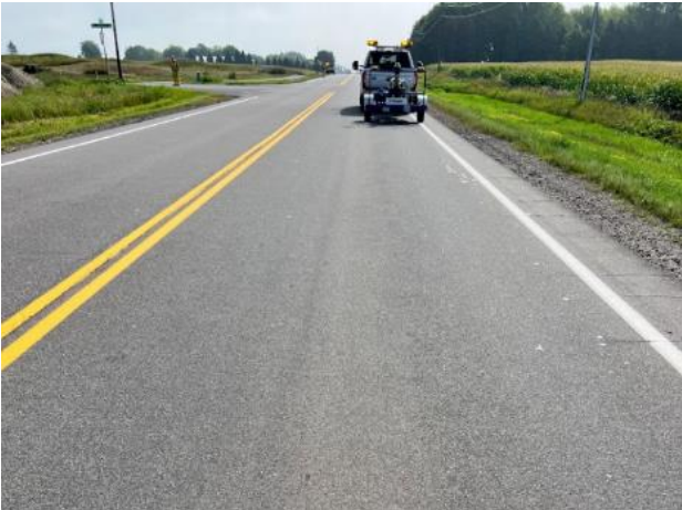
(a) CCPR – foamed asphalt
