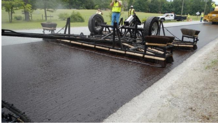
Figure 19. Scrub seal application.
