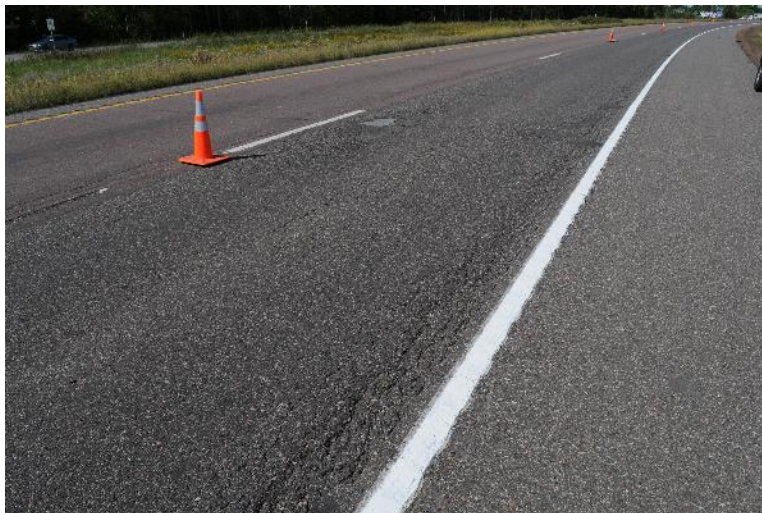
Figure 52. US-169 control section condition before resurfacing.
