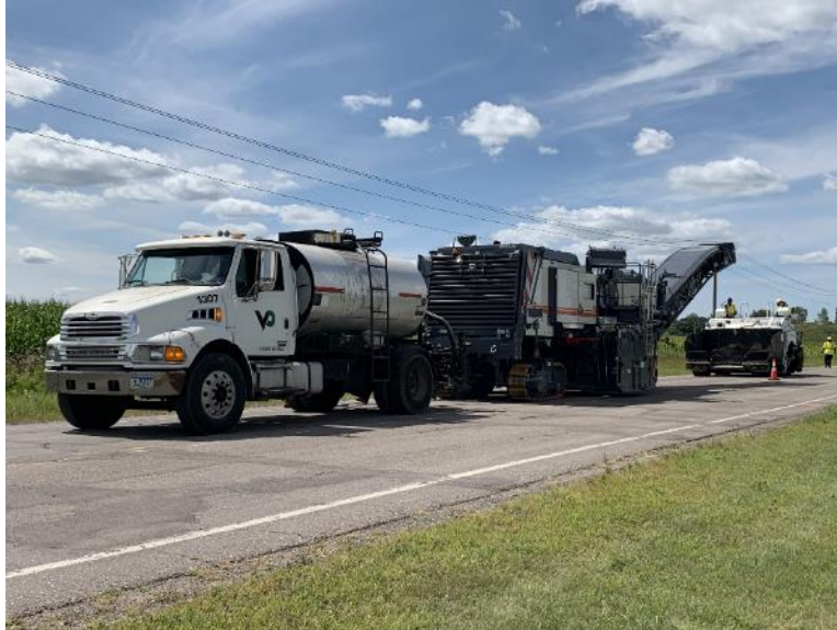
Figure 46. 70 th Street CIR equipment train.
