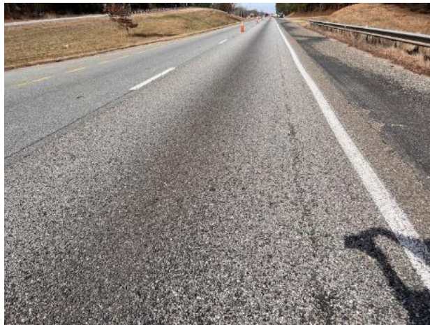
(a) CBC-1H (Spray paver)
