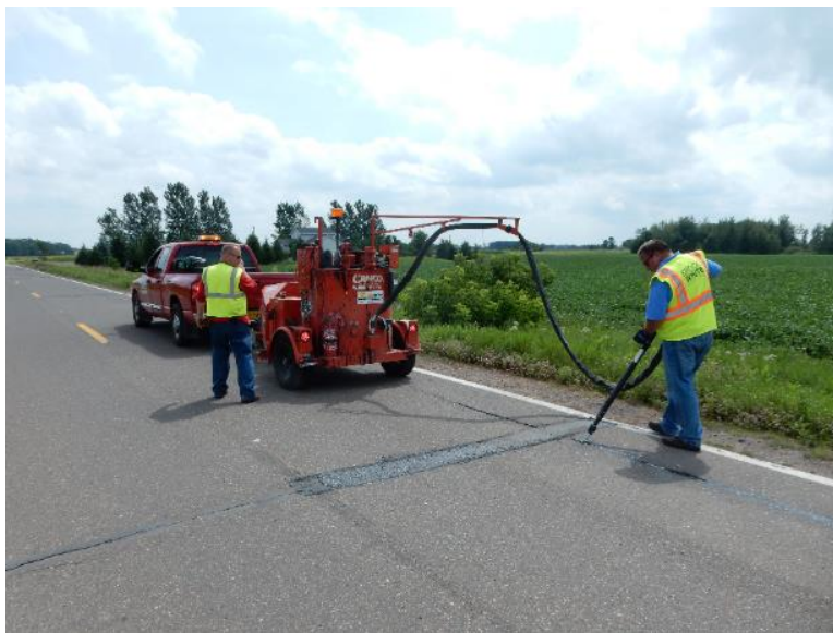
Figure 8. Crack sealing and mastic treatments in CSAH-8 test section.
