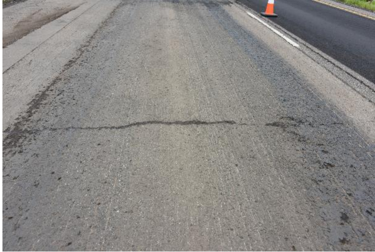
Figure 30. Milled surface of US-169 prior to thinlay application.
