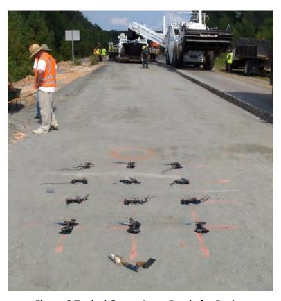
Figure 2 Typical Gauge Array Ready for Paving
