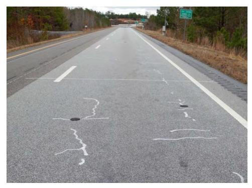
Figure 19 Photo of Typical Cracking Observed in GE Section on December 9, 2013
