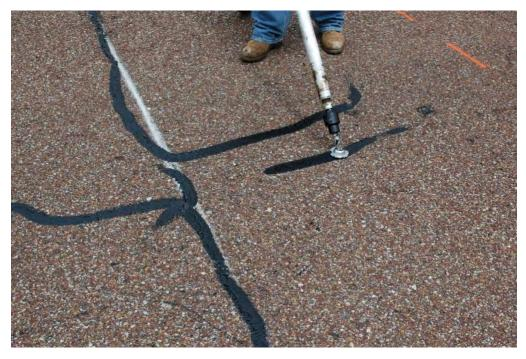
Figure 5 Blow/Band Crack Sealing in Section S2B
