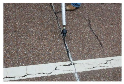
Figure 4 Filling Cracks in Section S2A
