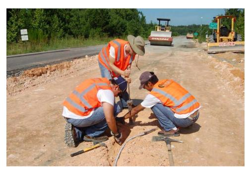
Figure 2 Installation of a Pressure Plate Before Placing the Aggregate Base
