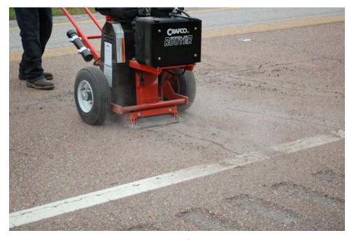
Figure 3 Routing Cracks in Section S2A
