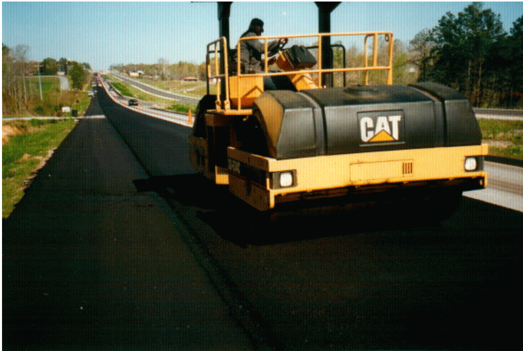
Figure 3. Alabama Hwy 157 Construction
