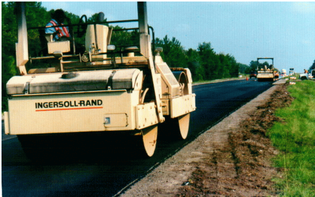
Figure 6. Florida Hwy 301 Construction
