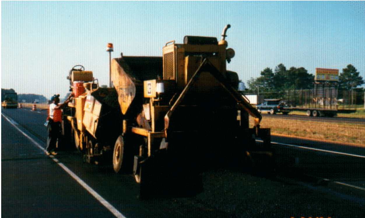
Figure 7. Mississippi Hwy 49 Construction
