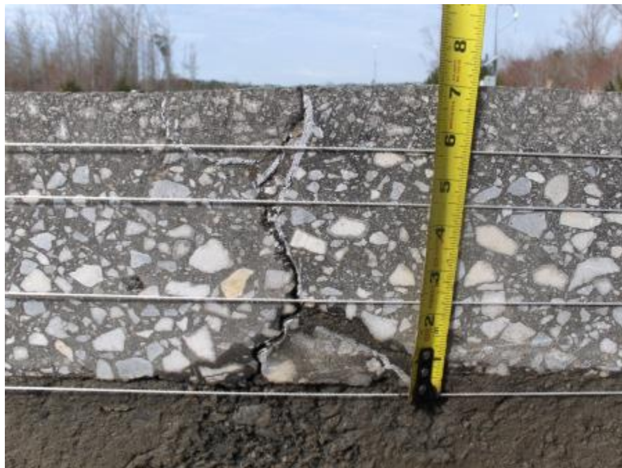
Figure 3 Example of Bottom-Up Fatigue Cracking Observed in Cross-Section.
