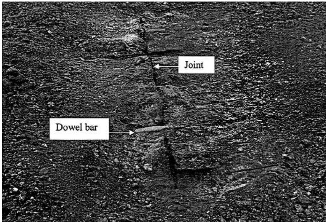
**Figure 2.3, Photo Showing Only Partial Destruction of Joint Integrity [Baladi et al, 2002]**
