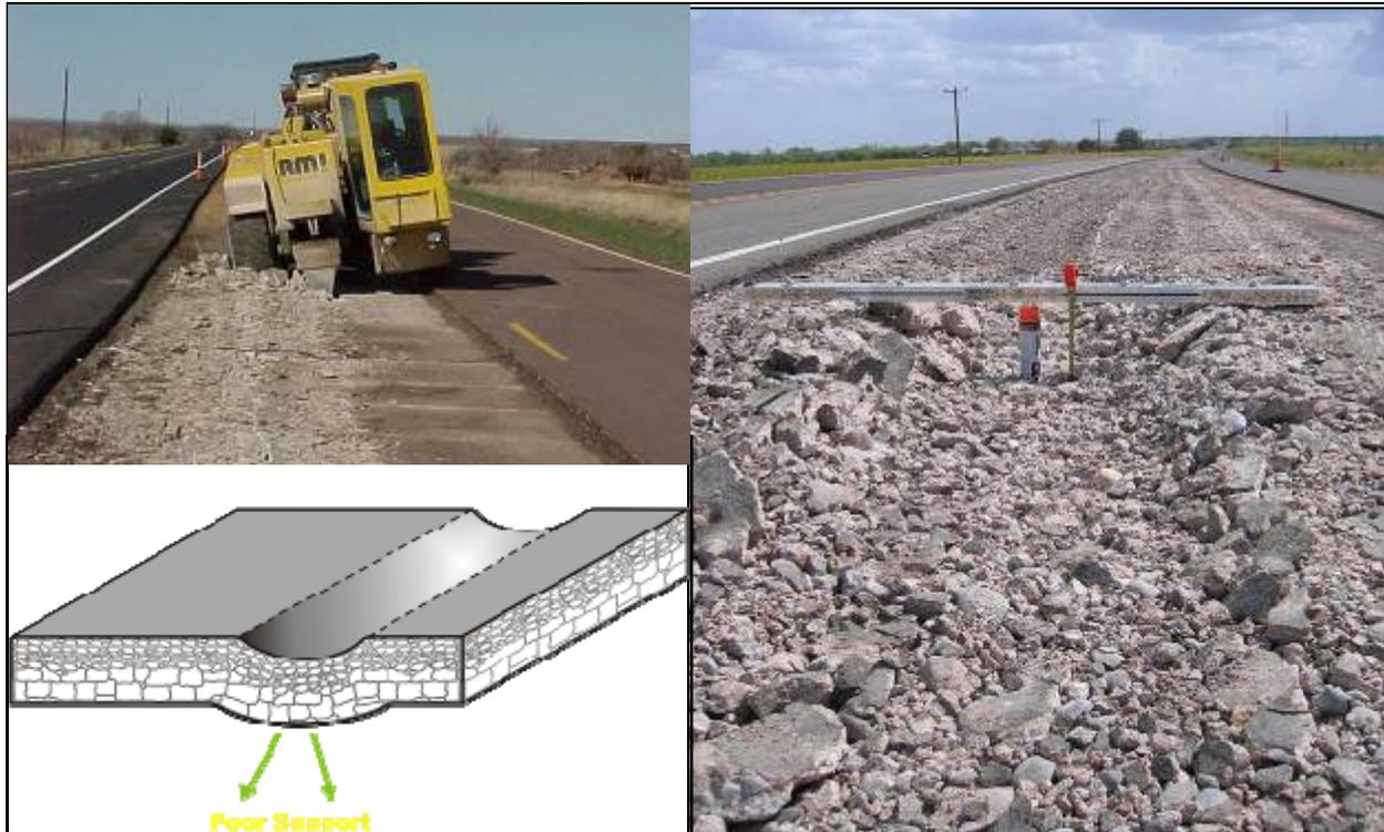
**Figure 3.13, RPB Causing Rutting Failures on a Texas Highway**
