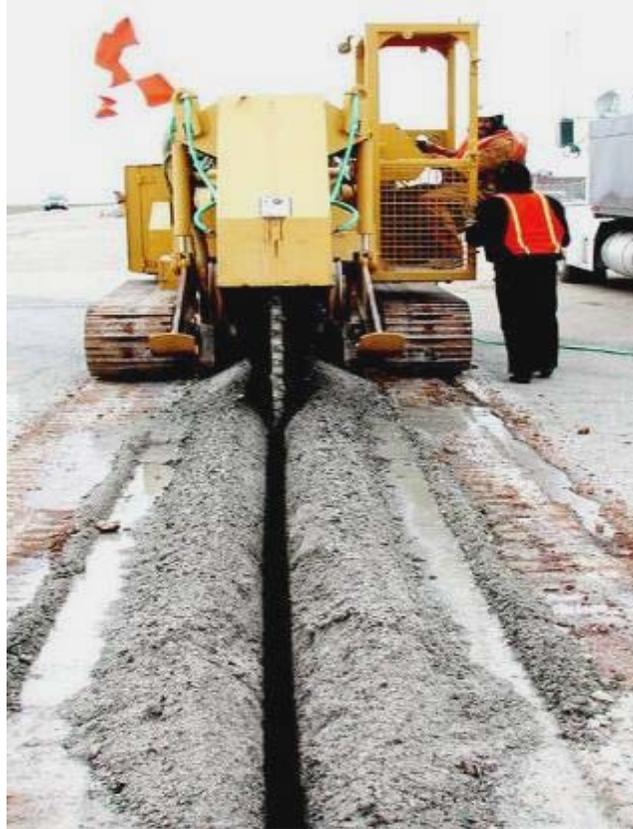
**Figure 6.2, Isolation Cut and Relief Trench by Wheel Saw**
