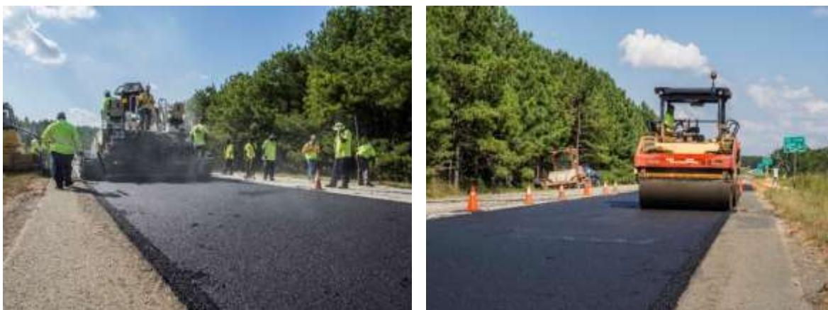
FIGURE 3 Laydown and compaction of S1 base mix.
