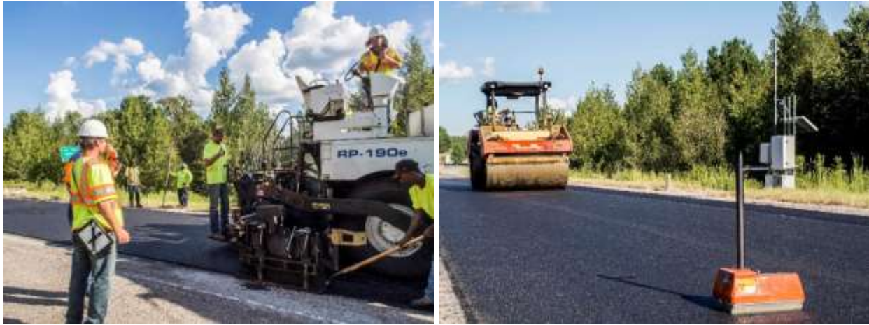
FIGURE 5. Constructing Section S11 with a volumetric mix.
