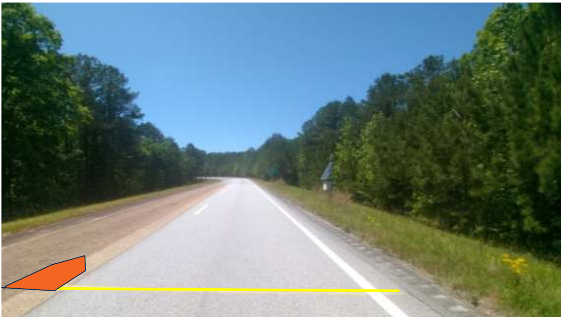
FIGURE 17 Subsection N13-B ARGG, 0.35-inch rutting, 3.1% cracking (April 2024).
