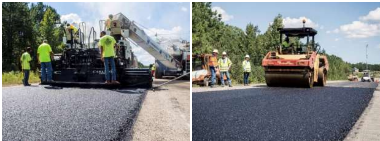
FIGURE 4. Constructing Section S10 with a BMD mix.
