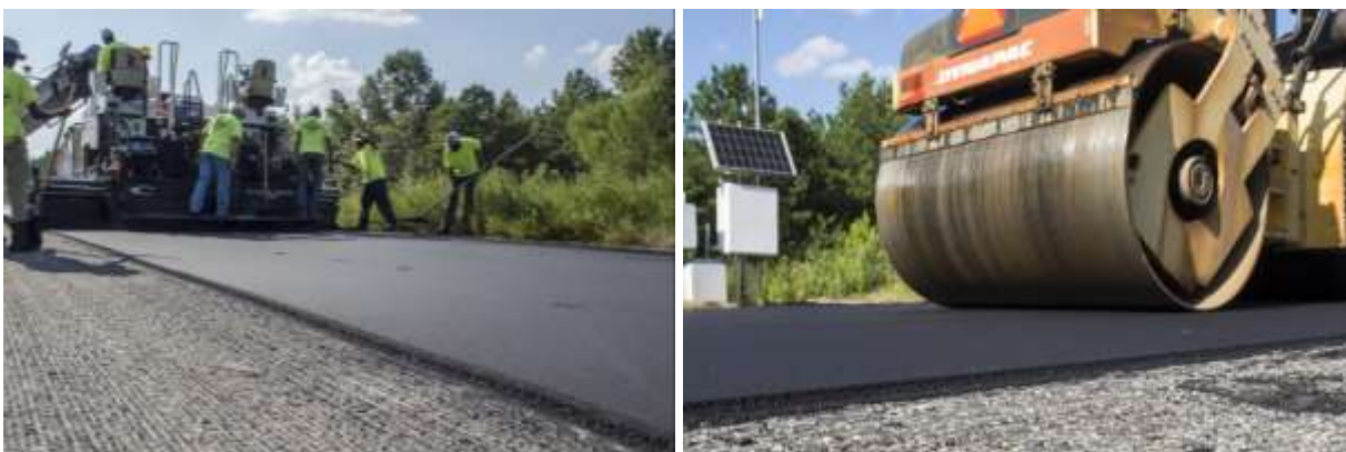
FIGURE 2 N11 mix placement and compaction.
