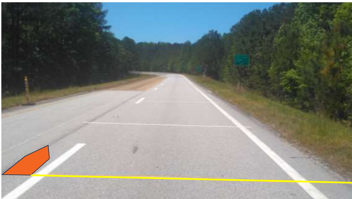
FIGURE 15 Subsection N12-C virgin chip seal, 0.21-inch rutting, no cracking (April 2024).
