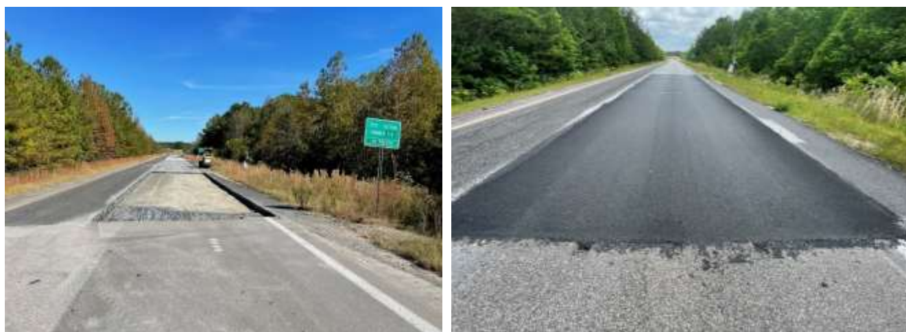
Figure 11. Partial Reconstruction of Section S8 (October 2022)
