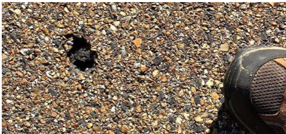
FIGURE 5 Pop-out in Section S2.
