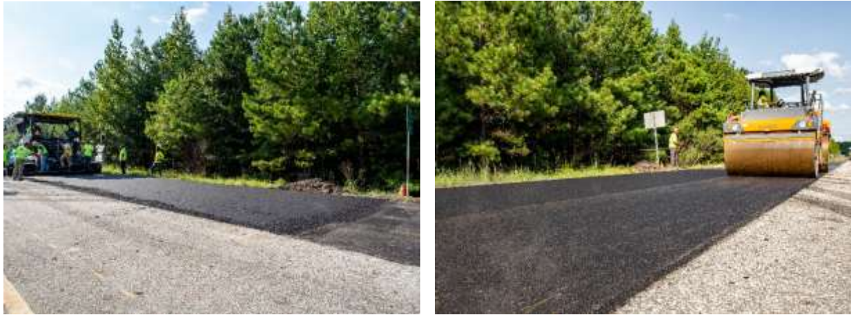
FIGURE 16 Laydown and compaction of N9 surface mix.
