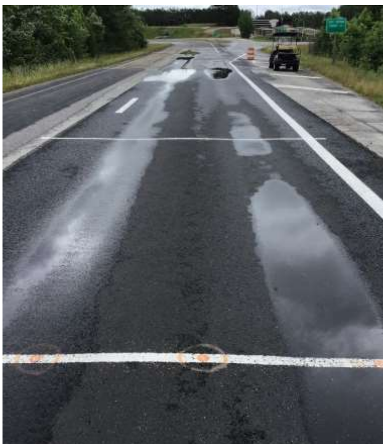
FIGURE 6 Rutting in Section S12 (April 2022).
