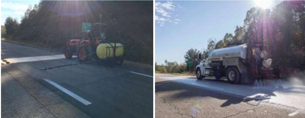
FIGURE 1 S3-A and S3-B application of spray-on rejuvenators.
