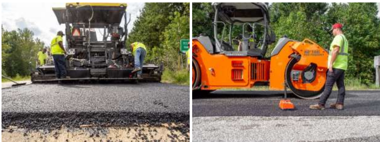
FIGURE 6. Constructing Section N6 with a BMD mix.
