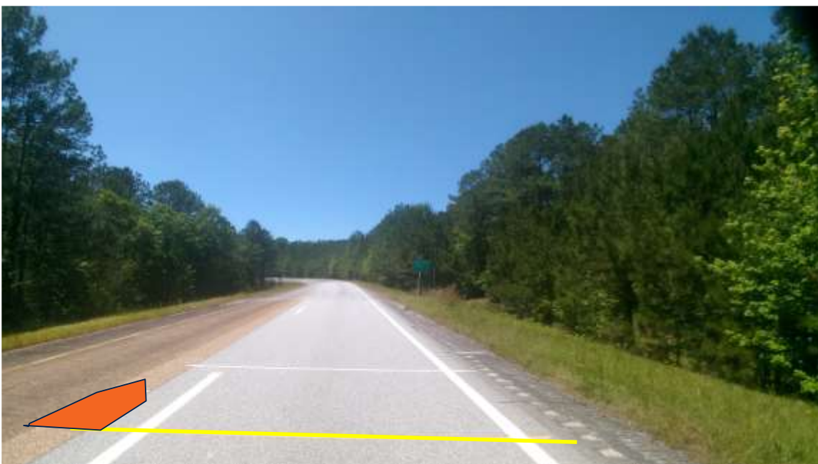
FIGURE 18 Subsection N13-B OGI, 0.19-inch rutting, 0.8% cracking (April 2024).
