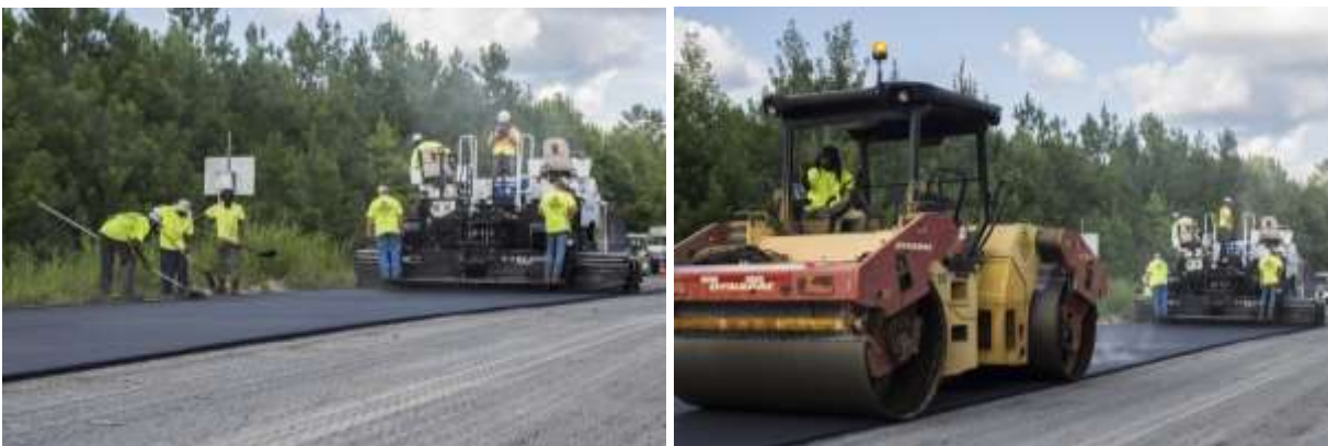
FIGURE 1 N10 mix placement and compaction.
