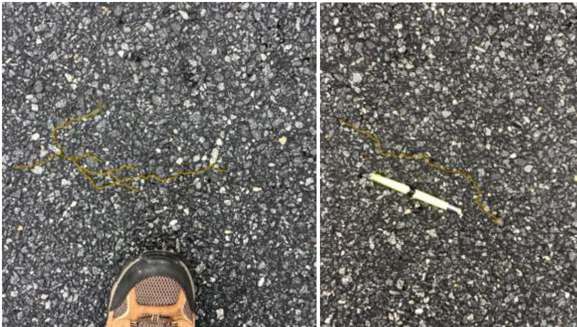
FIGURE 2 Sample cracking in N4 on 1/25/2021 (29.6 million ESALs).
