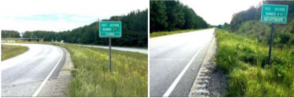
FIGURE 2 Paving of Sections E5A and W10.
