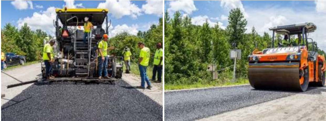
FIGURE 5 Construction of Section S7A.
