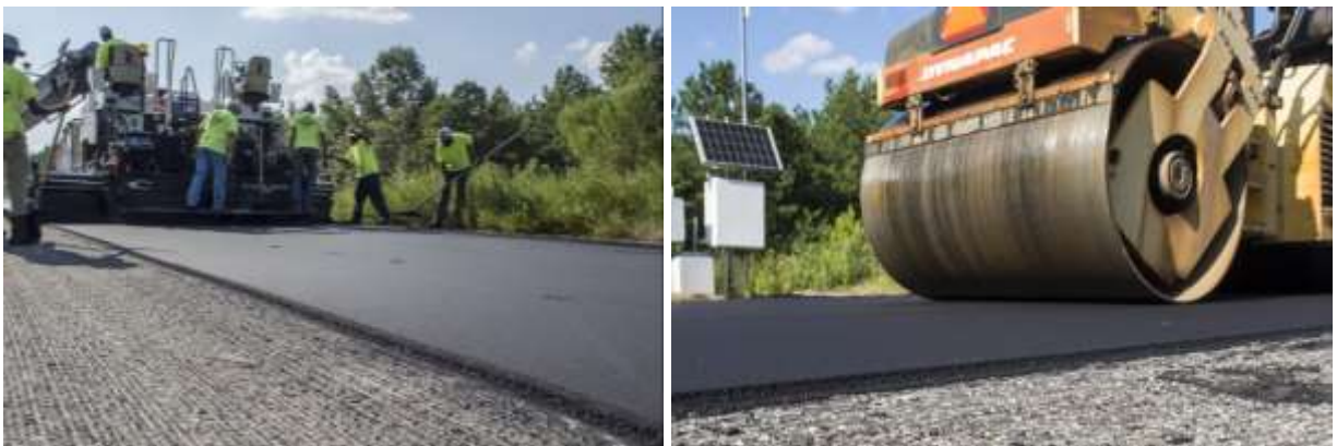
FIGURE 2 N11 mix placement and compaction.
