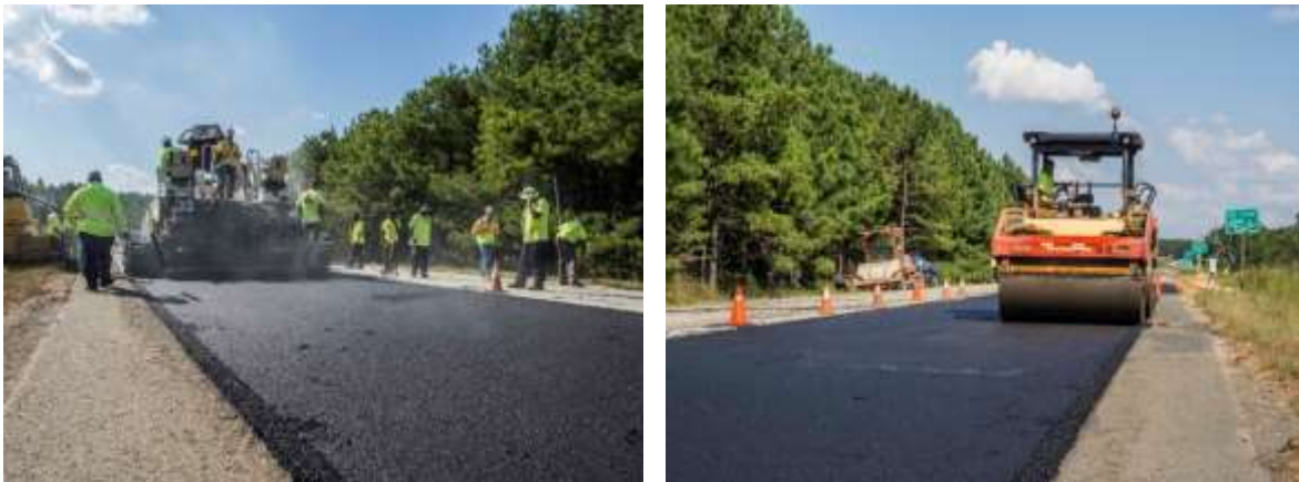
FIGURE 3 Laydown and compaction of S1 base mix.
