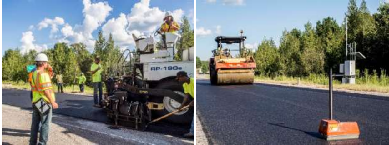
FIGURE 5. Constructing Section S11 with a volumetric mix.
