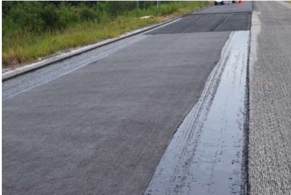
FIGURE 2 Section N12-B geosynthetic PETROMAT® (foreground) and N12-A GlasGrid® (background) interlayers.
