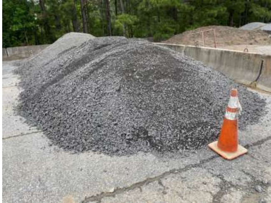
FIGURE 3 Stockpiled reclaimed CCPR millings.
