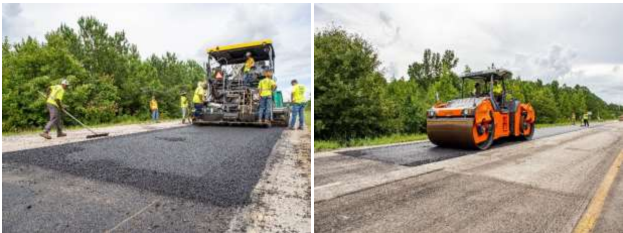
FIGURE 6 Construction of Section S7B.
