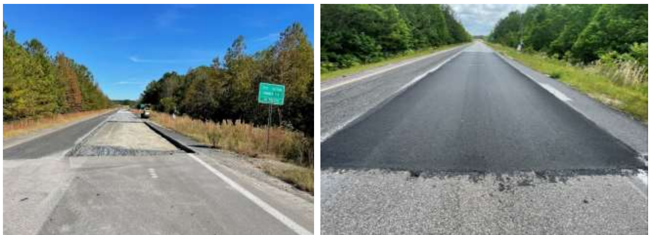
Figure 11. Partial Reconstruction of Section S8 (October 2022)
