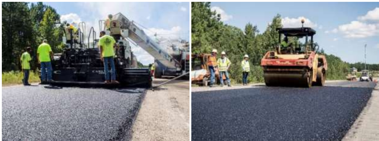
FIGURE 4. Constructing Section S10 with a BMD mix.
