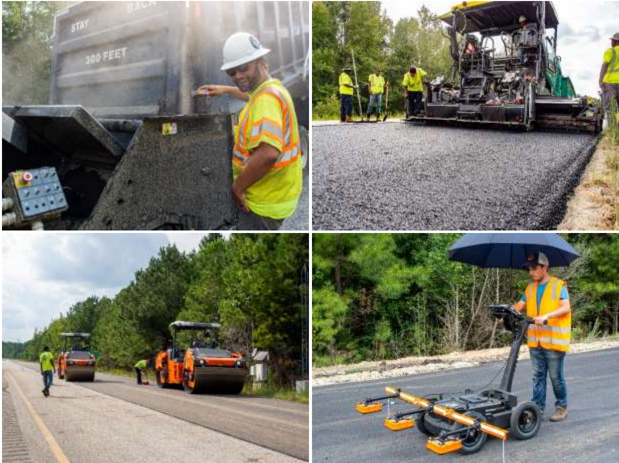
FIGURE 6 Paving test section N6 for the 2021-2024 research phase.
