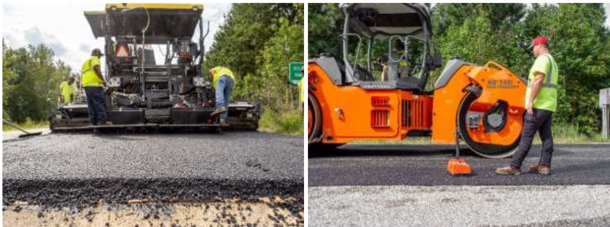
FIGURE 6. Constructing Section N6 with a BMD mix.
