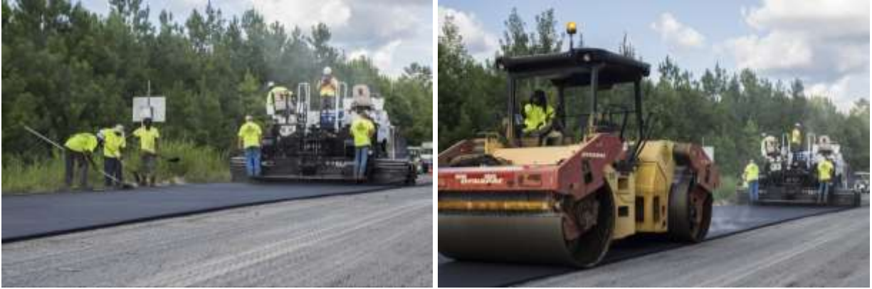
FIGURE 1 N10 mix placement and compaction.
