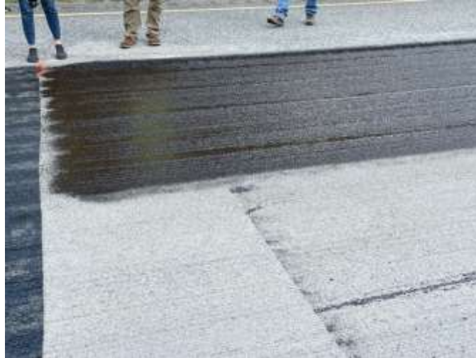
FIGURE 3 Tack coat application after milling in Section W4.
