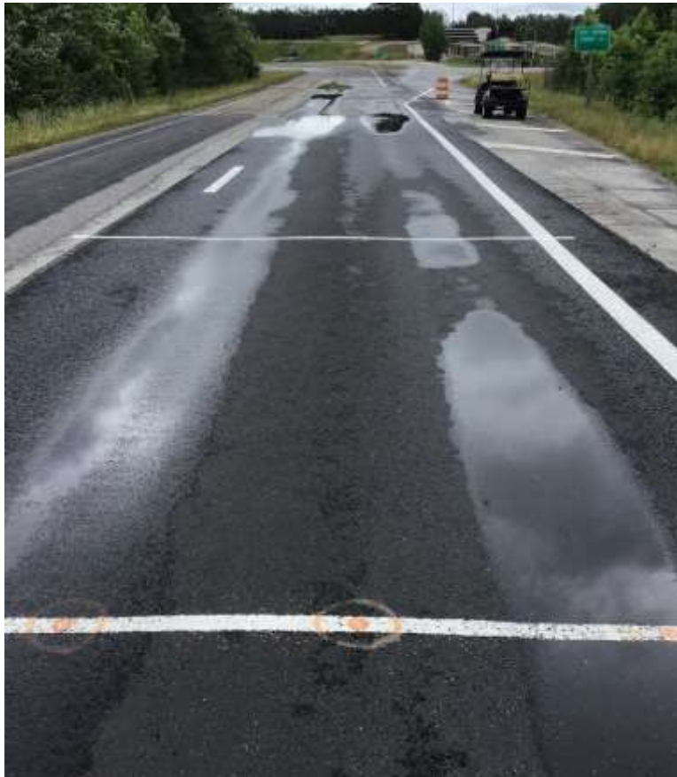
FIGURE 6 Rutting in Section S12 (April 2022).
