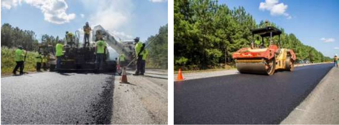
FIGURE 4 Laydown and compaction of S1 surface mix.
