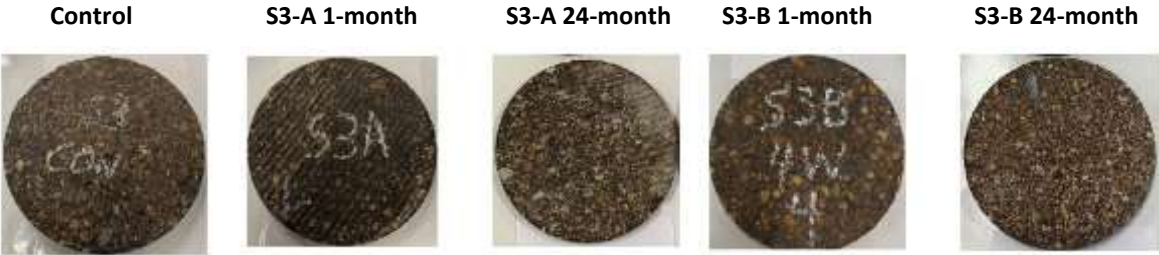
FIGURE 3 Section S3 pavement surfaces 1 month and 24 months after treatment application.
