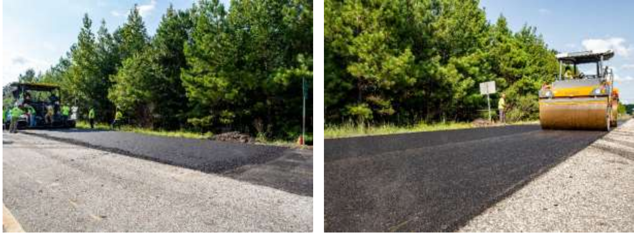
FIGURE 16 Laydown and compaction of N9 surface mix.
