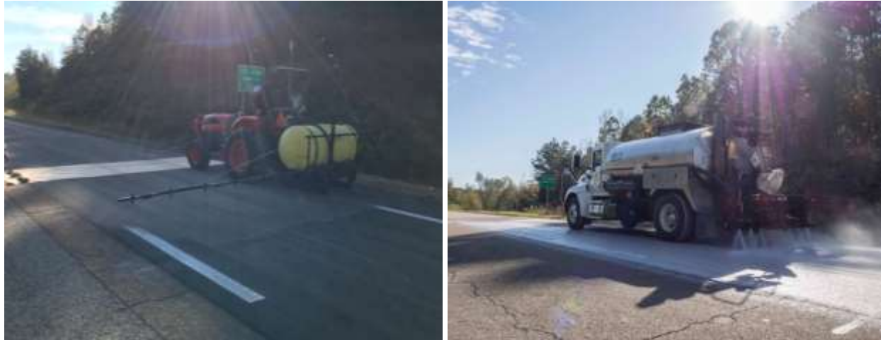
FIGURE 1 S3-A and S3-B application of spray-on rejuvenators.
