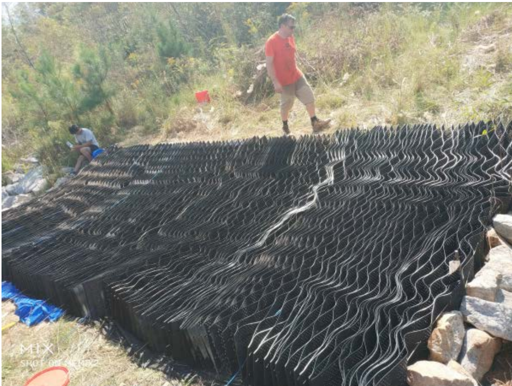
Figure 14 – Installation of the CCS in the region cleared from vegetation
