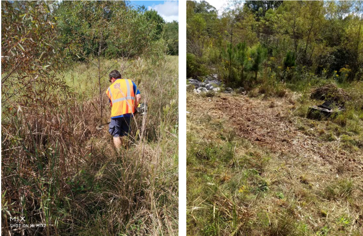
Figure 11 – Clearing of vegetated channel
