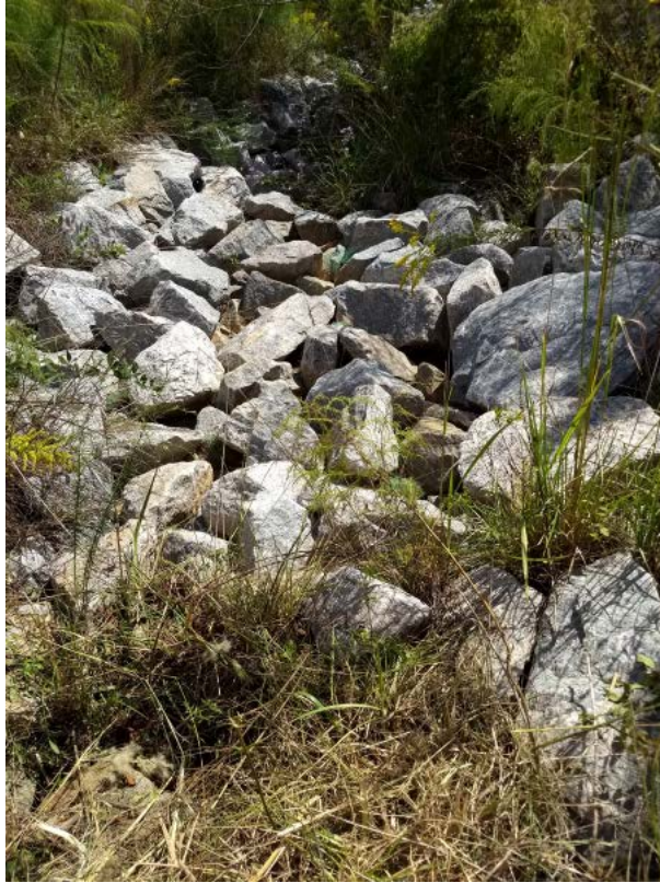
Figure 13 – Transition between the cleared channel and the beginning of the rip-rap lined channel.
