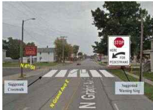
Figure E-96. Suggested mid-term treatments for un-signalized intersections.
