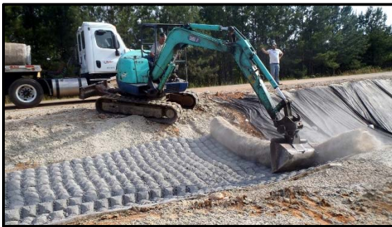
(e) Flexamat Installation
