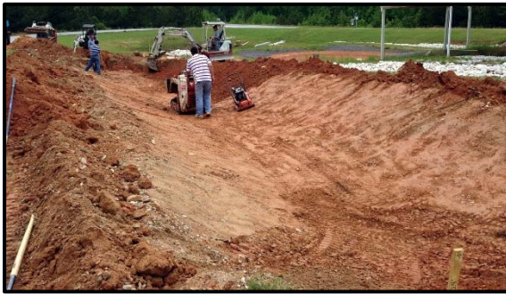
(c) Channel Compaction
