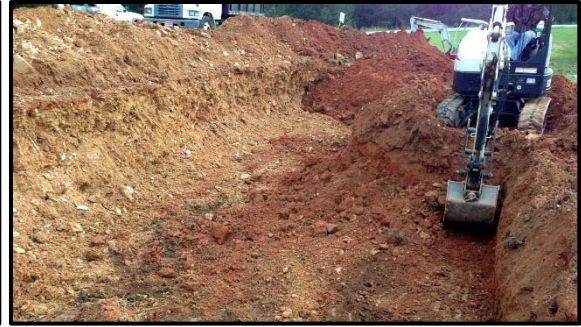
(b) Sediment Basin Excavation
