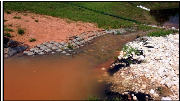
(b) spillway breach
