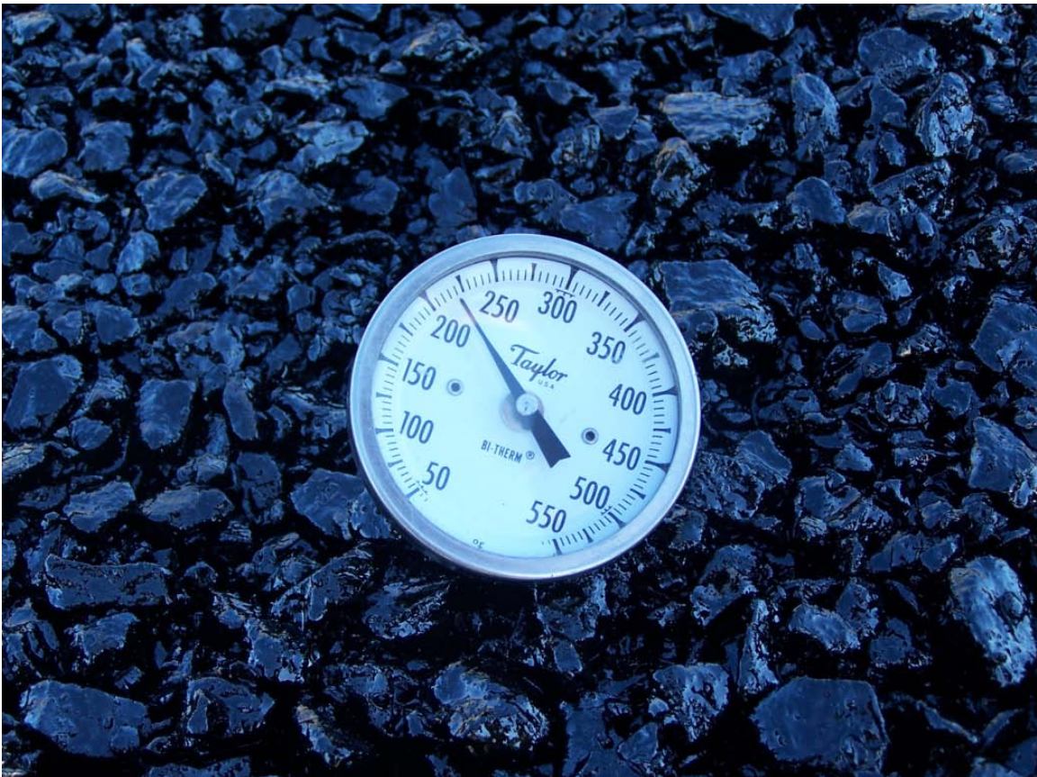
Figure 4-1. Temperature of Freshly Paved PATB on US 280.
