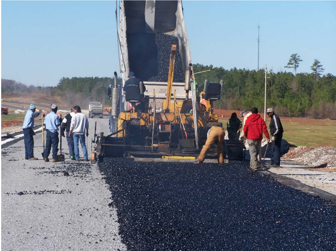
Figure 1-1. PATB Paving on US 280 near Camp Hill, Alabama.
