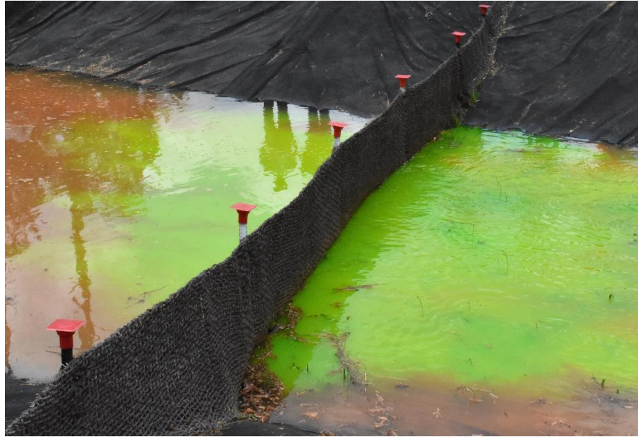
Figure 2.5: AU-SRF Sediment Basin Subjected to Green Dye to Show Baffle Performance.
