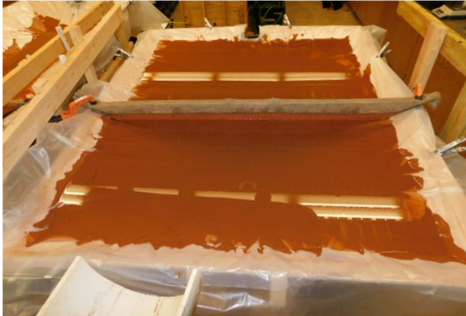
Figure 3.32: Undersized Basin: Flocculant, Single Coir Baffle, and No Skimmer.
