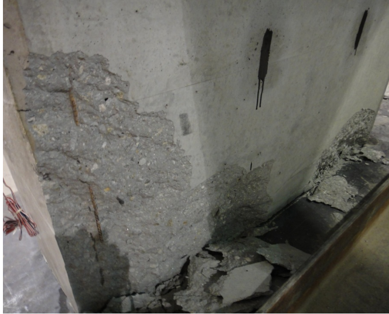
Figure 4-9 Initial Spalling on Bridge Leg
