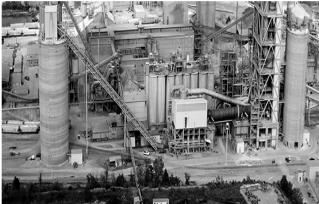
Figure 1-1: Full-Scale Portland Cement Production Facility (Folta 2010)
