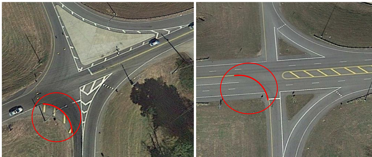
Figure 5. Examples: Left – Corner Radius Tangent to Crossroad Edge; Right – Corner Radius Tangent to Crossroad Median
