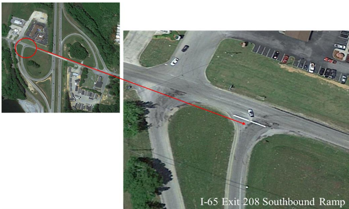
Figure B.4 High-Risk Exit Ramp Terminal of Parco Interchange
