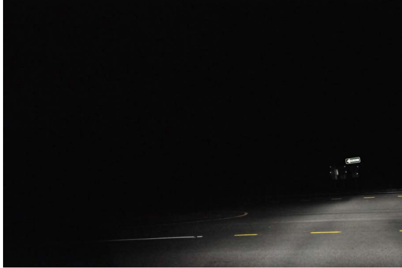
Figure 5.6 Example of DNE Signs Placed Too Far From the Nose of the Median in AL
