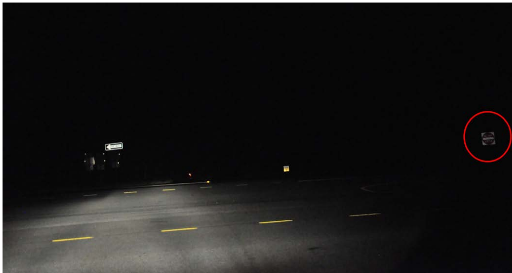
Figure 5.5 Example of an Improperly Oriented Sign in AL
