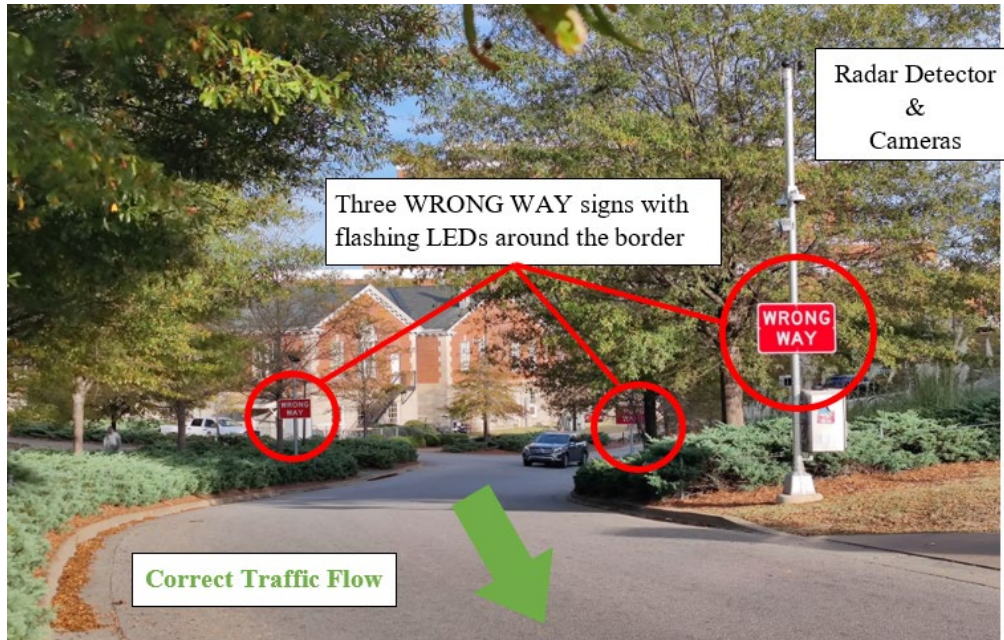
Figure 2 Wrong-way alert system configuration
