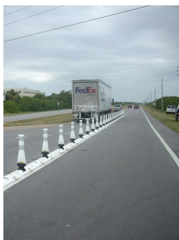
Figure B-11 (a) Qwick curb and (b) RIGHT TURN ONLY sign
