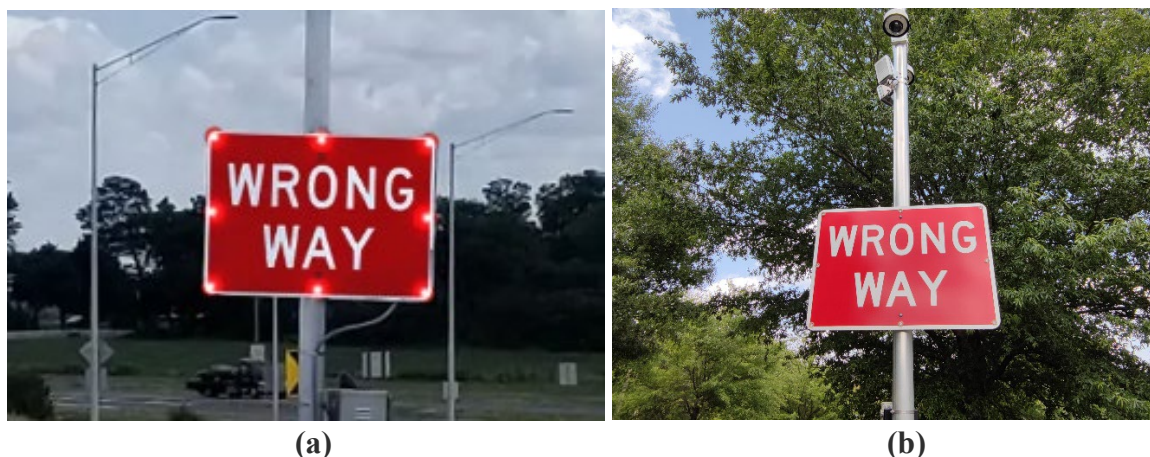
Figure D-2 (a) WRONG WAY sign with flashing LEDs around the border, and (b) Flashing LEDs were turned off
