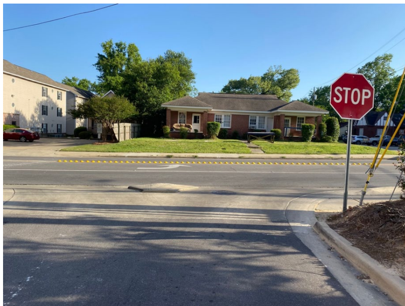
Figure C-4 Driver's View of Stop Sign and Raised Markers
