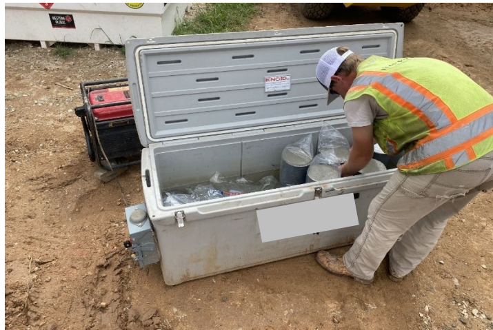
Figure 5-3: Example of Contractor Curing Environment
