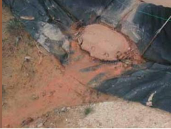
(b) lack of protection from sun and sediment [A]
