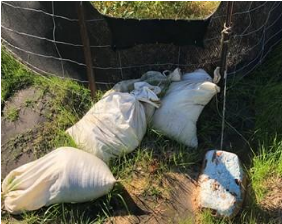
(c) incorrect placement of flocculant
