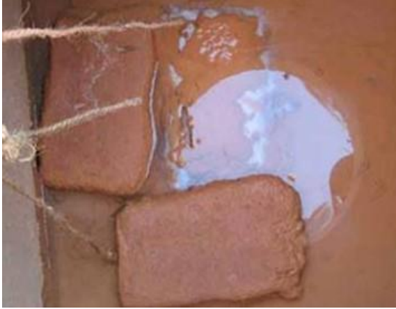
(a) improper maintenance in storm drain inlet [A]
