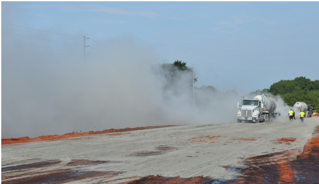
Figure 2.12: Cement Dusting into the Air
