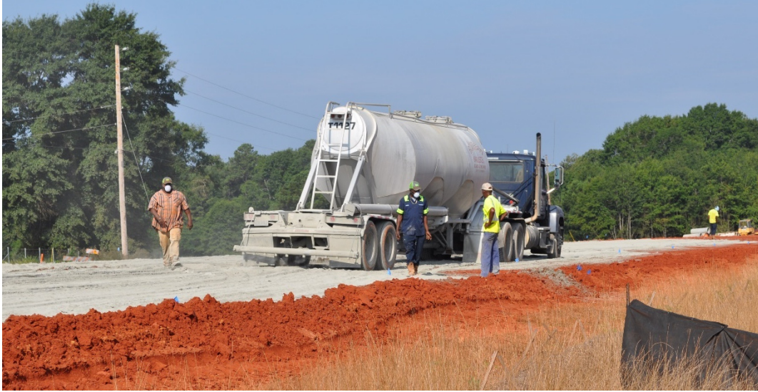
Figure 2.11: Cement Being Spread by Mechanical Spreader
