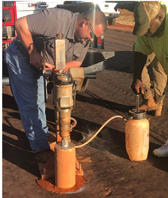
Figure 2.23: Core Removal Process
