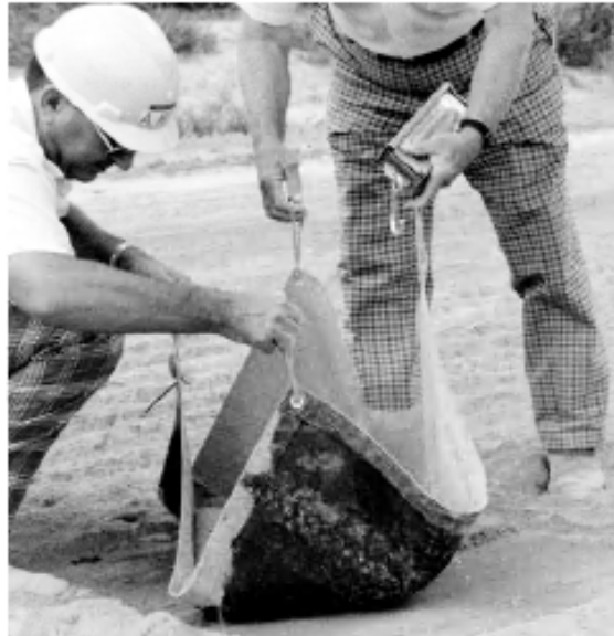
Figure 2.19: Cement Content being Checked (ACI 230 2009)
