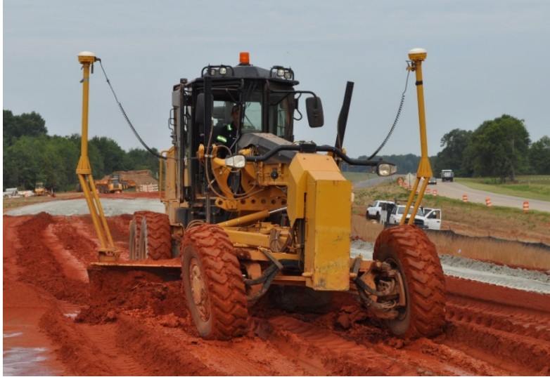
Figure 2.15: Motor Grader Spreading Soil Cement
