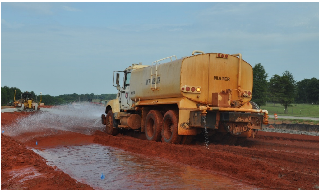
Figure 2.13: Water Truck Applying Water to Soil Cement
