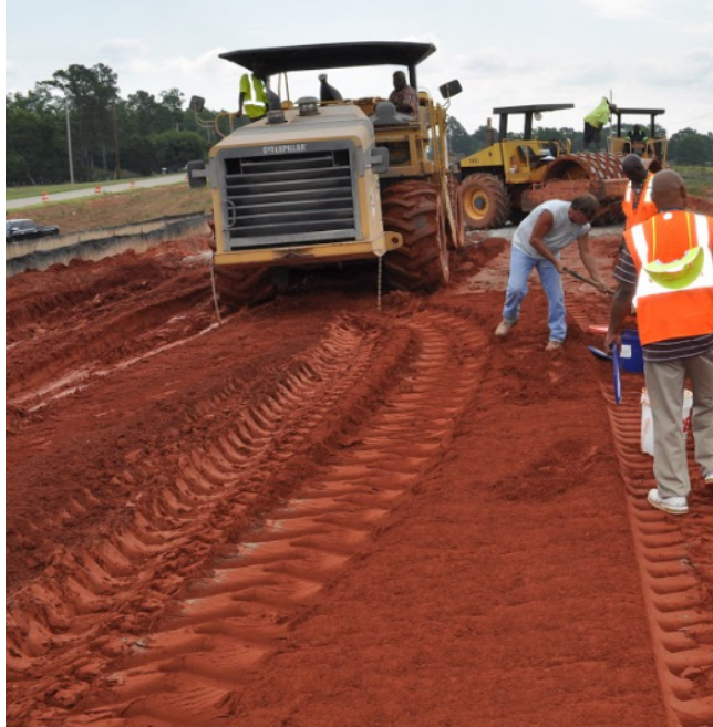
Figure 3.26: Material Ready to be Sampled for PM Cylinder Production
