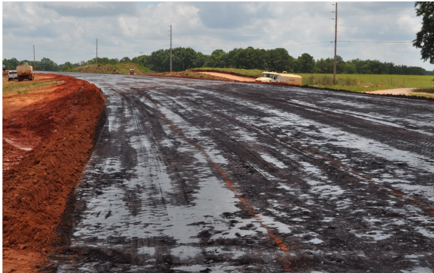
Figure 2.18: Emulsified Asphalt Coating the Compacted Soil Cement
