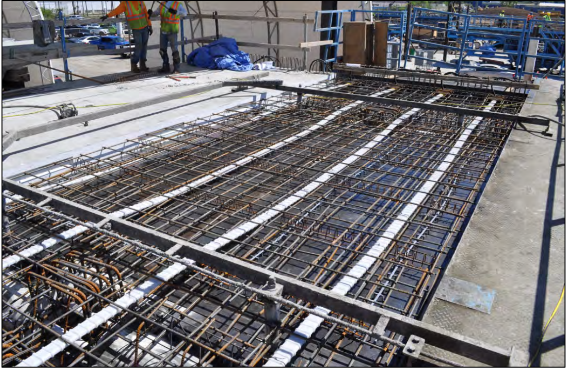
Figure 5-5: Formwork for a segment ready for concrete placement
