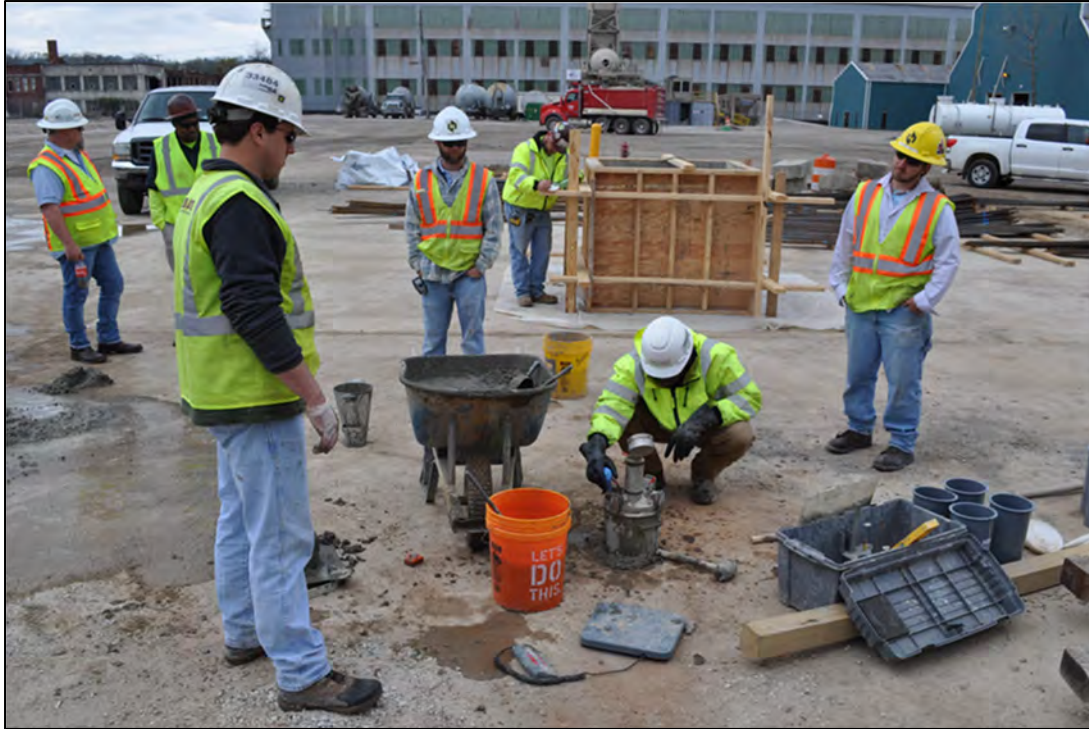
Figure 5-7: Quality assurance testing prior to concrete placement
