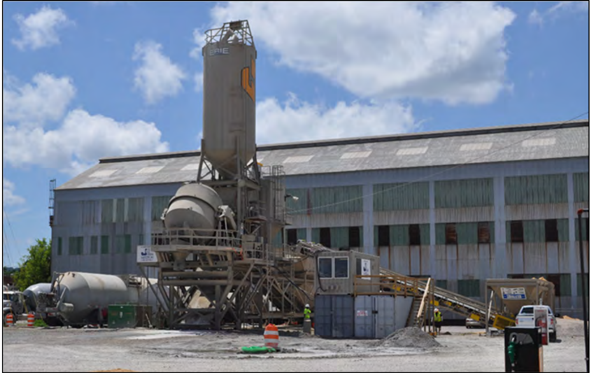
Figure 5-6: On-site batching plant for concrete production
