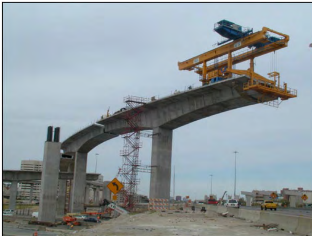
Figure 2-15: Balanced cantilever construction using mobile lifter (ASBI 2019)
