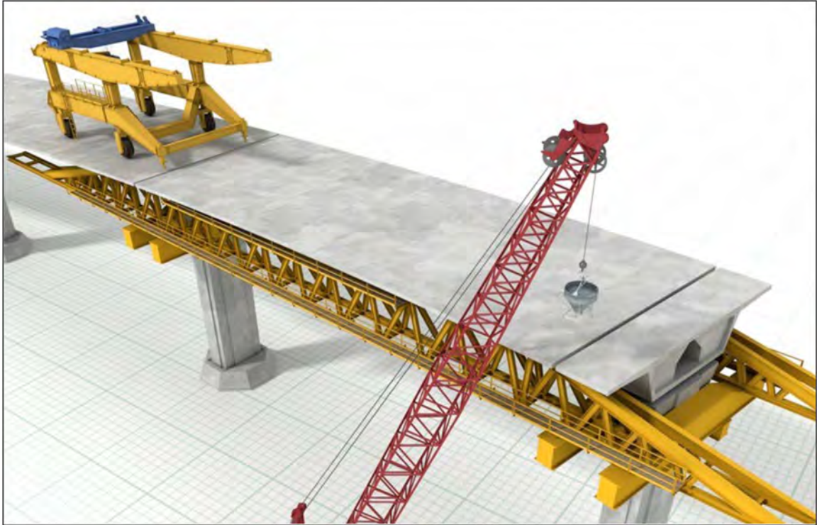
Figure 2-12: Cast-in-place closure joint (ASBI 2019)
