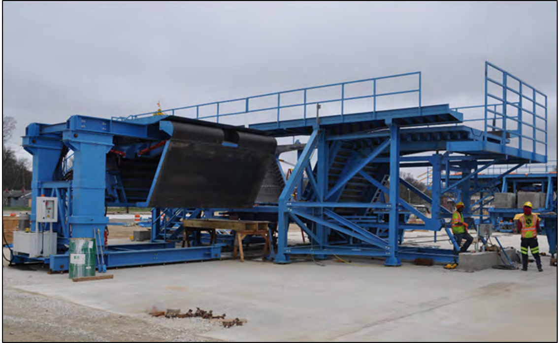
Figure 5-4: System on rails used to remove internal cell of the formwork
