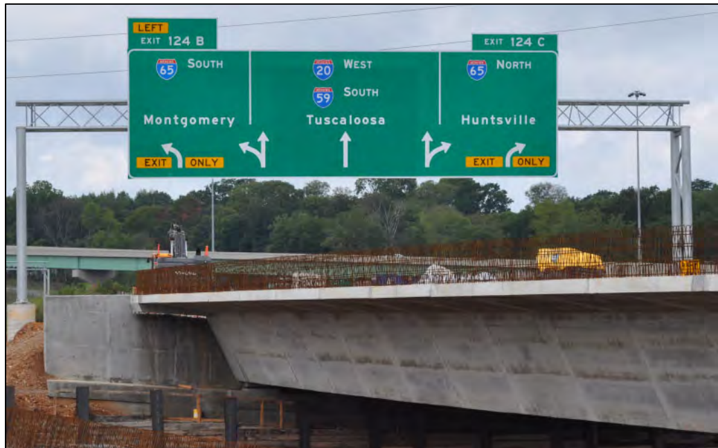
Figure 1-1: Birmingham I-59/I-20 segmental bridge during construction
