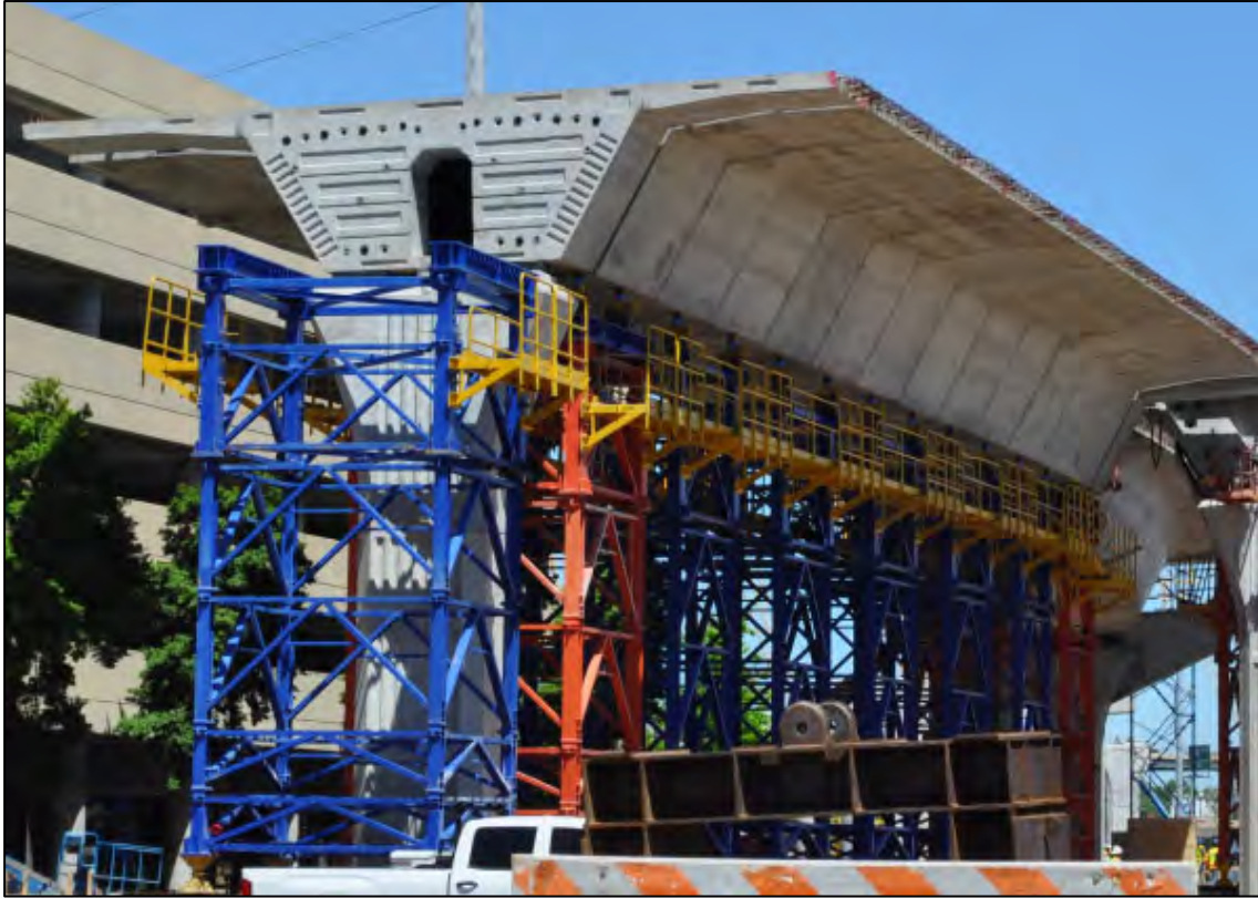
Figure 5-15: Falsework used to erect each span
