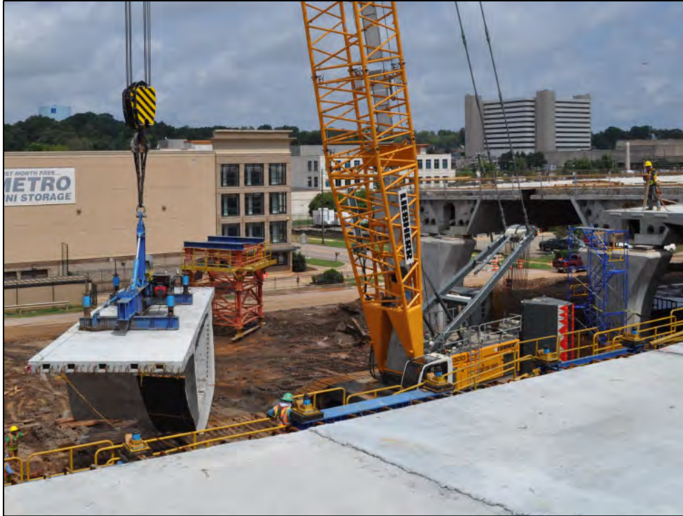
Figure 5-16: Crane lifting a segment into place
