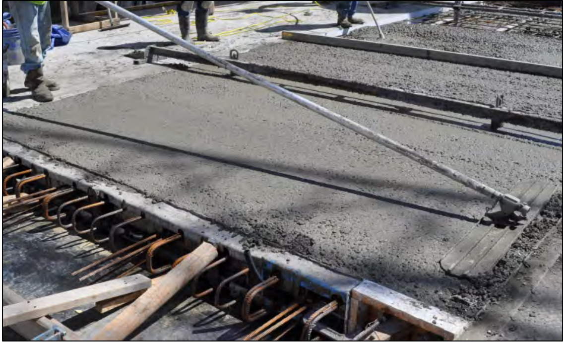
Figure 5-12: Concrete being floated using a bull float
