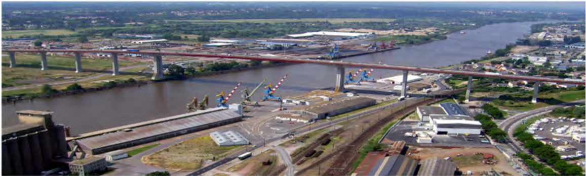
Figure 2-18: Bridge of Cheviré in France
