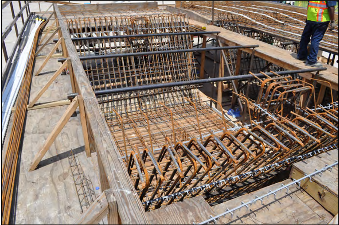
Figure 5-3: Reinforcement fabrication box for increased construction efficiency
