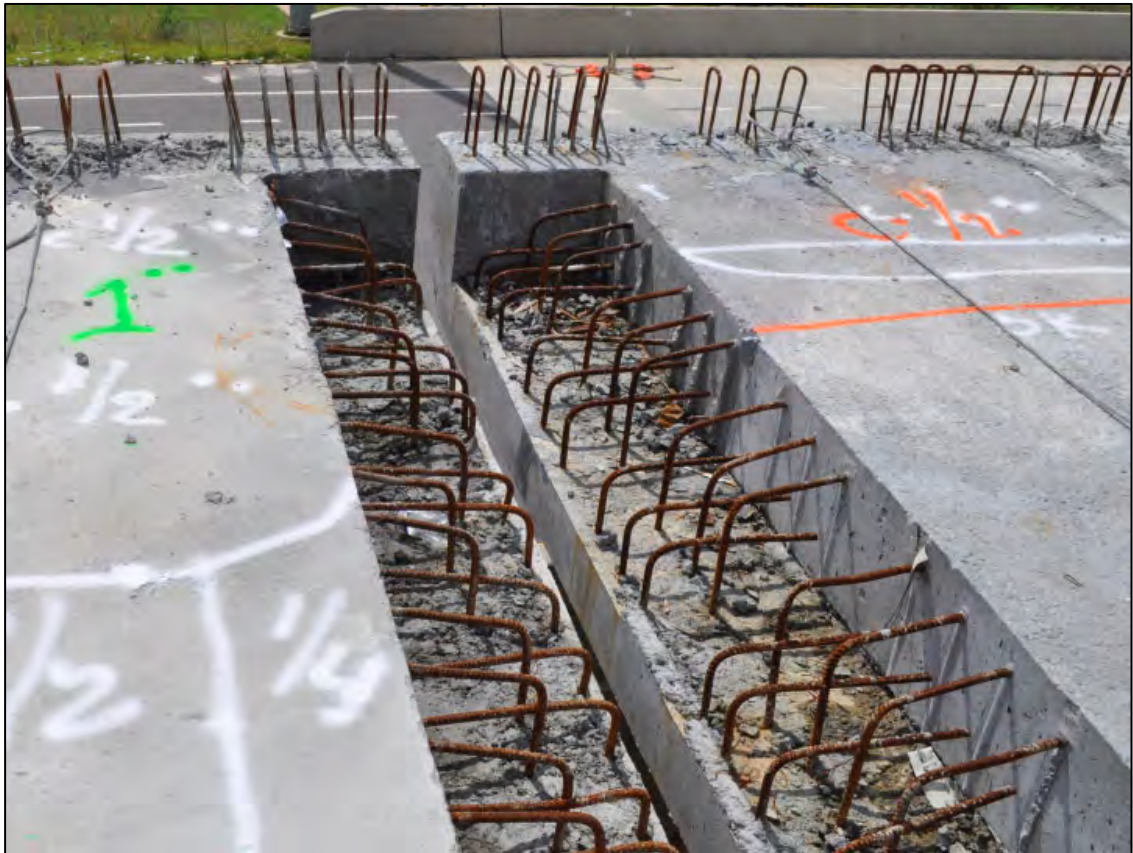
Figure 5-18: Closure strip between two spans to be filled with concrete
