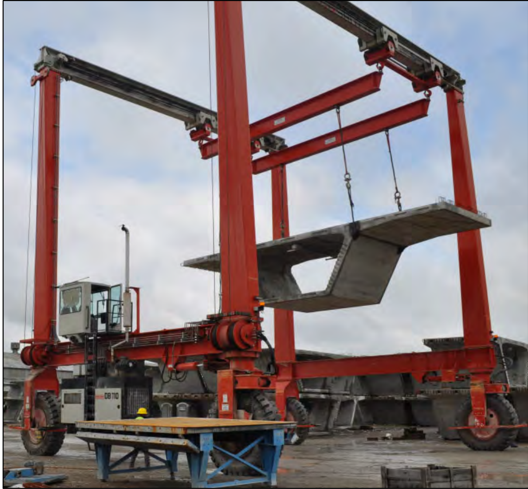
Figure 5-14: Rubber-tired gantry crane used to transport segments around the casting yard
