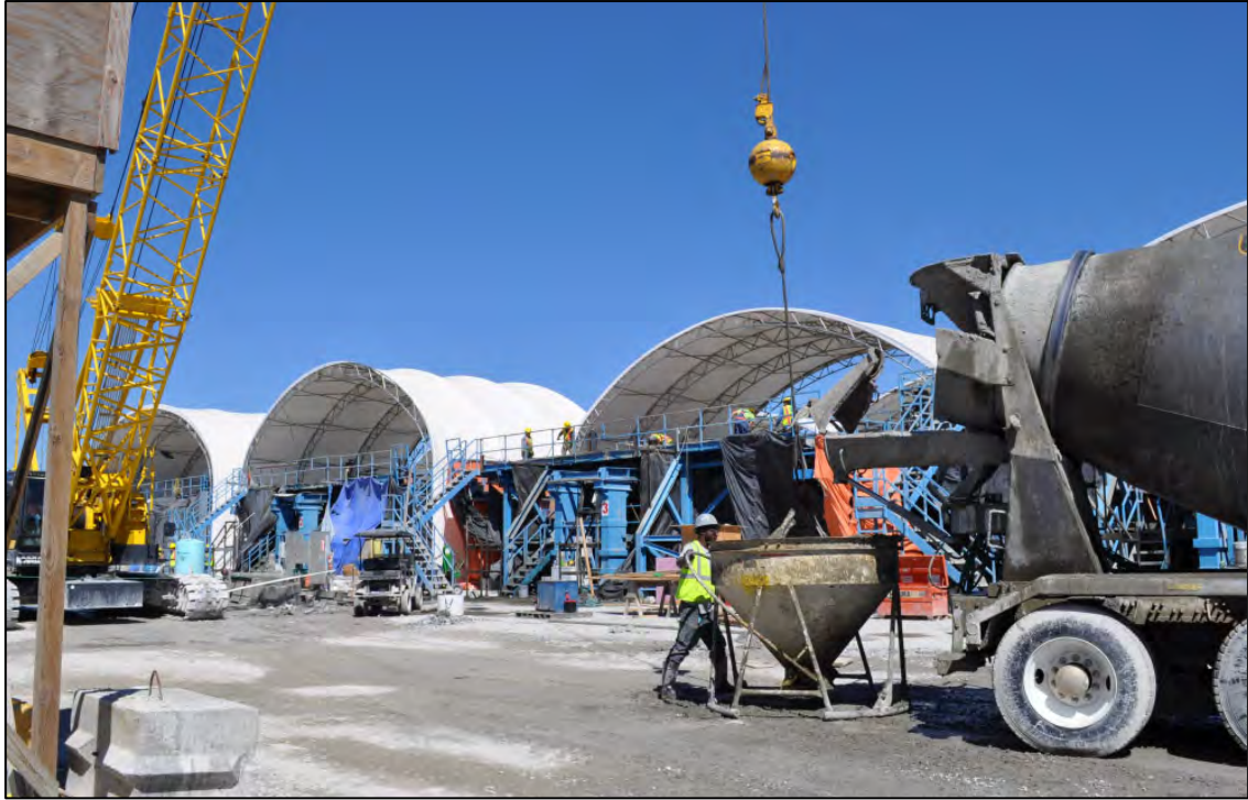
Figure 5-9: Concrete bucket being filled by ready-mixed concrete truck
