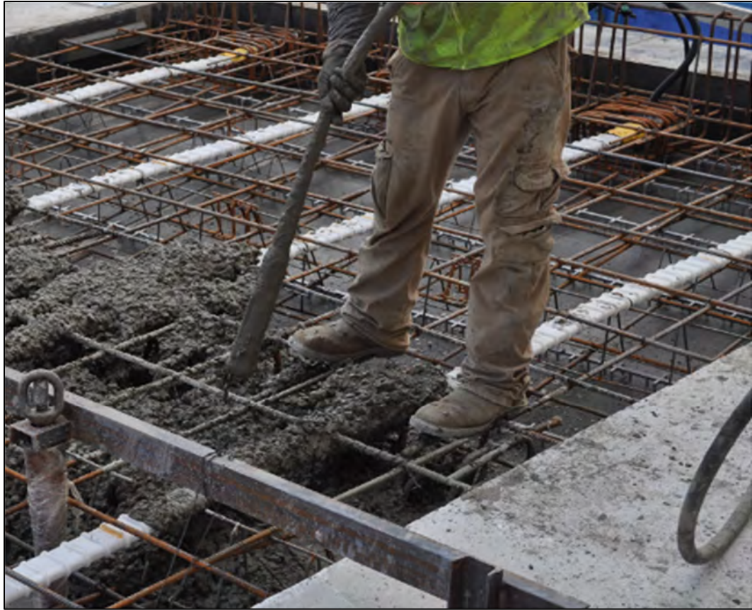
Figure 5-11: Consolidation using a portable vibrator
