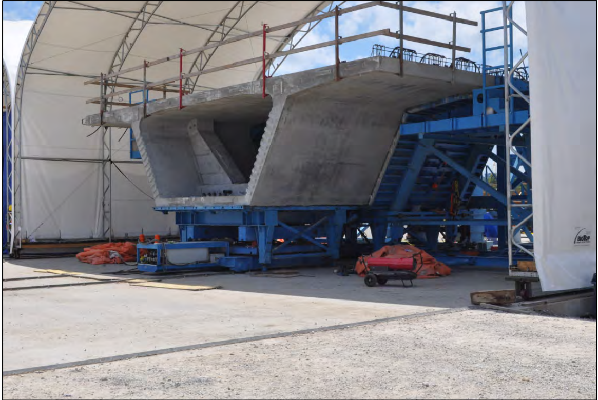
Figure 5-13: Roll-away canopy to protect each form from severe weather
