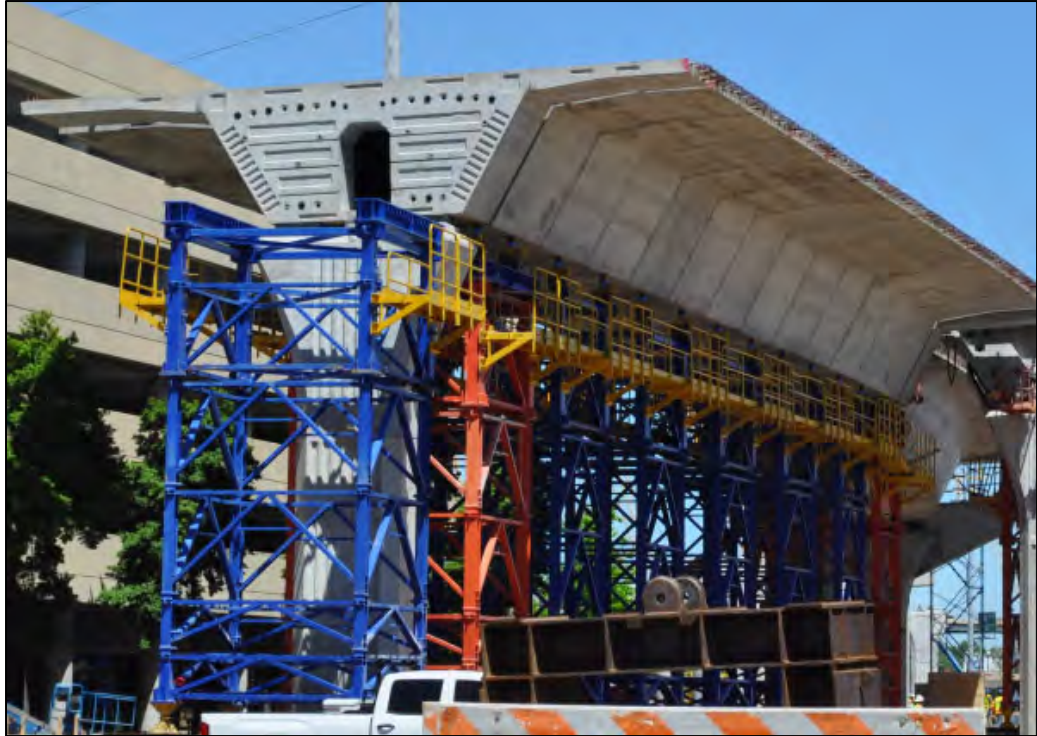
Figure 1-2: Birmingham I-59/I-20 segmental bridge during construction
