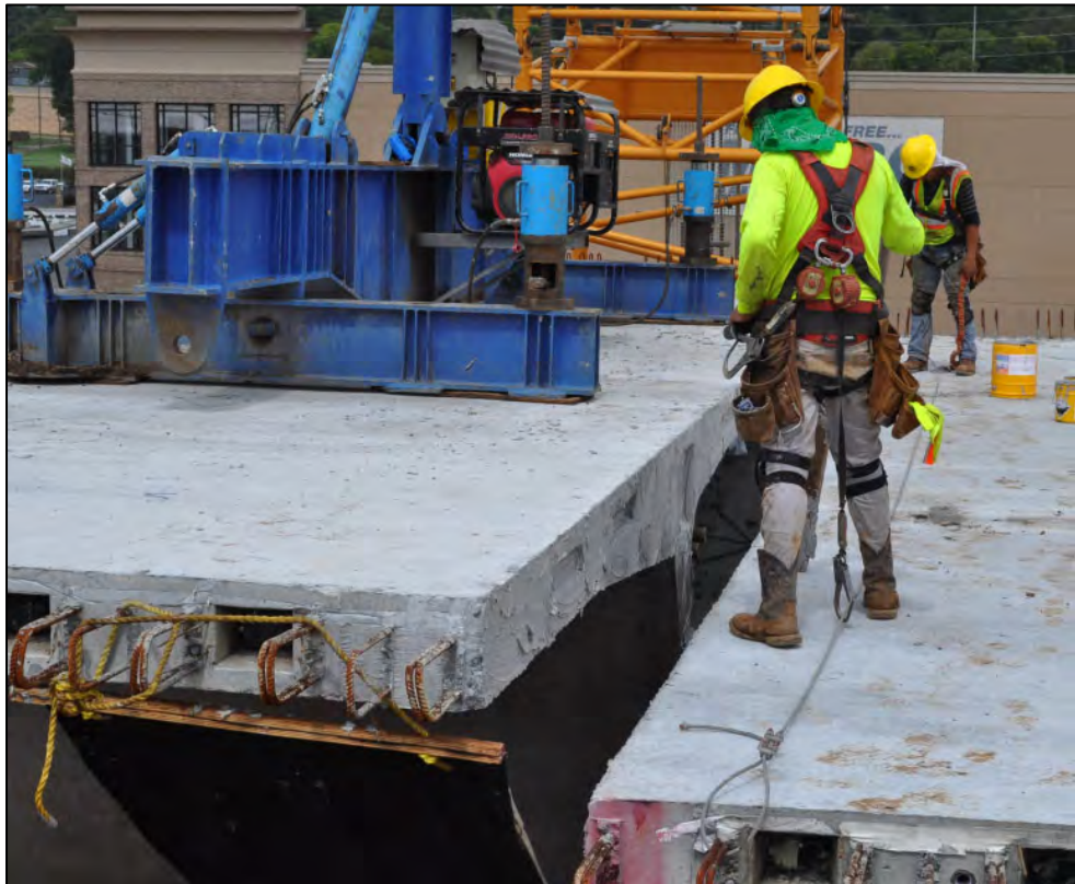
Figure 5-17: Segment being guided into place on falsework
