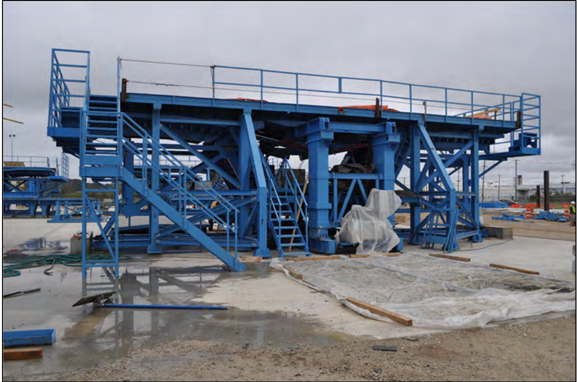
Figure 5-2: Formwork used to cast segments
