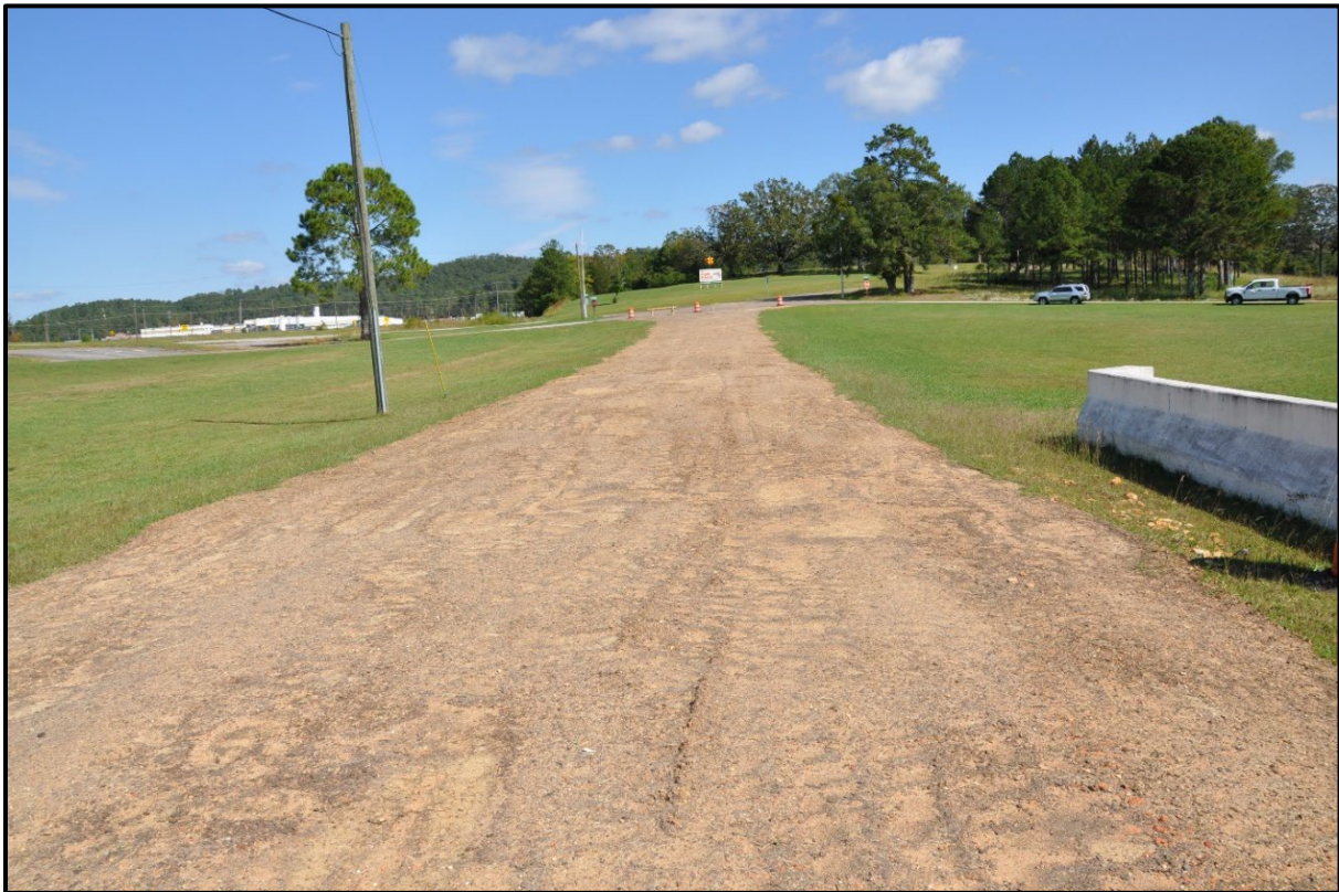
Figure 4.9. BIN 20432 road surface.
