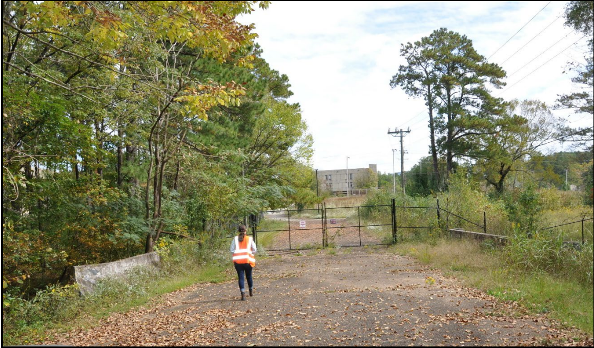
Figure 4.17. BIN 20442 and fence.
