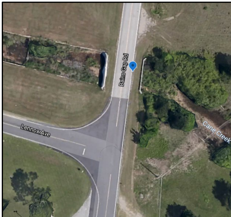
Figure 5.4. BIN 20433 Bain's Gap Road culvert aerial photo (Google Earth).
