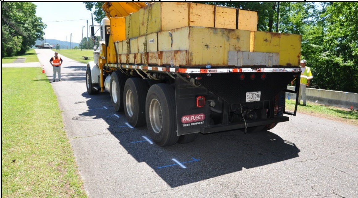
Figure 5.33. Load truck in crown stopping point (load line 2) at Berman Road culvert.
