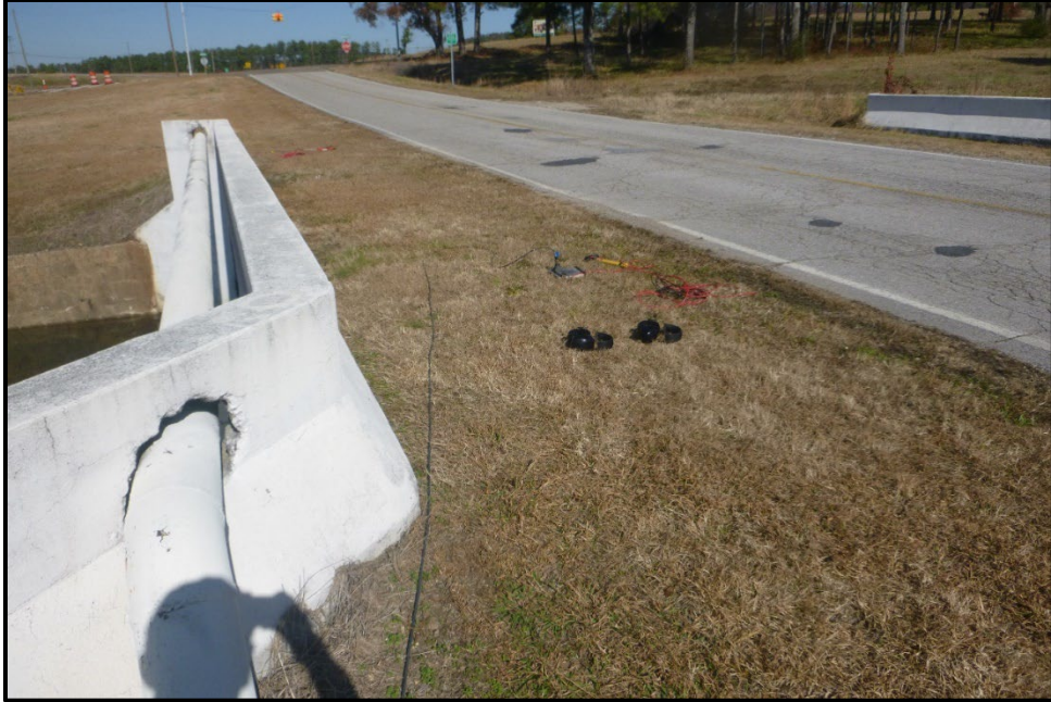
Figure 4.22. Seismic wave testing at Lennox Avenue.
