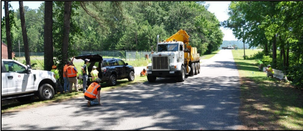
Figure 5.34. Load truck in reverse pass at Berman Road culvert.
