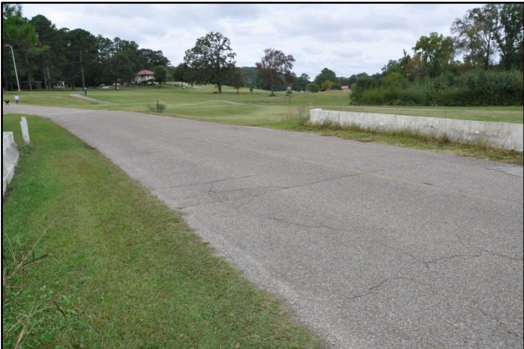
Figure 4.8. BIN 20431 road surface.
