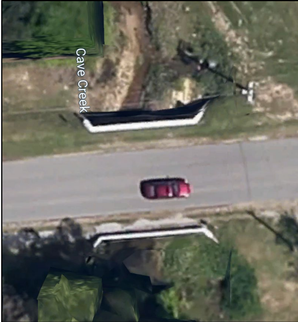
Figure 4.5. BIN 18615 (Google Earth).
