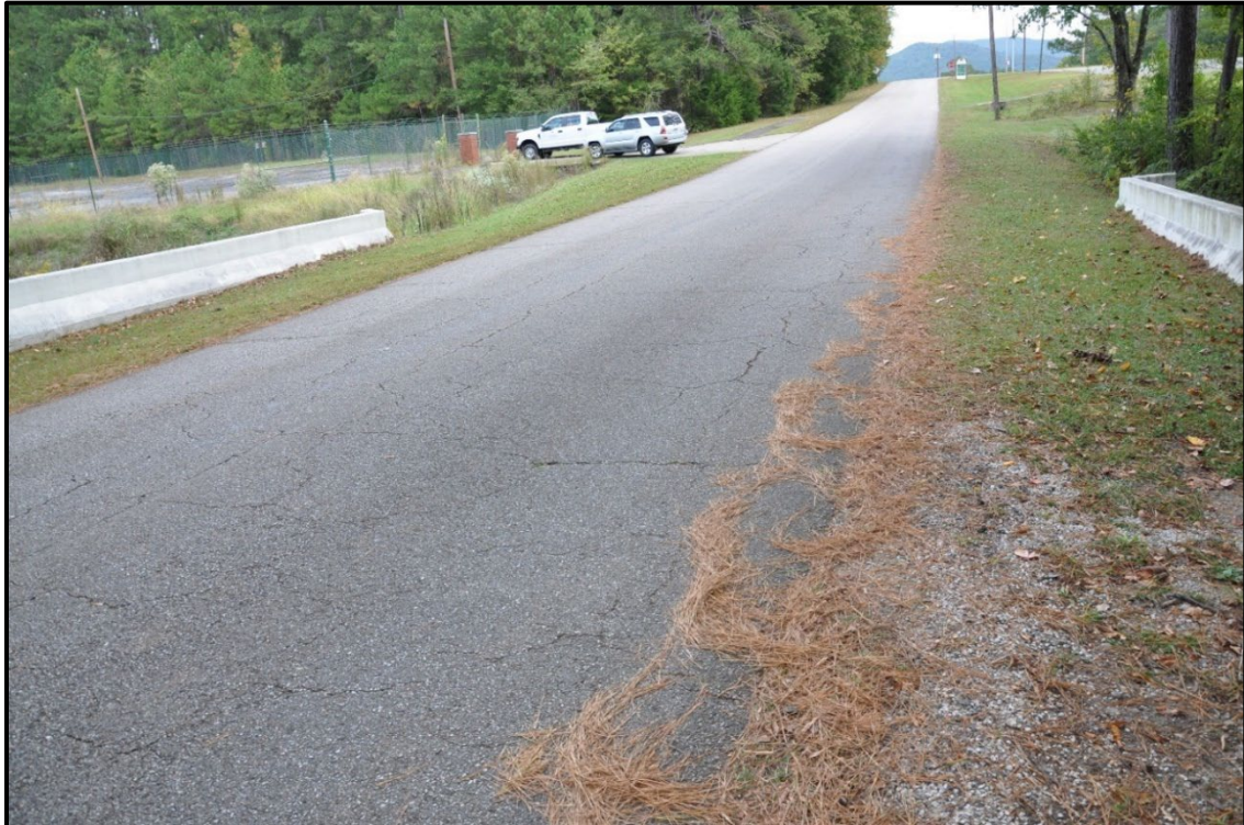
Figure 4.15. BIN 20441 road surface.
