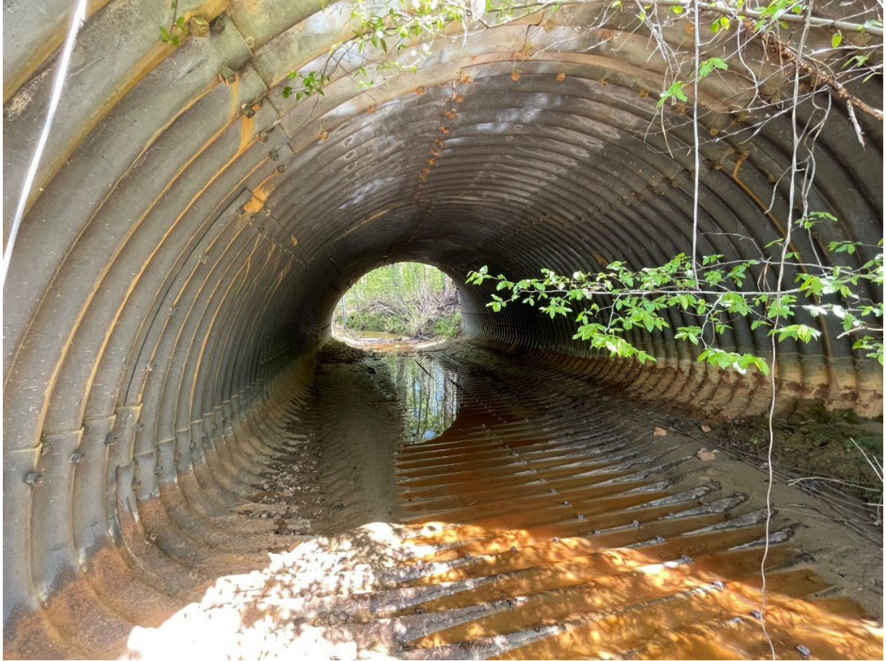
Figure 4.4. BIN 18609 from site visit.
