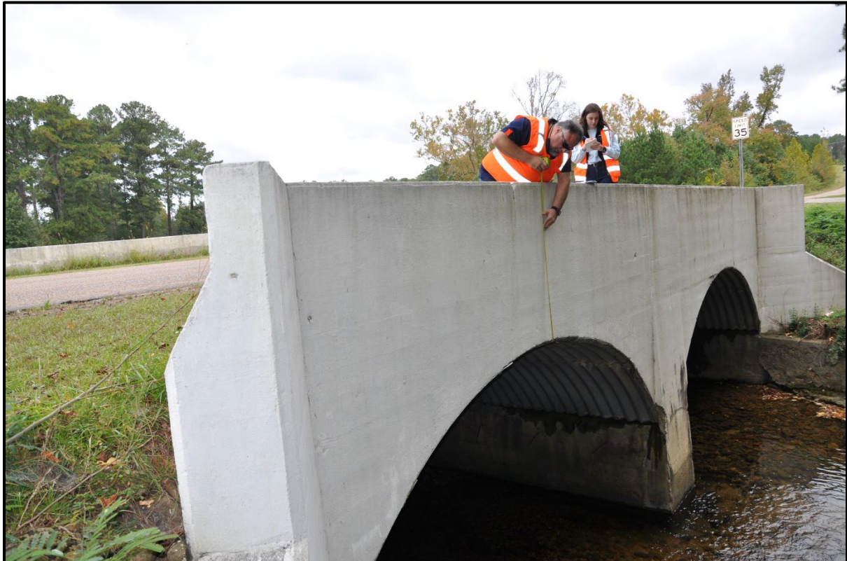
Figure 4.25. October 16, 2020 site visit.
