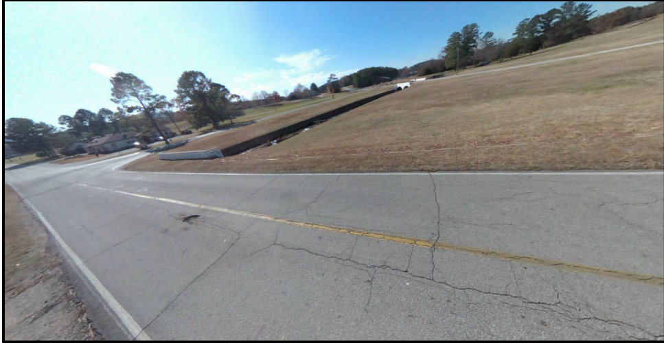
Figure 4.20. Seismic tests at Lennox Avenue.
