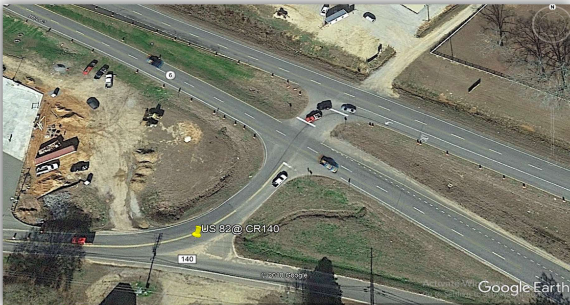
Figure 19. US 82 at County Road 140 Before Condition (Google Earth)
