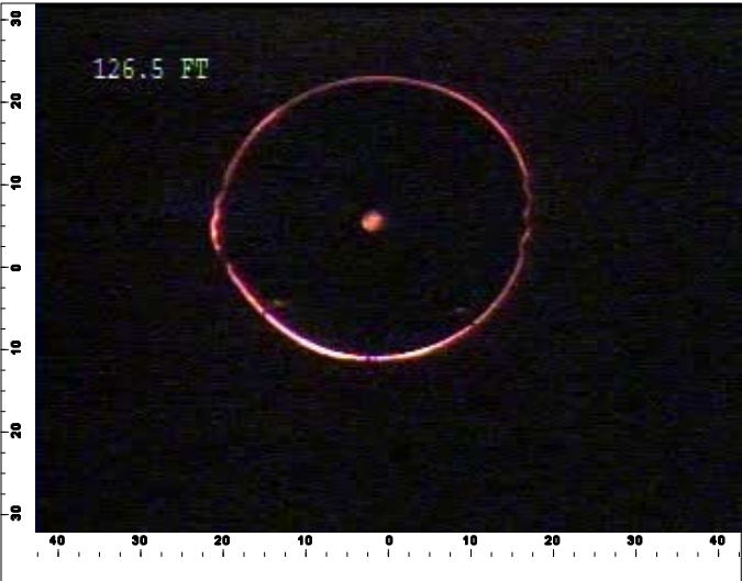
Racking- pipe losing its stability
