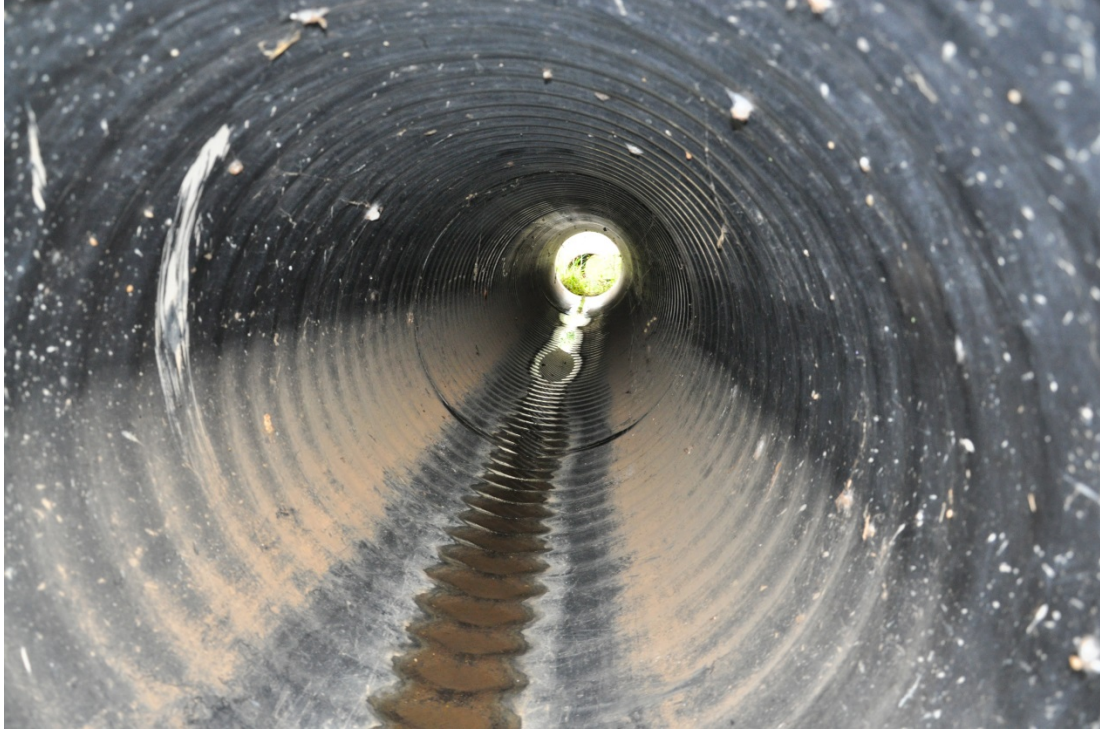
Figure 3-16: Internal Conditions of Center Pipeline
