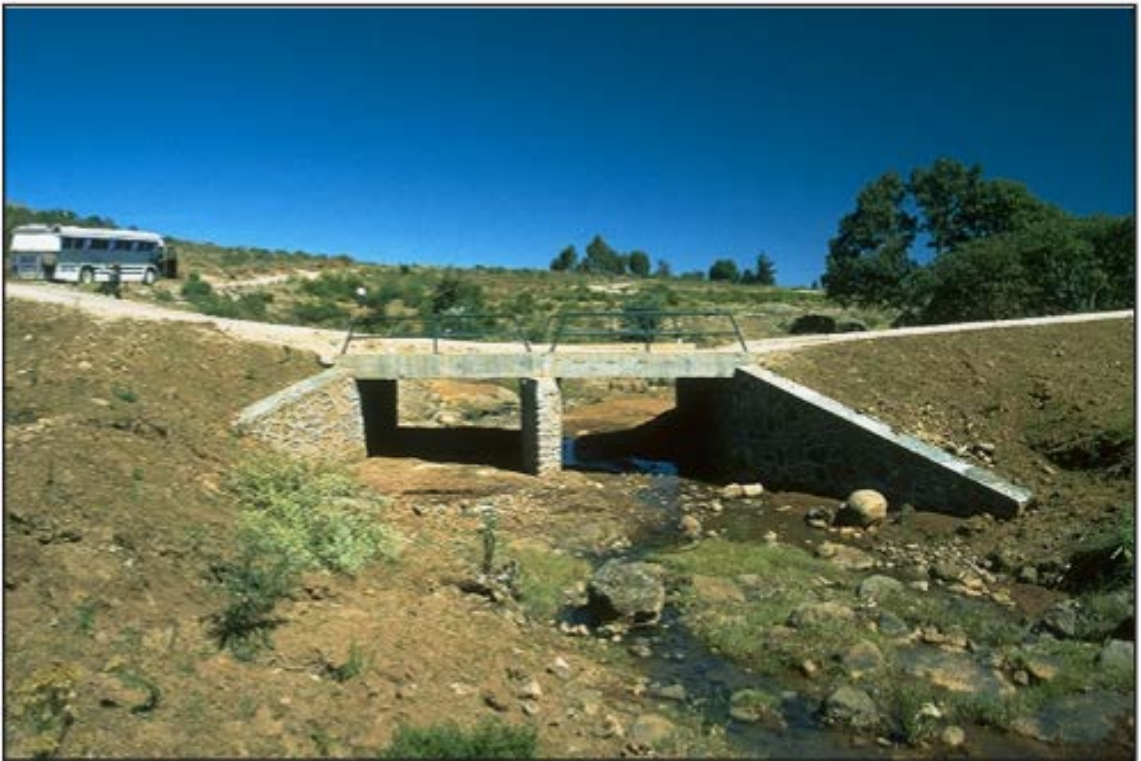
Figure 5-45: Reinforced Concrete Box Culvert (Keller 2003)
