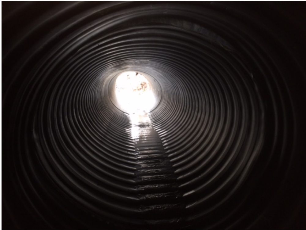
Figure 3-8: Large Deflections Occurring in Pipe B
