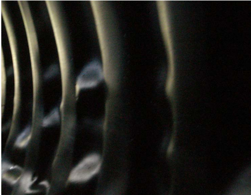
Figure 3-5: Rippling Discovered along Pipe Sidewalls
