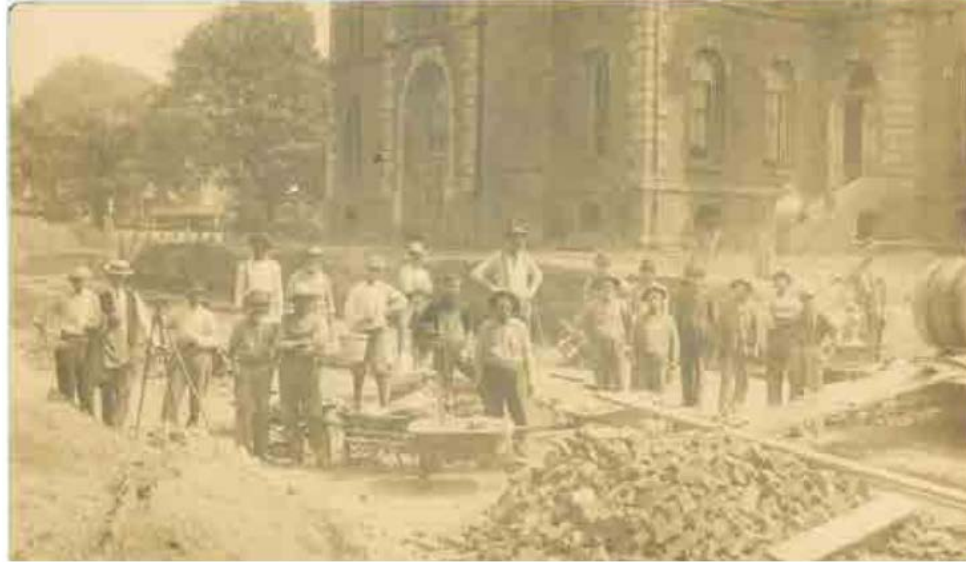
Figure 5-3: Installation of Corrugated Metal Culvert (Baldwin 2014)
