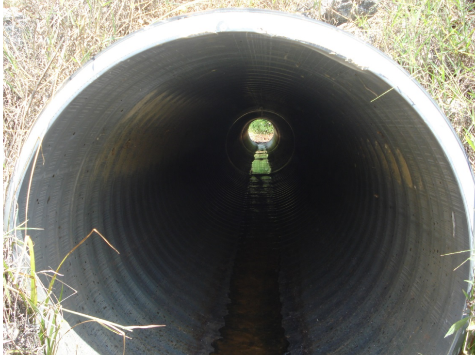
Figure 3-20: Internal Inspection of Wetumpka Pipeline
