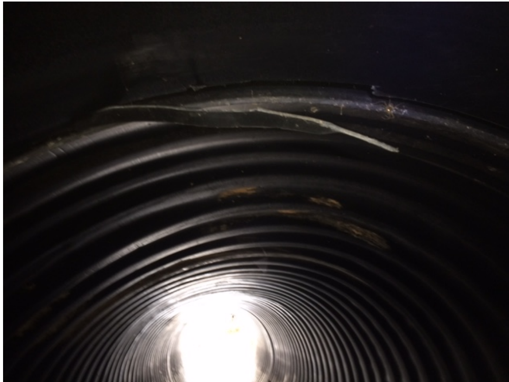
Figure 3-11: Tear in the Pipe End at a Joint Location within Pipe A
