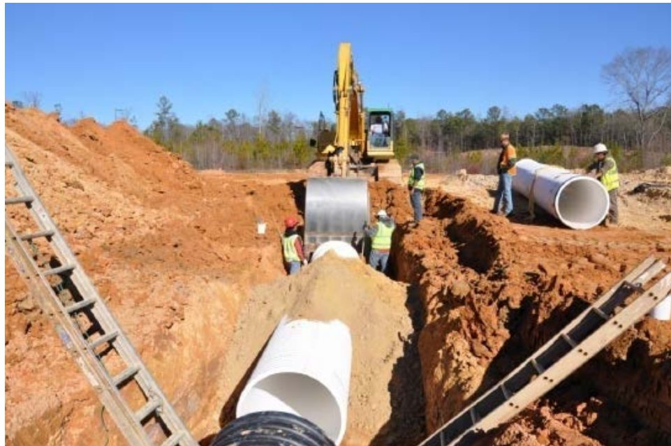
Figure 4-7: Backfill Placed to Secure PVC Pipe Segments (Stuart et al. 2011)
