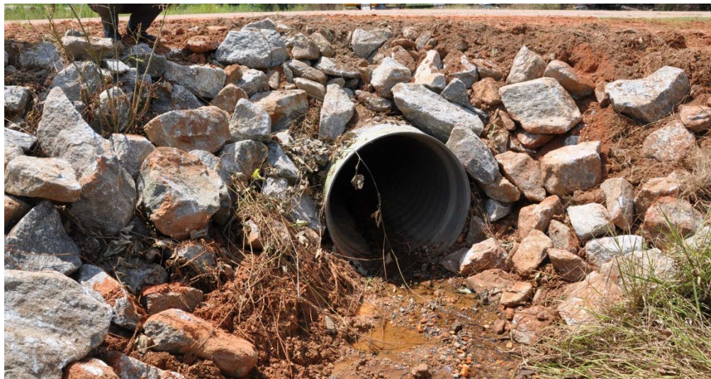
Figure 3-18: 36-inch Diameter Pipe underneath County Service Road
