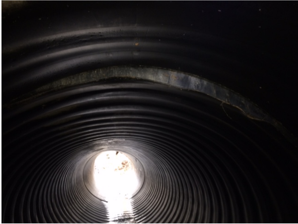
Figure 3-12: Joint Separation
