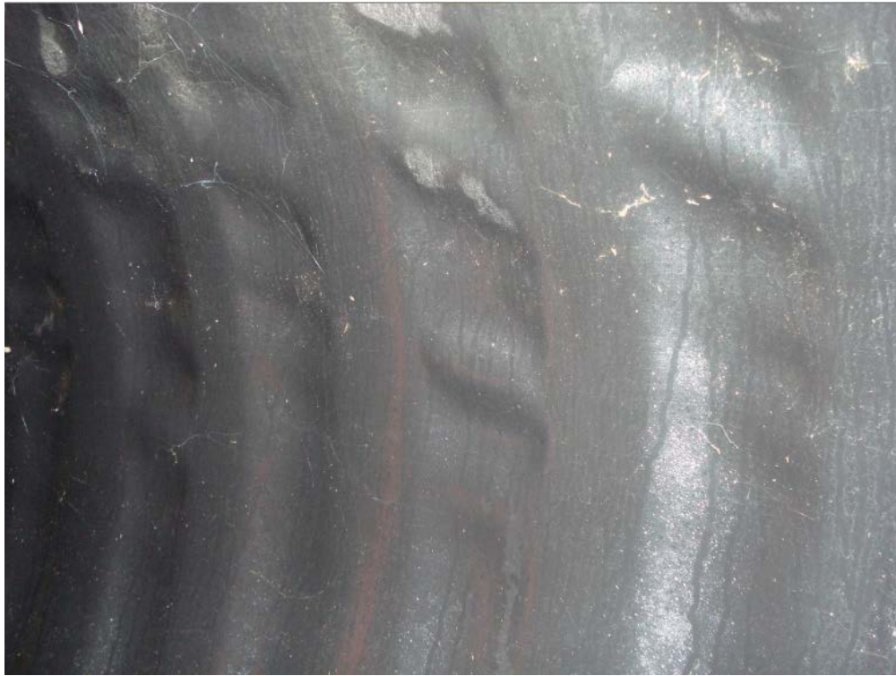
Figure 3-6: Rippling Damage in the Pipes Sidewall
