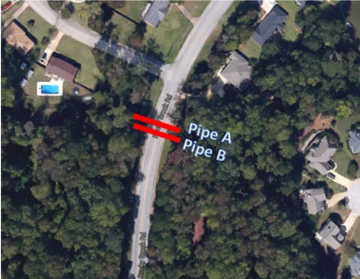
Figure 3-2: Overhead View of the Opelika Pipe Location (Google Maps)
