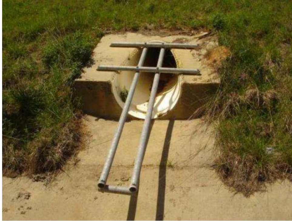
Figure 4-16: Entry Protection Installed at Pipe Ends
