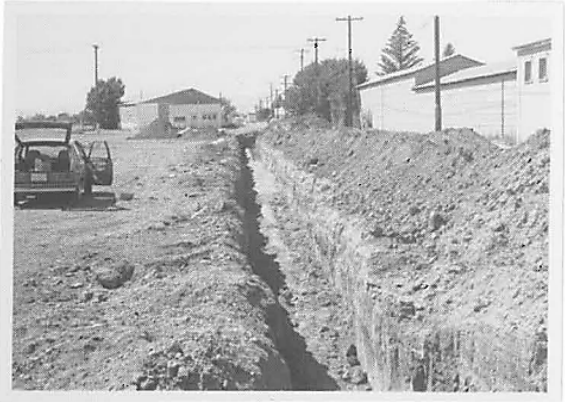
Figure 5-50: 21-inch Polyvinyl Chloride Sewer Pipe after Backfill (Woodham 1988)
