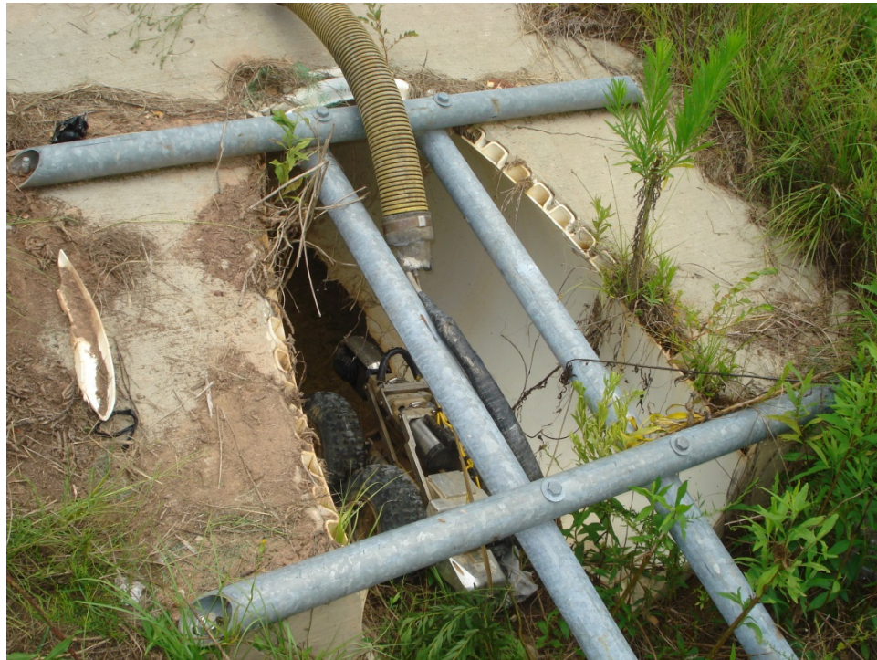
Figure 4-54: Laser Robot Entering PVC Pipe
