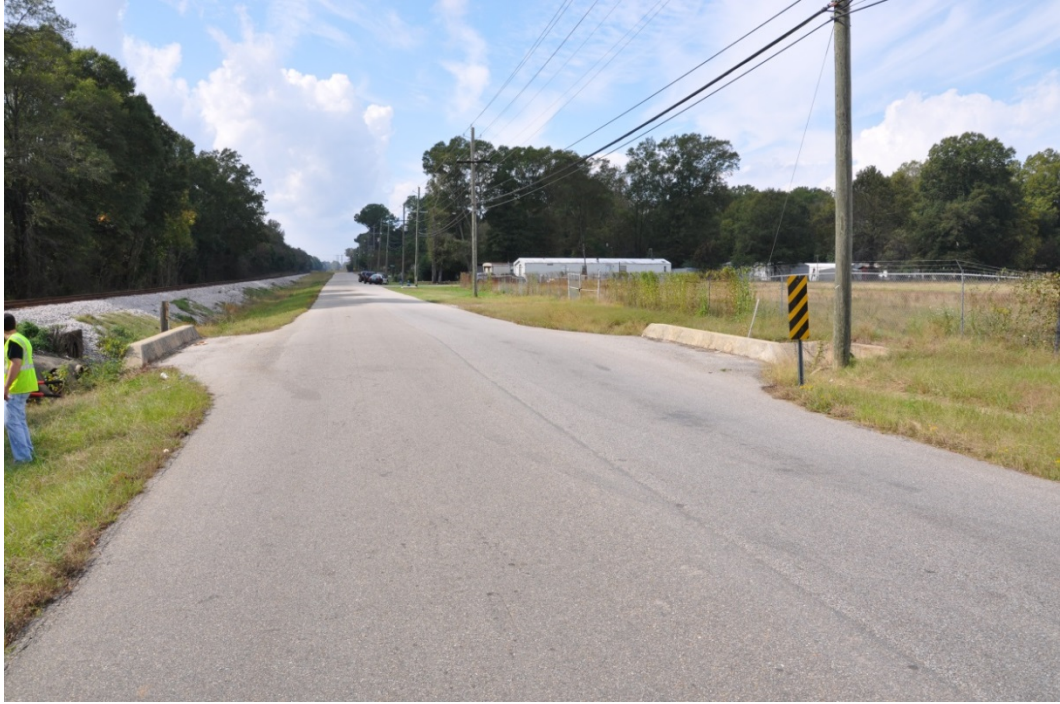
Figure 3-15: Two Lane Road Traveling over Montgomery Site
