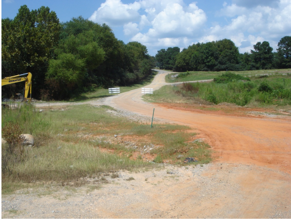
Figure 3-19: Service Road chosen for Pipe Installation
