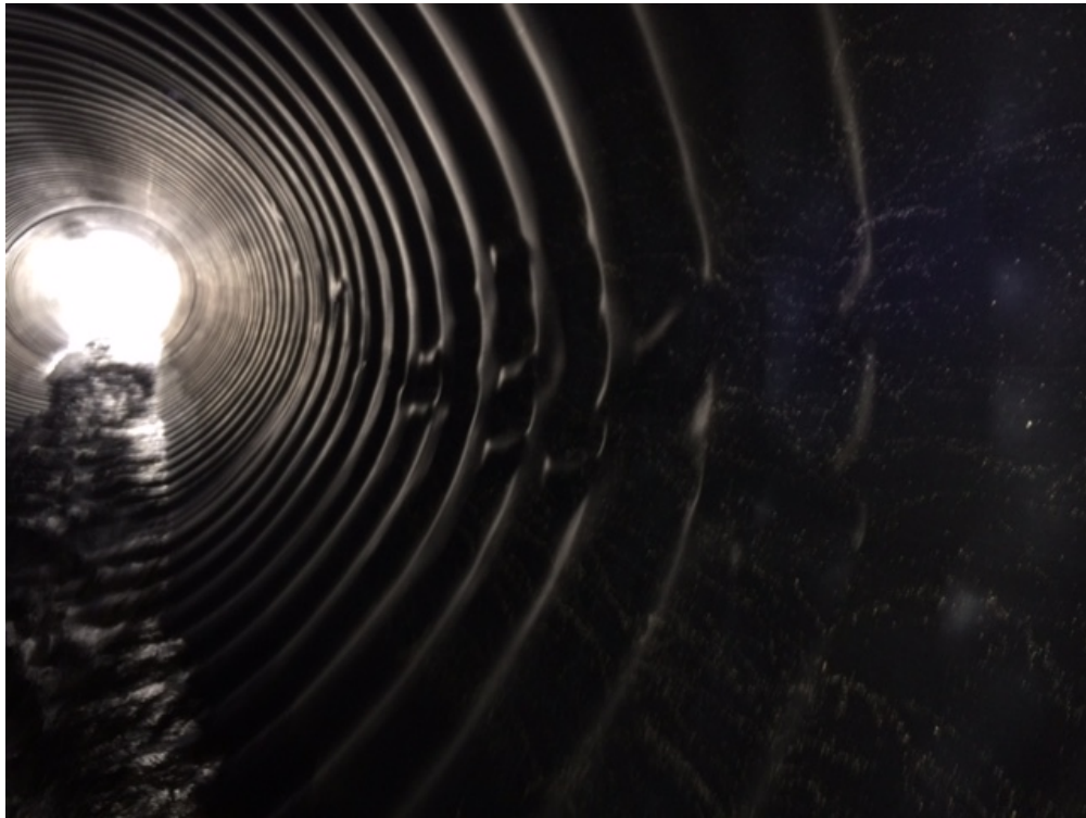
Figure 3-13: Continued Rippling throughout the Length of both Pipes
