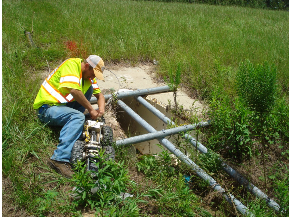
Figure 4-53: Preparing Laser Robot for Pipe Inspection
