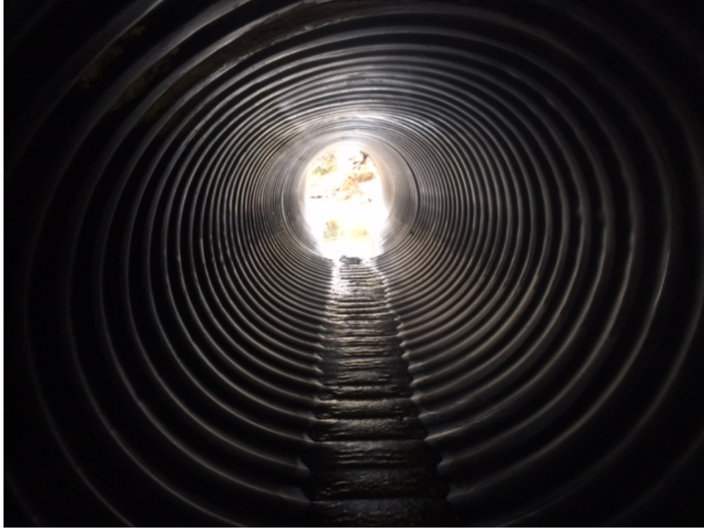
Figure 3-7: Increased Deflections Occurring within Pipe A
