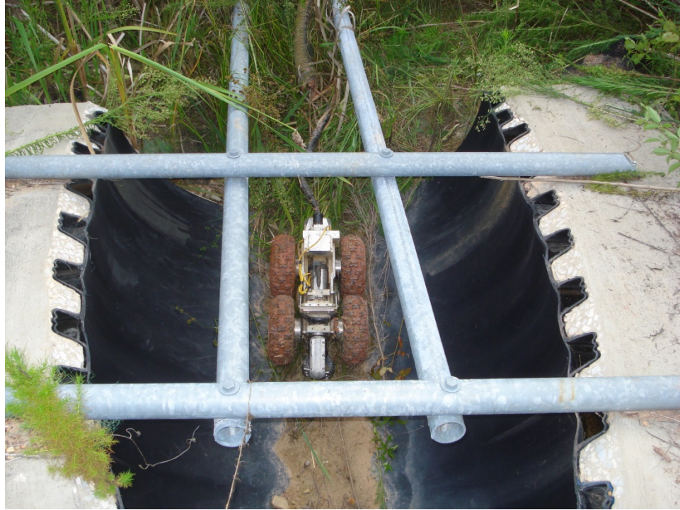
Figure 4-55: Top View of Laser Robot Entering HDPE Pipe
