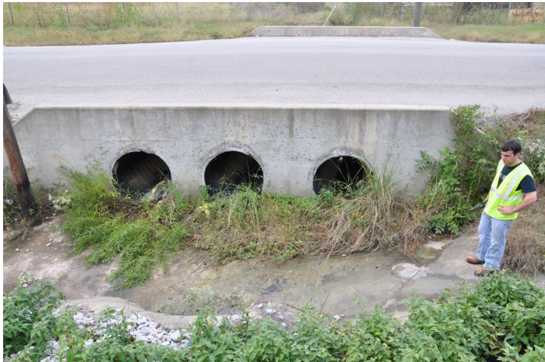
Figure 3-14: Three 36-inch HDPE Pipes in Montgomery
