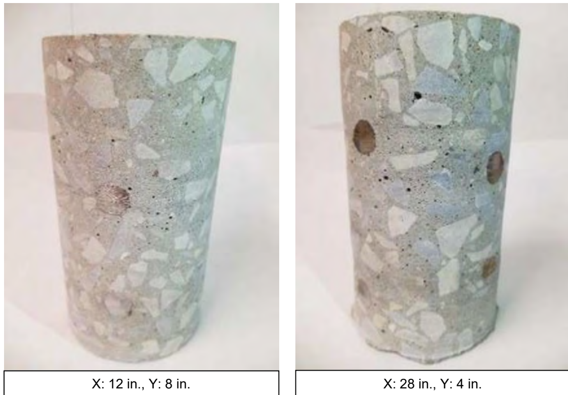
Figure 4-32: Poor Delamination Simulation using Sand Layer in Specimen DL3
