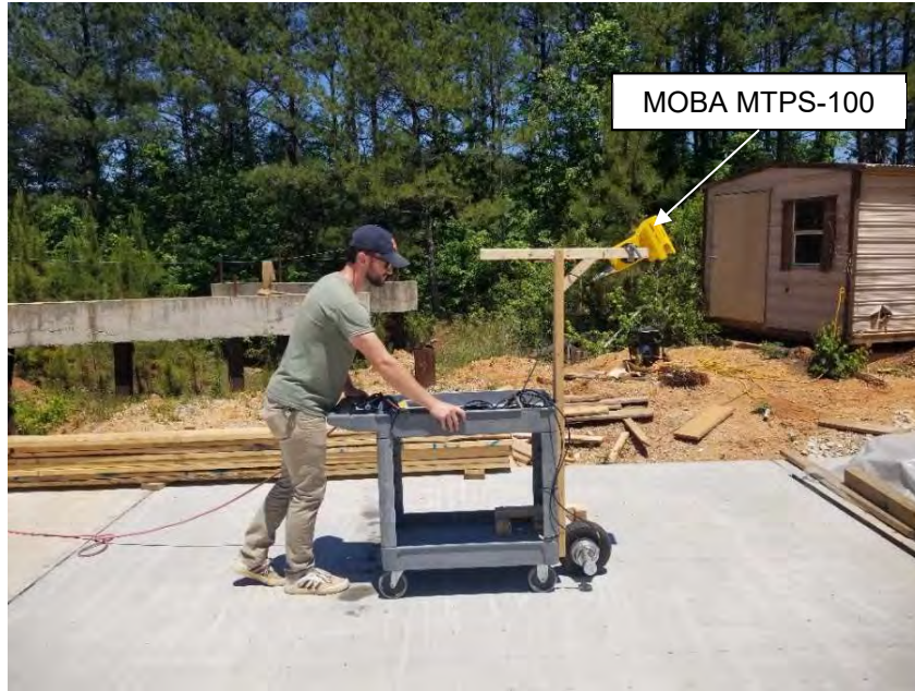
Figure 5-12: IRT Evaluation of Bridge Deck using the MOBA MTPS-100 Cart System
