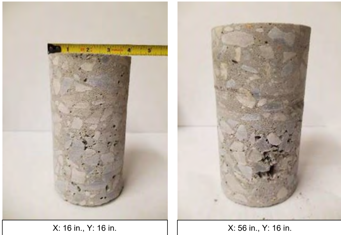
Figure 4-40: Honeycombing in Miniature Slab Concrete of Specimen DE3
