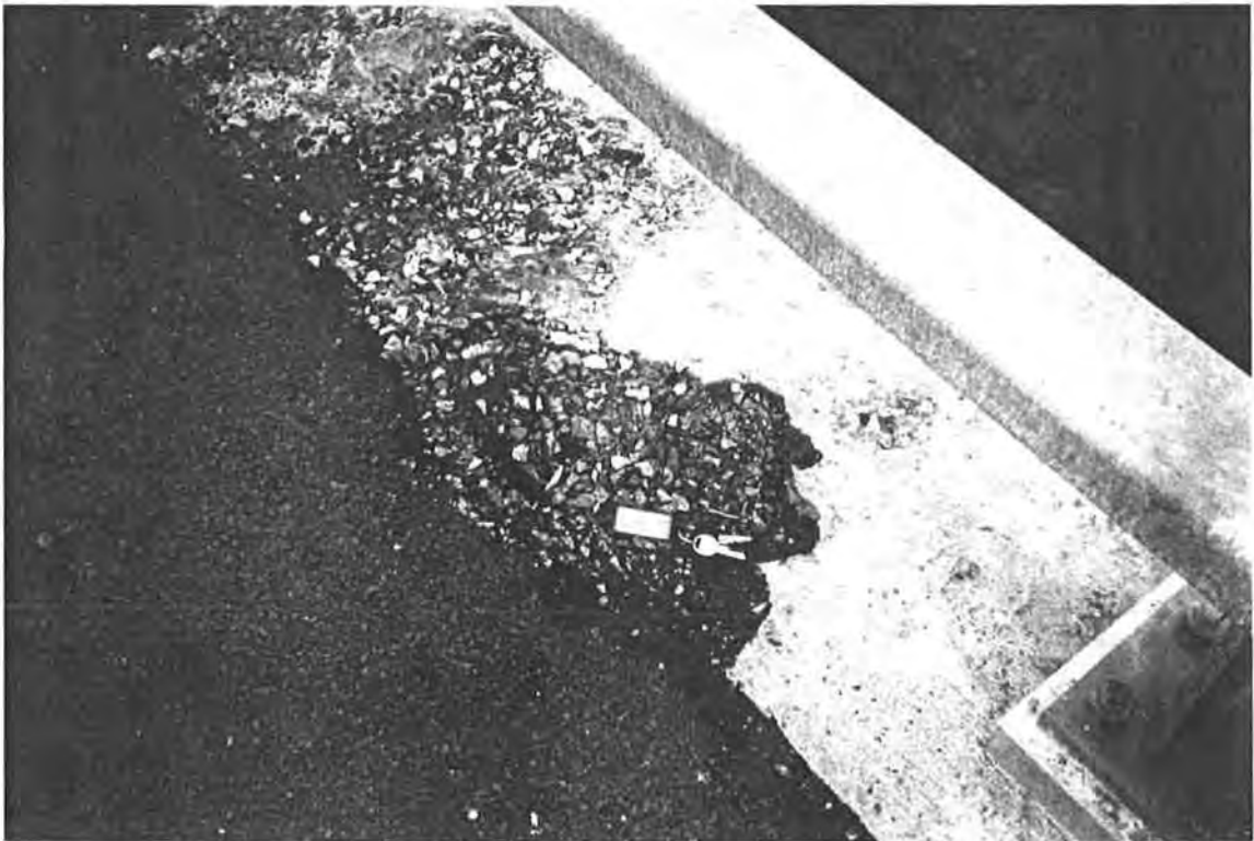
Figure 4.60. Additional Spalling Along Curb
