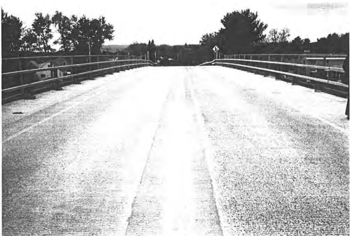
Figure 4.39. Dunnsville Bridge with Replacement Deck of SCC
