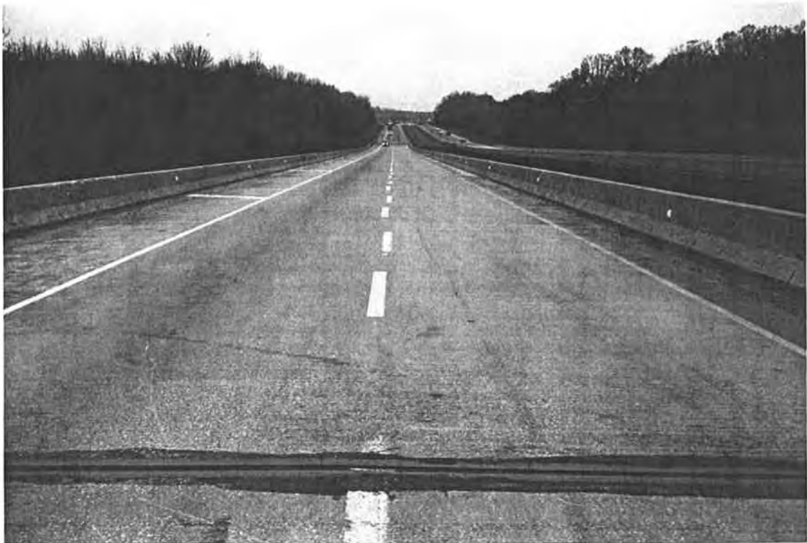
Figure 4.29. Eleven Year Old SCC Bridge Deck
