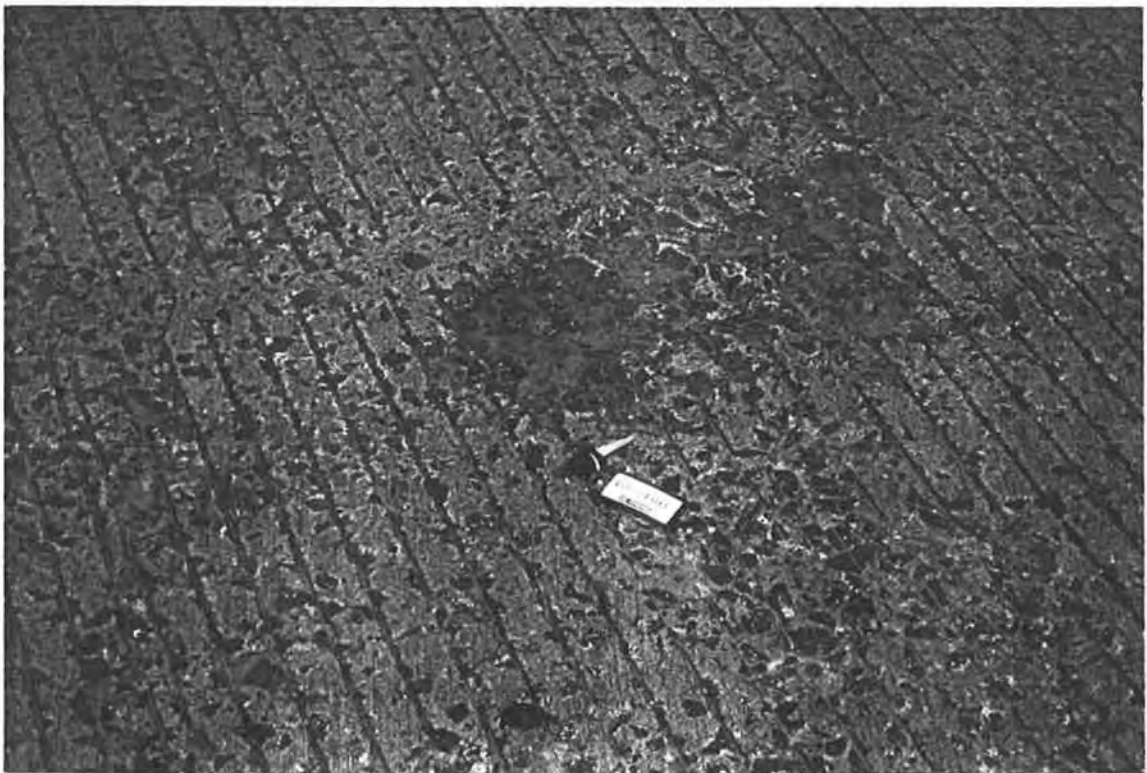
Figure 4.50. Close-Up of Surface Spalling in Wheel Path
