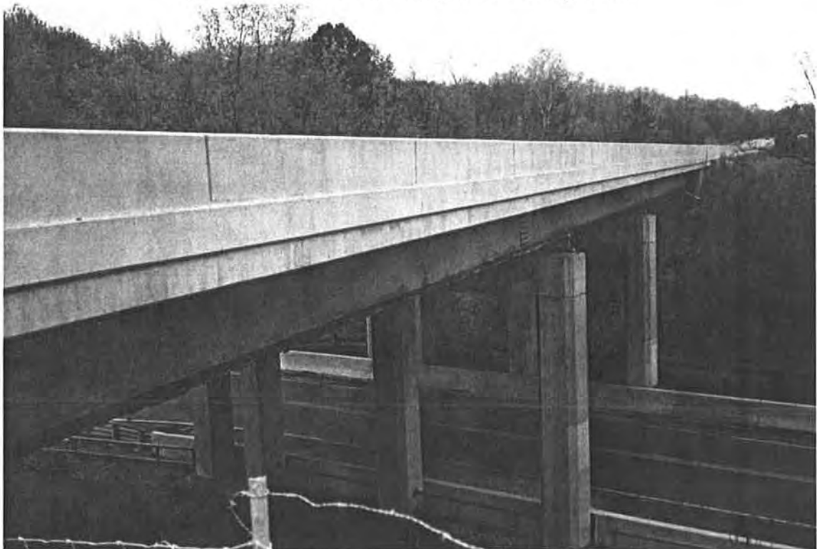
Figure 4.24. Typical Ohio Turnpike Continuous Steel Girder Bridge
