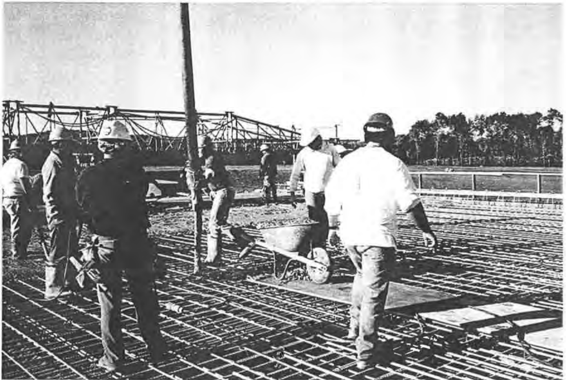
Figure 4.15. Concrete Sampling at End of Pump Line
