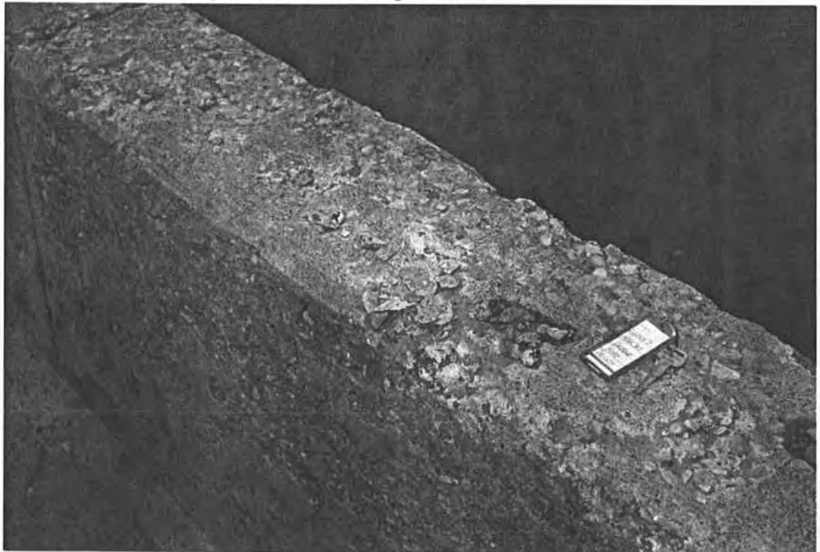
Figure 4.34. Close-Up of Guardrail Scaling
