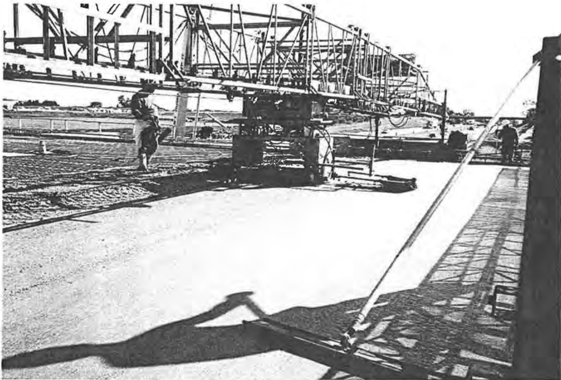
Figure 4.12. Close-Up of Roller Screeding and Bull Floating
