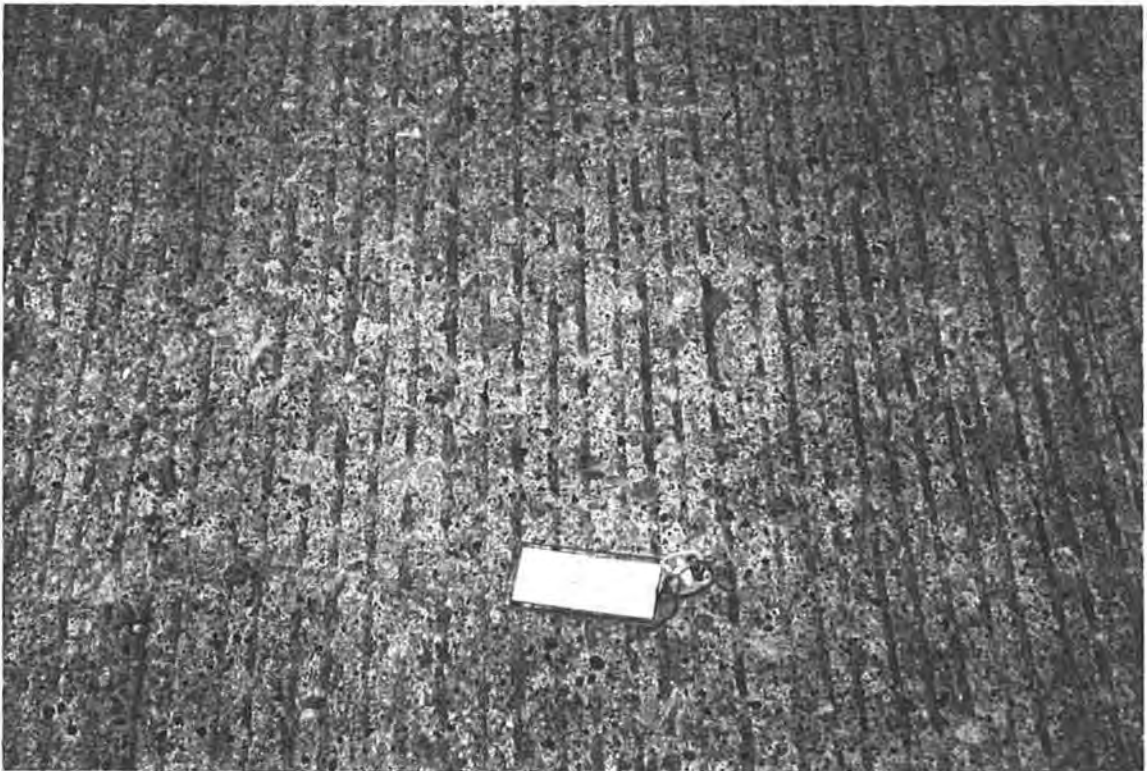
Figure 4.32. Close-Up of Traffic Wear
