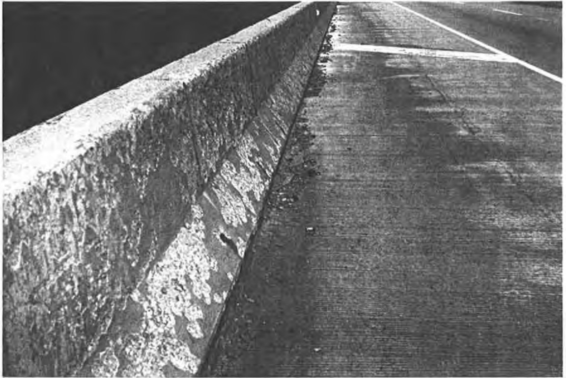
Figure 4.33. Bad Scaling of SCC Guardrail
