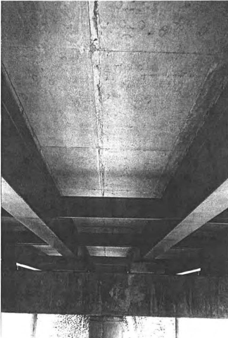
Figure 4.65. Mint Condition of Underside of Bridge/Deck
