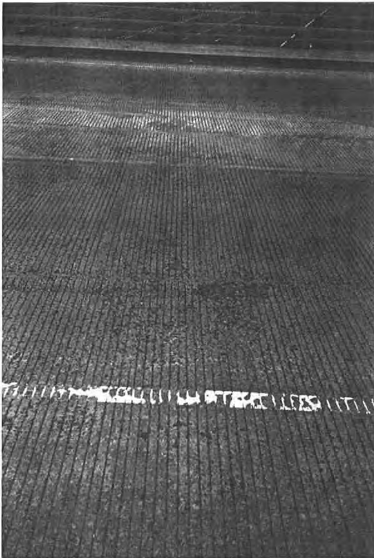
Figure 4.49. Surface Spalling in Wheel Path
