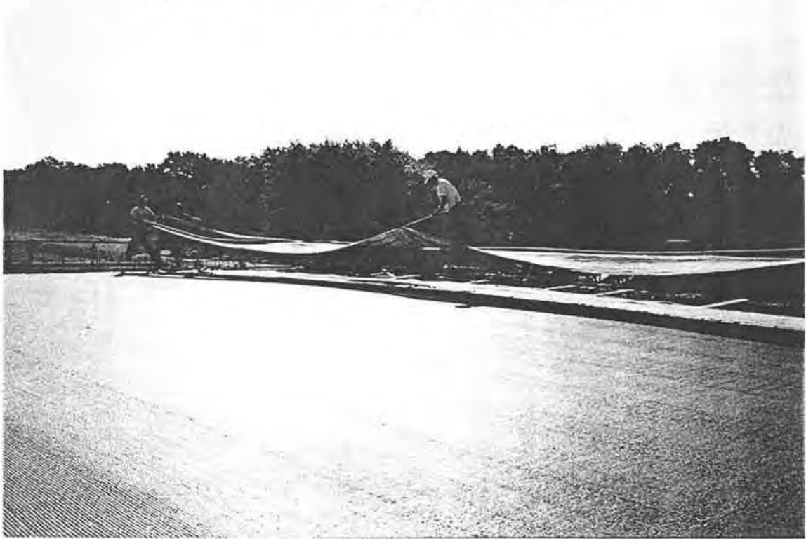
Figure 4.21. Placing Wet Burlap for Curing
