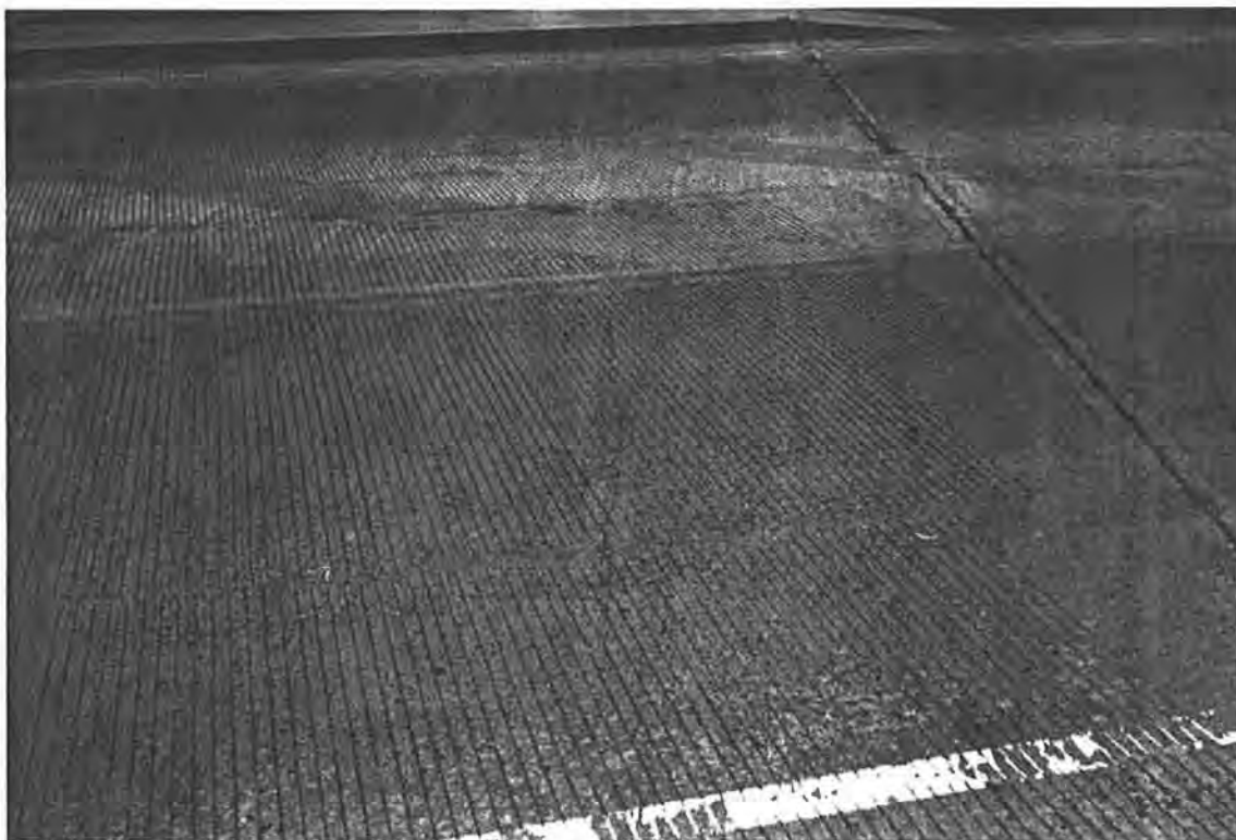
Figure 4.47. Transverse Crack Near Abutment Joint
