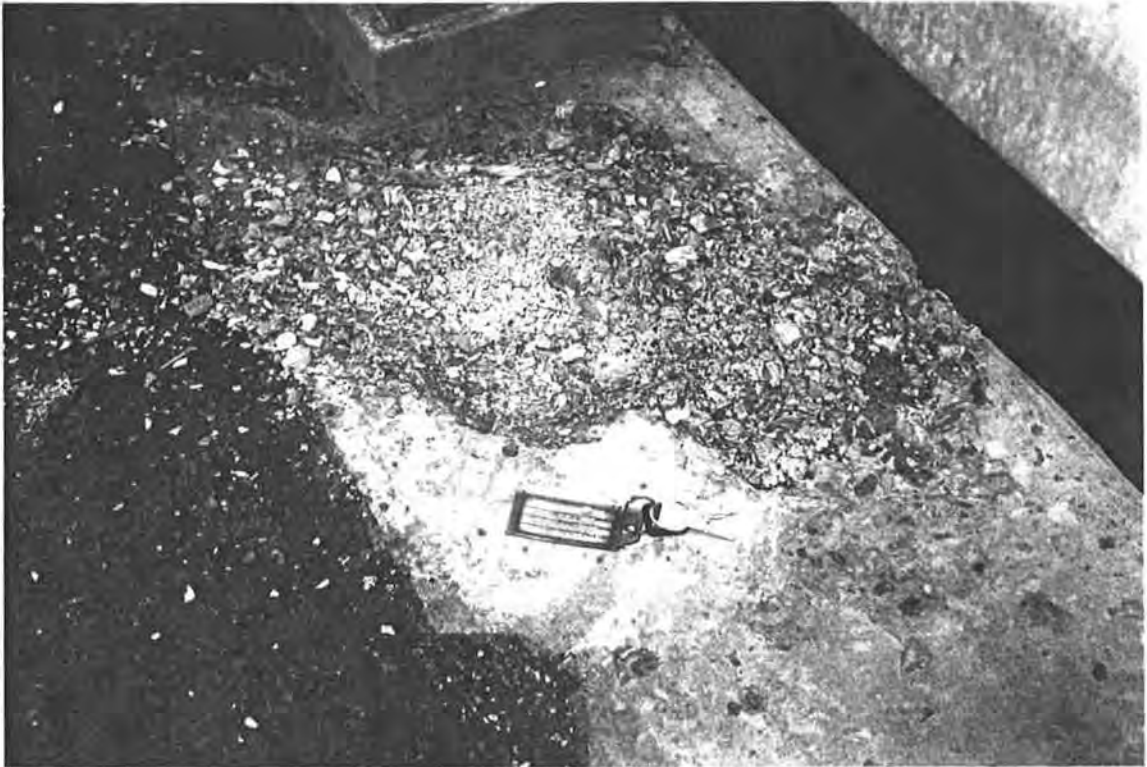
Figure 4.59. Severe Spalling Along Curb
