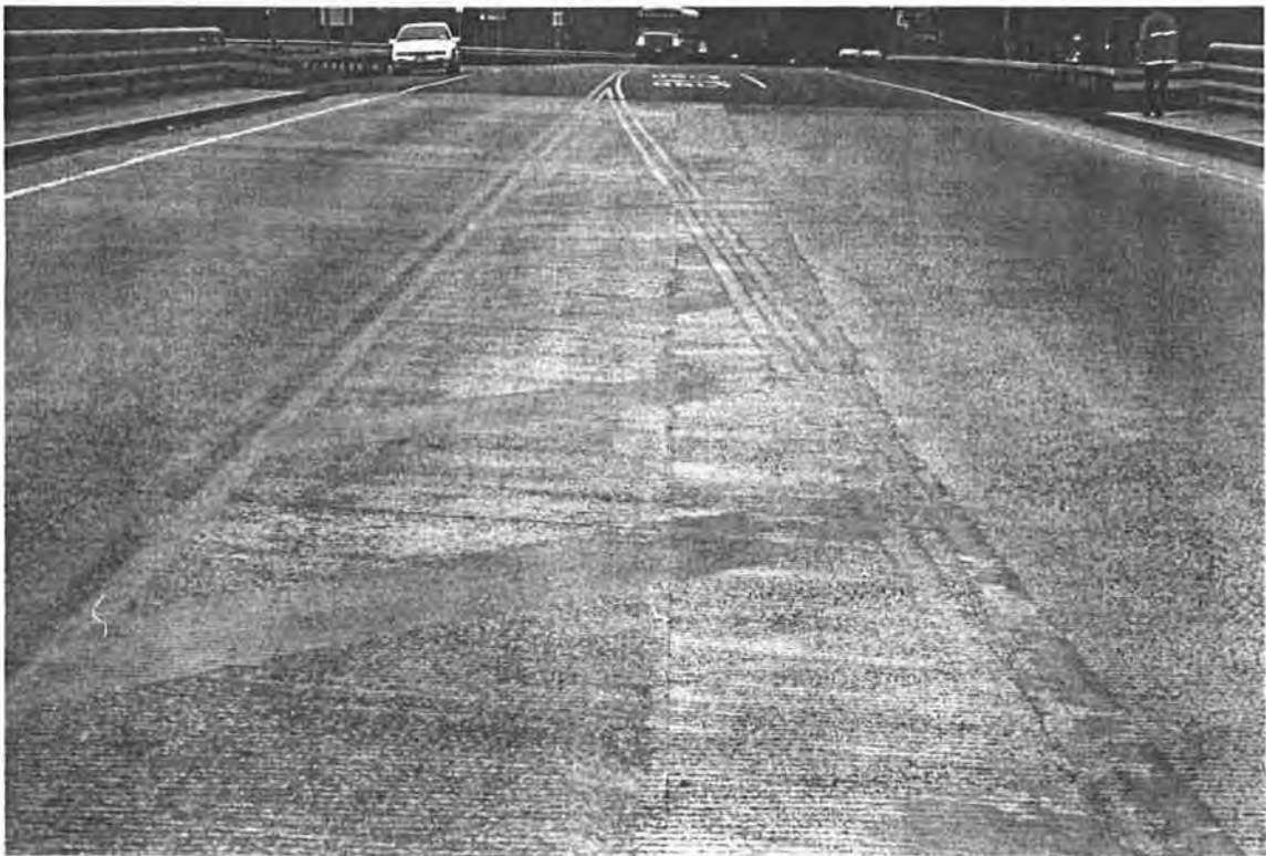
Figure 4.46. SCC Deck Showing Center Closure Concrete
