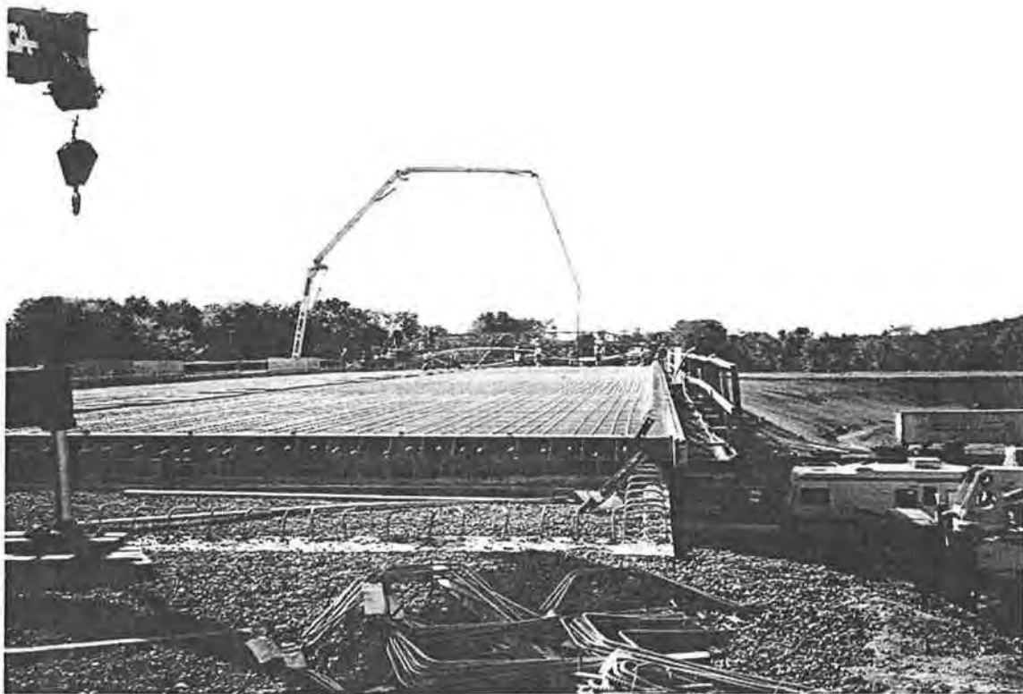
Figure 4.4. Entire Bridge Deck Ready for Concrete Placement Via Pumping
