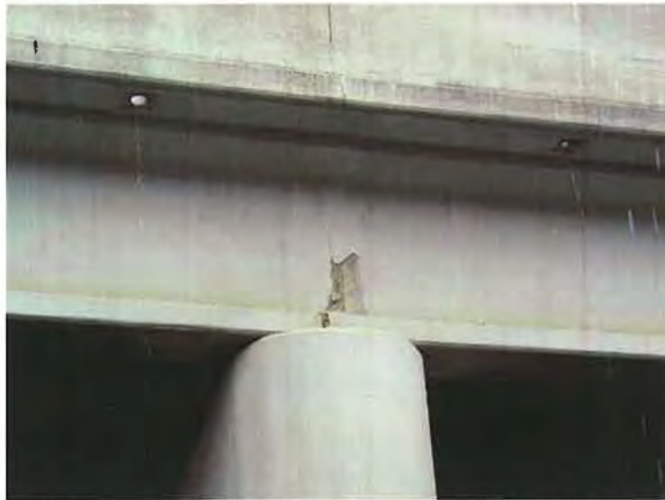
Figure 3.3 – Typical End Crack in a Continuity Diaphragm
