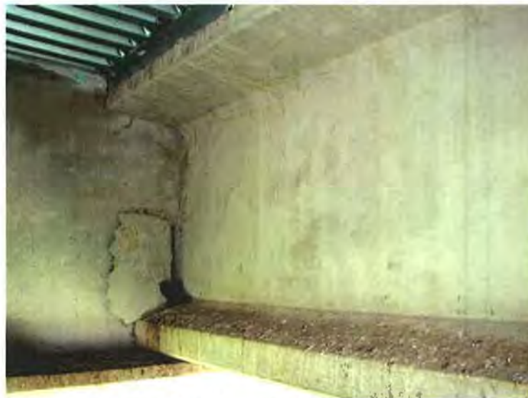
Figure 3.2 – Typical Pull-out Failure of a Prestressed Concrete Bulb-tee Girder
