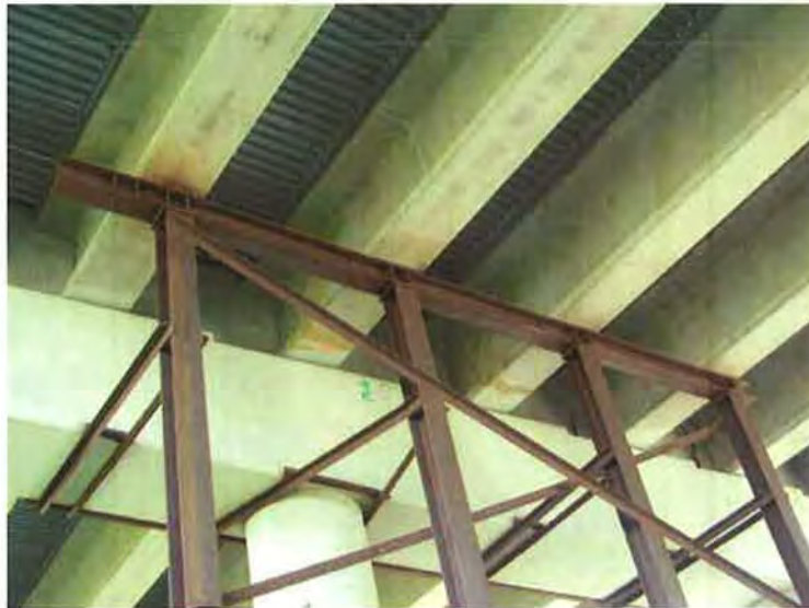
Figure 3.4 – Typical False Support
