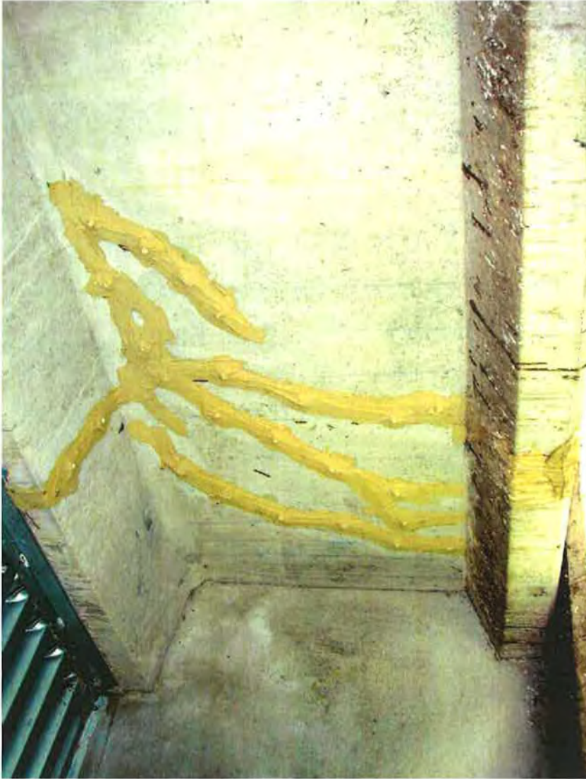
Figure 3.5 – Typical Girder with Epoxy-injected Cracks
