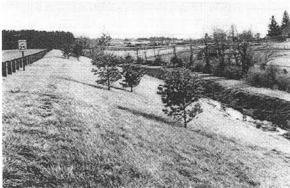
Figure 5. A construction site protected through permanent seeding (2).
