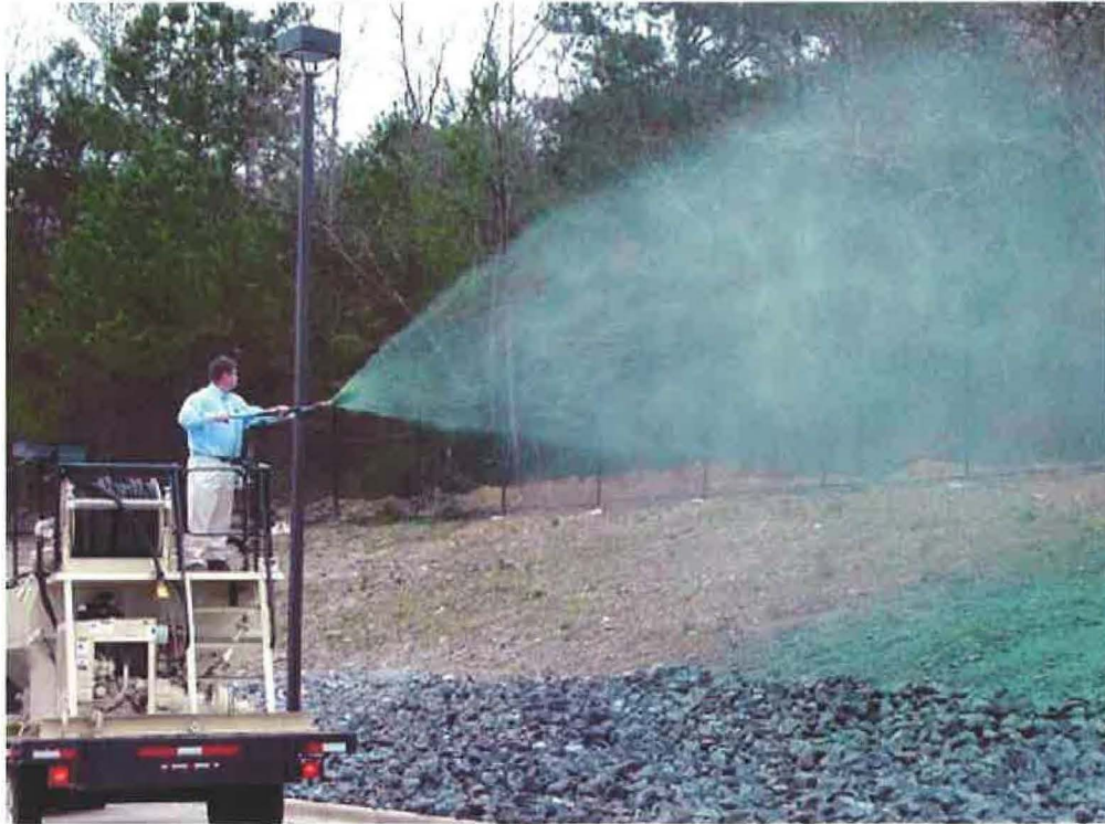
Figure 2. Applying PAM to a construction site (1).
