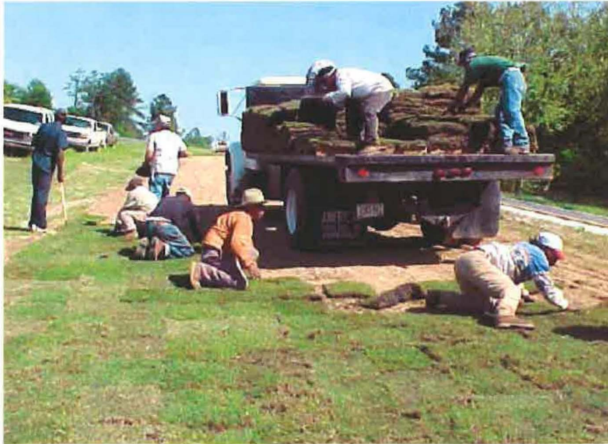
Figure 6. Sodding at a construction site (1).
