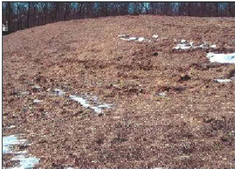
Figure 3. Mulching at a construction site (11).
