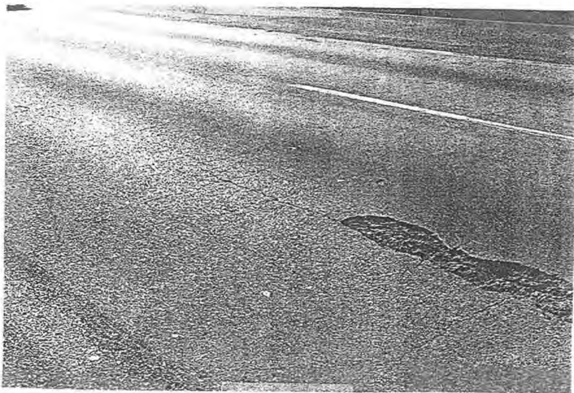
Fig. 2.2 I-65 Deck Surface Spall in Birmingham, AL (22)
