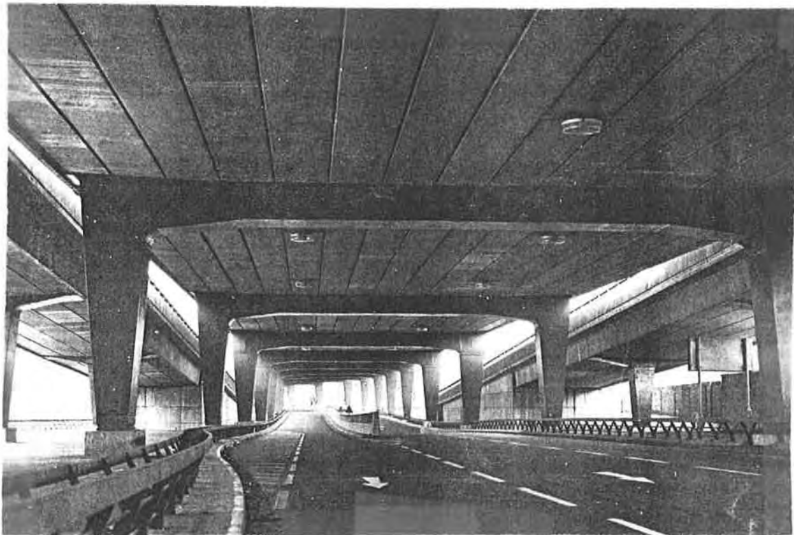
Fig. 4.2 Beam-and-Slab Deck with Contiguous Concrete Beams (16)
