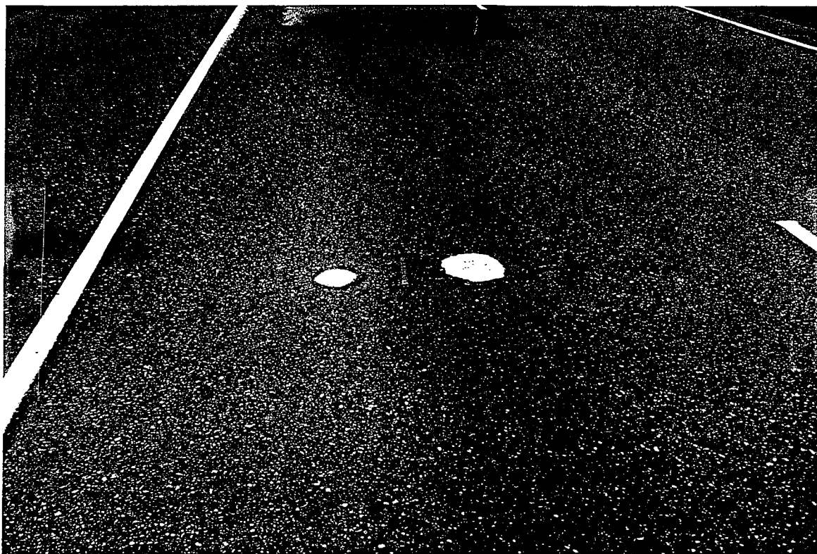
Figure 8. Typical end of load segregation at site 4.
