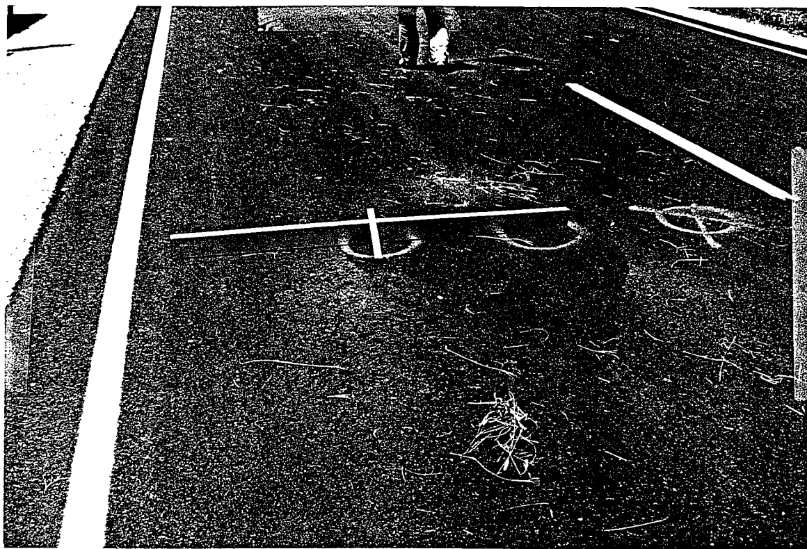
Figure 6. Pulling and tearing of mat at site 3.
