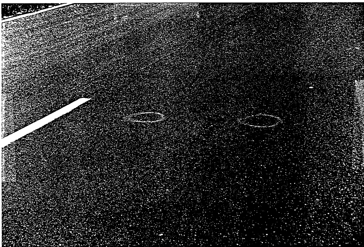
Figure 5. Segregation without raveling at site 2.
