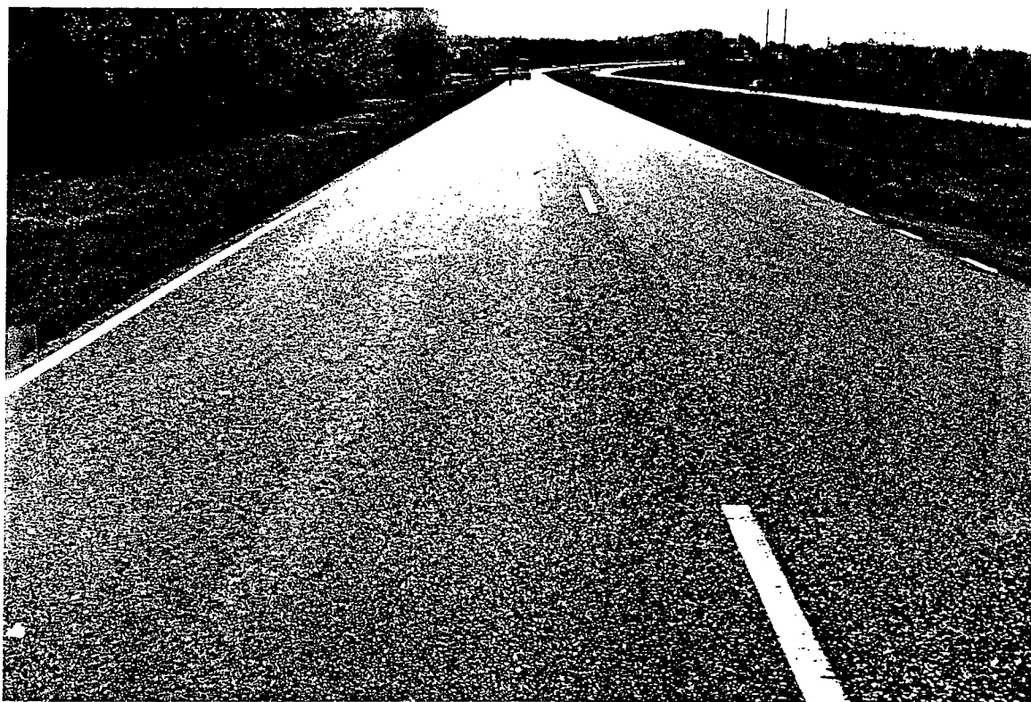
Figure 2. Typical end of load segregation at site 1.
