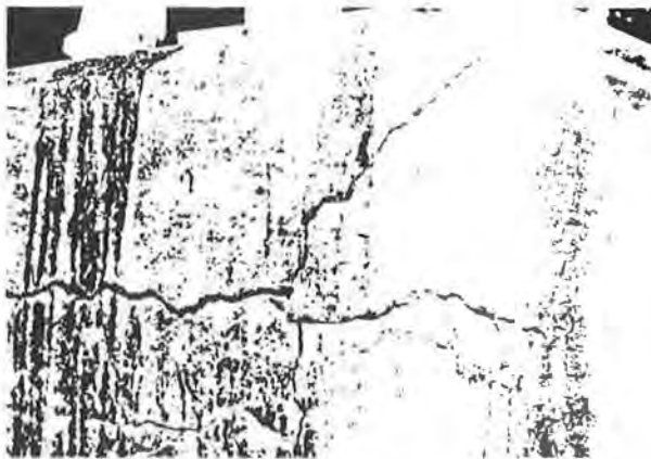
Figure 6.12 Concrete Cap with Horizontal Cracking.
