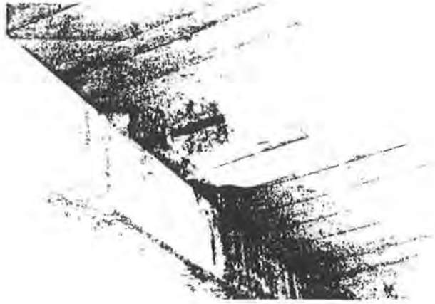
Figure 6.10 Concrete Girder with Considerable Spalling and Rebars Exposed [16].
