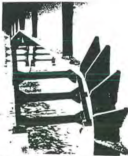
Figure 2.17 Water Trapping Stiffners.
