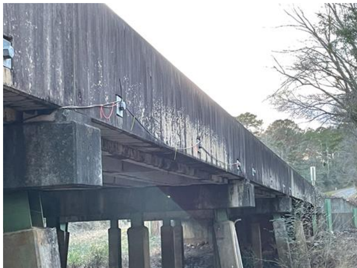
Figure 64. BIN 015002, Enterprise, AL. Sensors cables installation.
