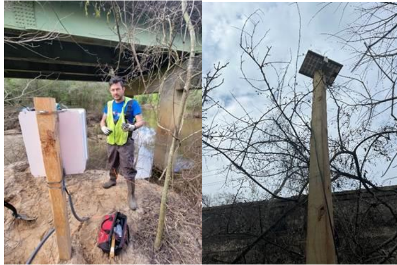
Figure 70. BIN 013310, Goshen, AL. Enclosure and Solar panel attached to a wooden post, grouted to the ground.
