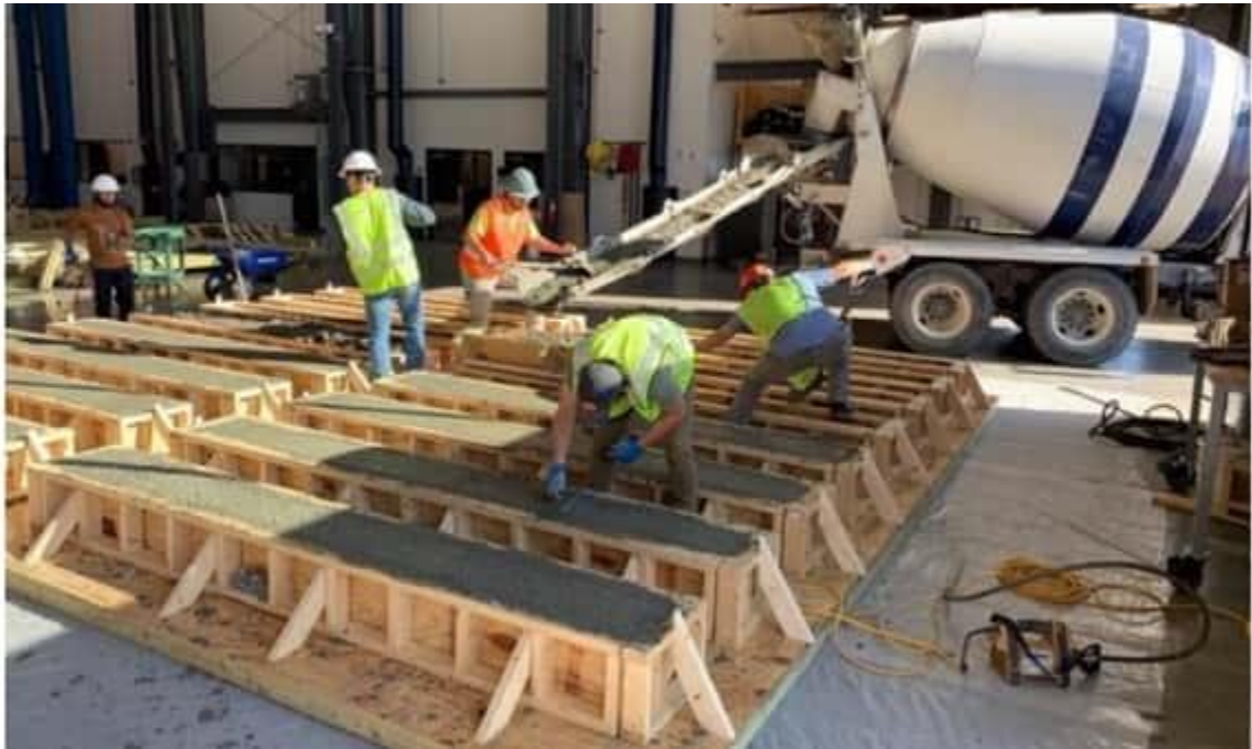
Figure 4-6 Concrete casting, vibrating and finishing
