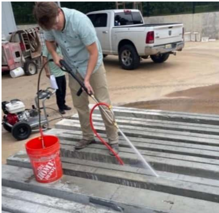
Figure 4-18 Low-pressure water blasting with abrasives
