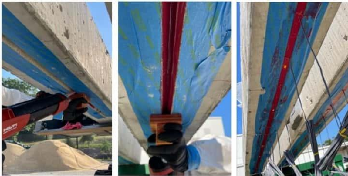
Figure 4-19 First lift of epoxy application (left and middle), and Installed TiAB after final epoxy lift (right)
