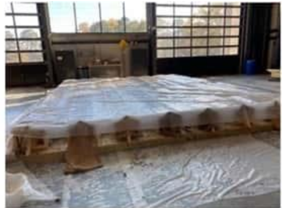
Figure 4-8 Beam after placement (Left) and moist curing (Right)
