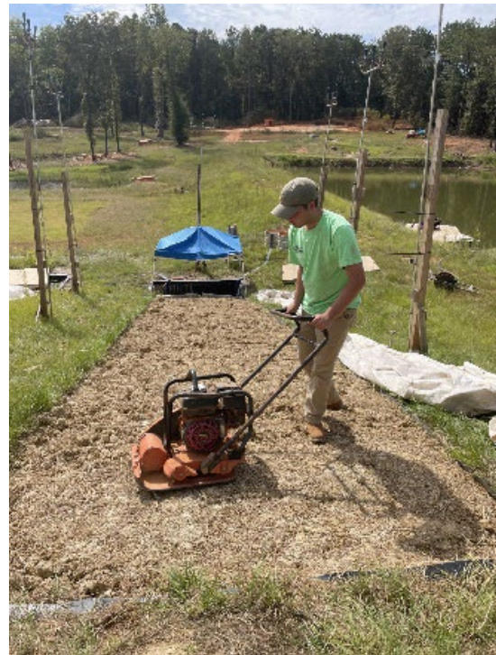
(b) Plot Compaction
