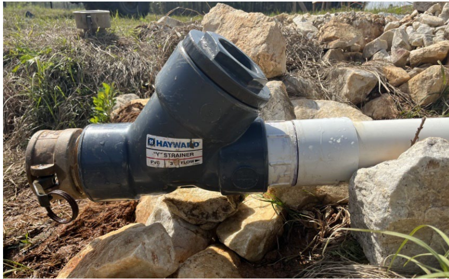
Figure 3-18: Supply Pipe Intake Debris Filter
