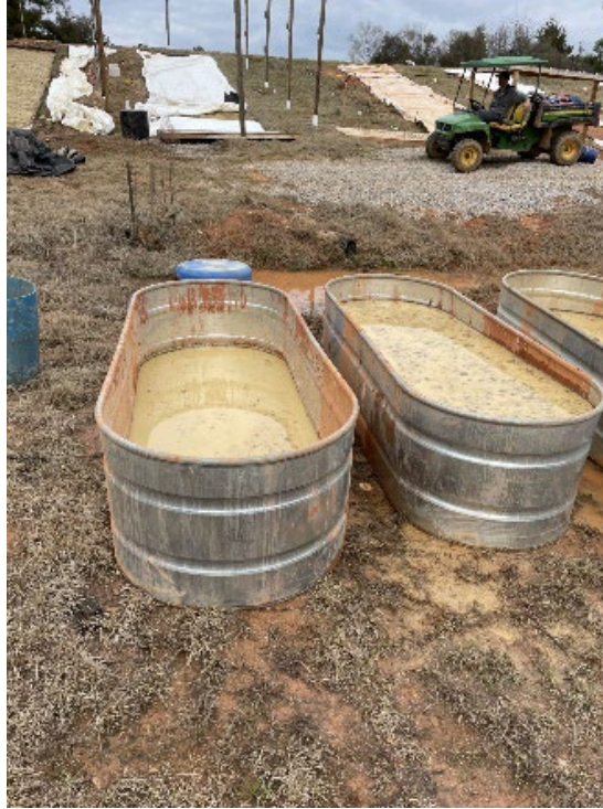
Figure 3-40: Sediment Collection Troughs
