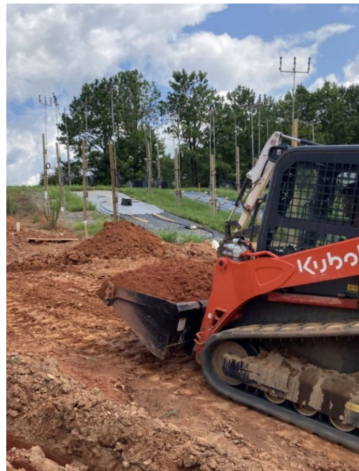
(b) adding soil to plot with skidsteer
