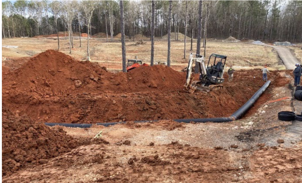
Figure 3-13: Drainage Pipe Installation
