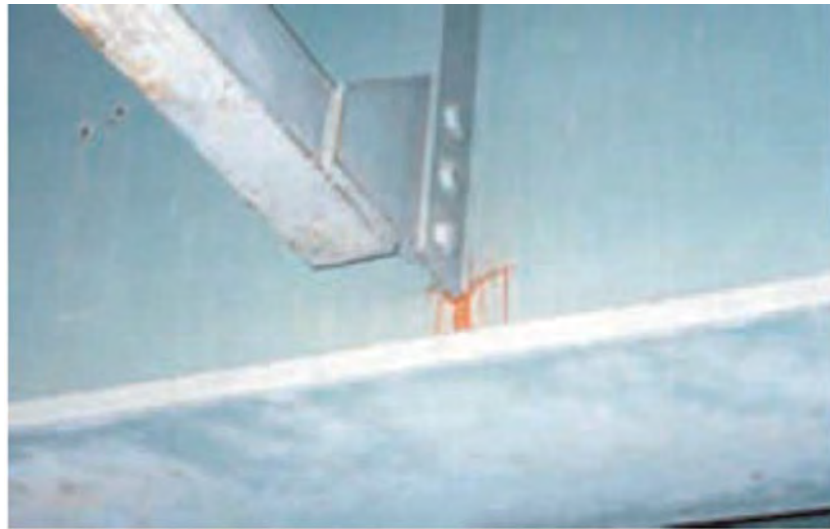
Figure 2.15: Fatigue cracks at the lower end of the vertical connection plate (Bowman et al. 2012)
