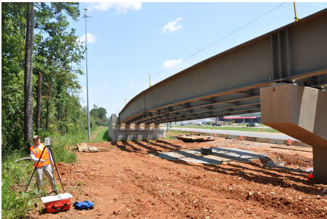
Figure 4.27: Scanner setup for Girder No. 1, erection condition
