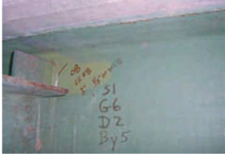
Figure 2.16: Fatigue cracks at the upper end of the connection plate (Bowman et al. 2012)
